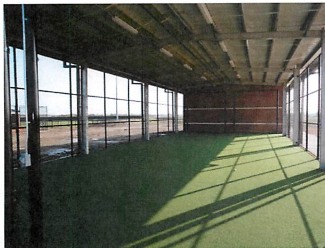
5. Turf installation at batting cage
