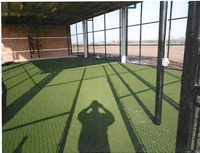
3. Turf installation at batting cage
