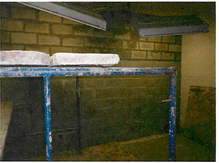
6. CMU partition at Men's restroom
