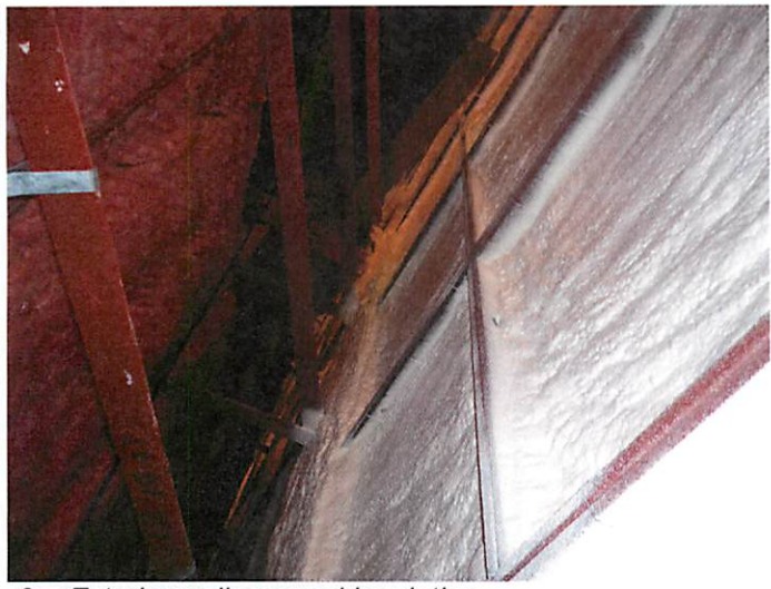
3. Exterior wall sprayed insulation
