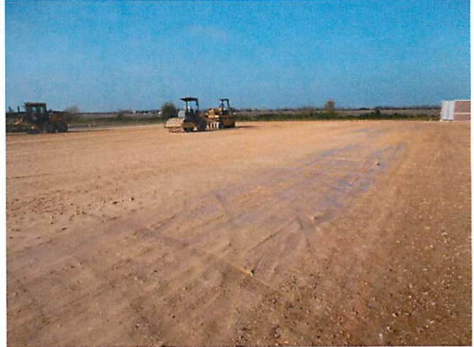
2. Limestone installation at parking area
