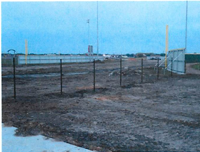
9. Post installation at security fencing
