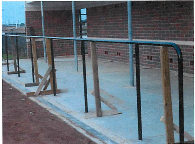
8. Protective pipe rail at dugouts
