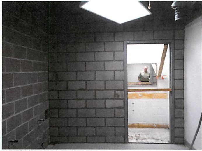
5. CMU and door frame at storage
