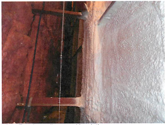
2. Exterior wall sprayed insulation
