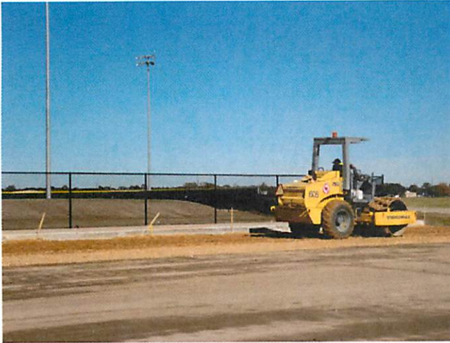
1. Limestone installation at parking area
