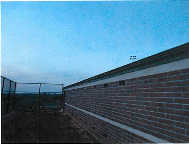
7. Gutter installation at dugouts
