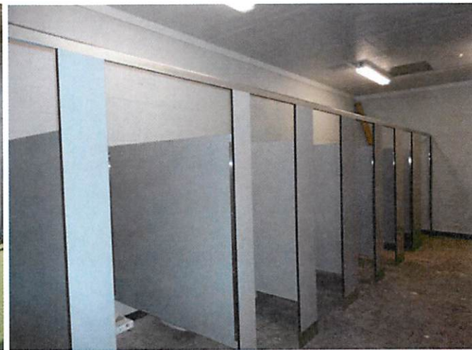
6. Toilet partitions at women's restroom
