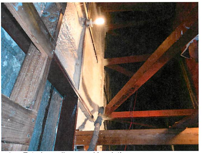
4. Exterior wall sprayed insulation
