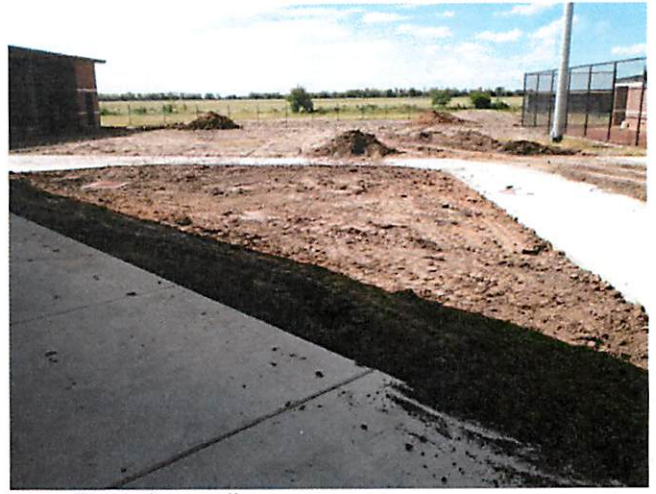
4. Final site grading
