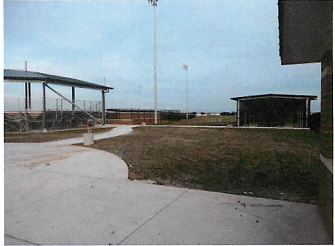
8. Final grading and irrigation system
