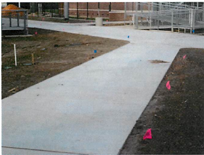
5. Irrigation system at commons
