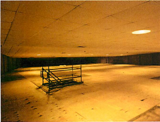
7. Upper level scaffolding
