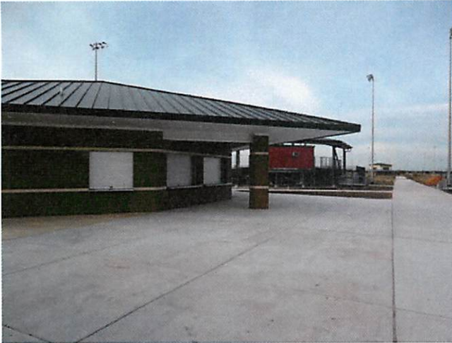
7. West elevation concession building
