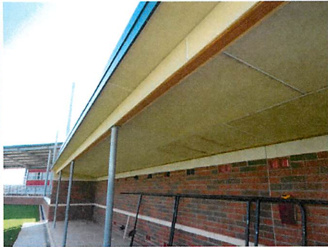
6. Hardi soffits and trim at baseball dug-outs
