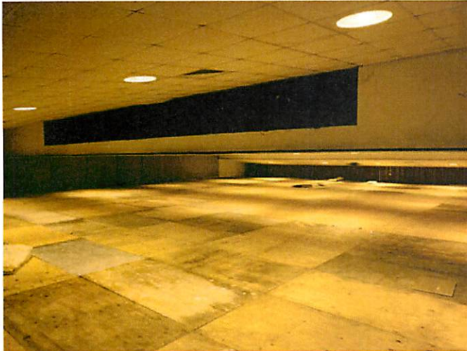
9. Upper level scaffolding at theatrical lights
