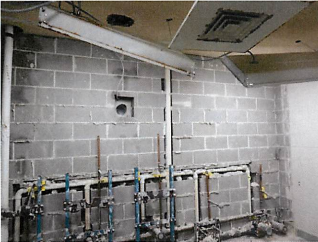
1. Demolition at men's restroom
