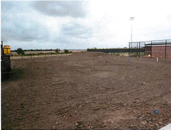
3. Final site grading at softball field
