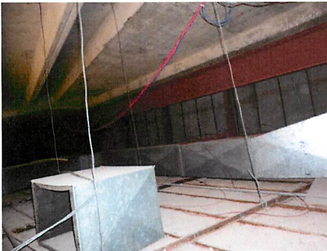
3. Attic space above entry soffit
