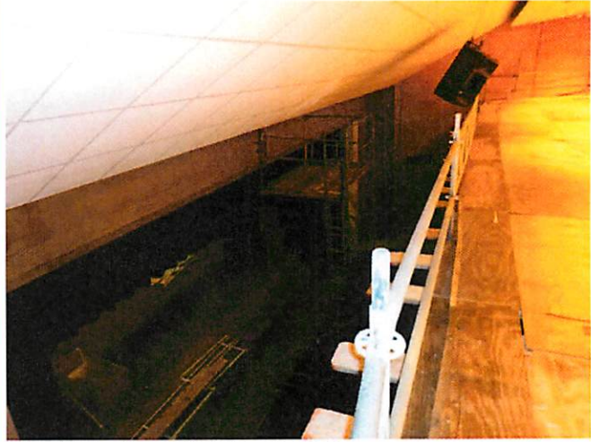
8. Portable scaffolding at stage
