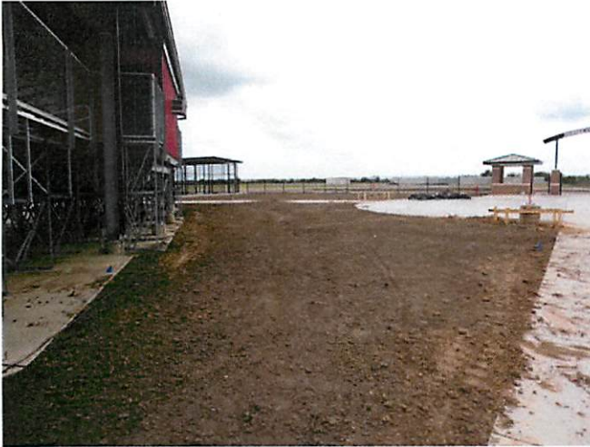
1. Final site grading at commons area
