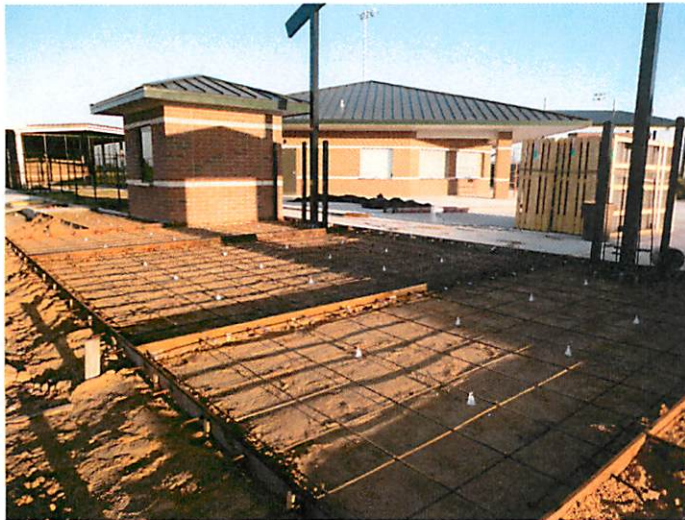
9. Concrete preparation at main entrance
