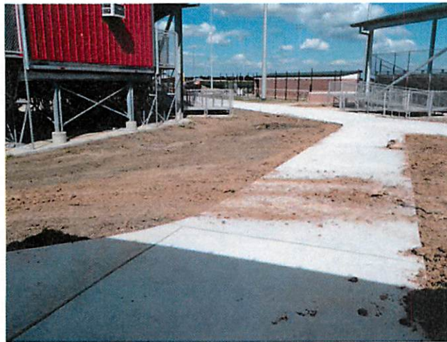
5. Final site grading
