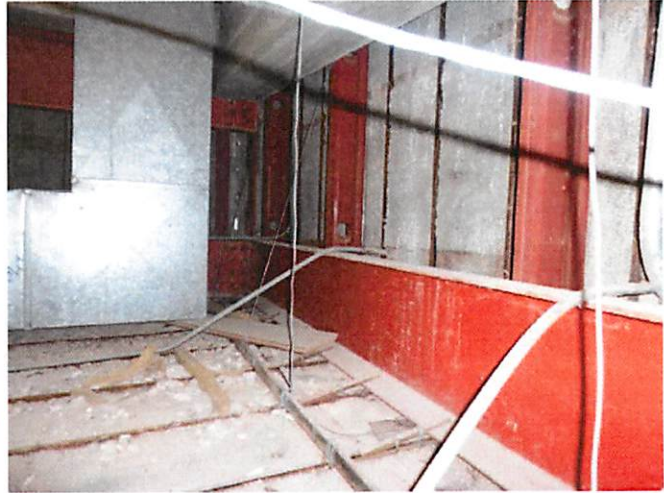
4. Attic space above entry soffit
