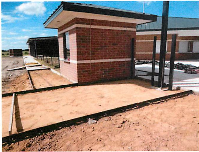
3. Concrete preparation at main entrance
