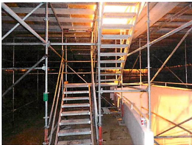
5. Stair access to upper level scaffolding
