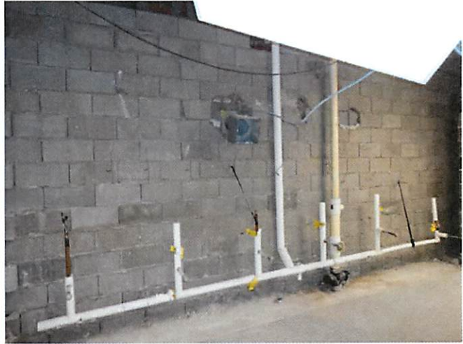
2. Plumbing chase wall at women's restroom
