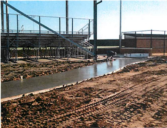
1. Concrete walks at baseball commons area
