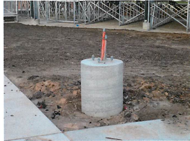
4. Site lighting concrete foundation
