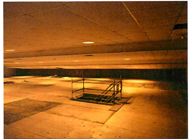
6. Upper level scaffolding
