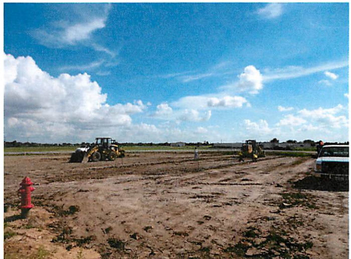
6. Subgrade prep @ parking area
