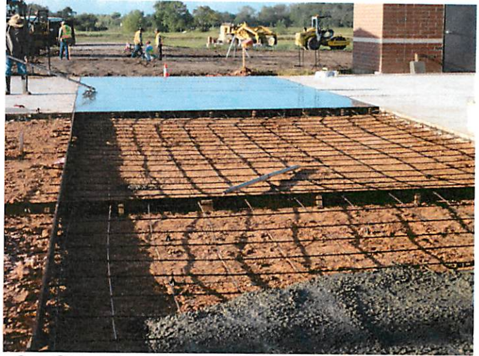
2. Concrete walk prep at Concession area
