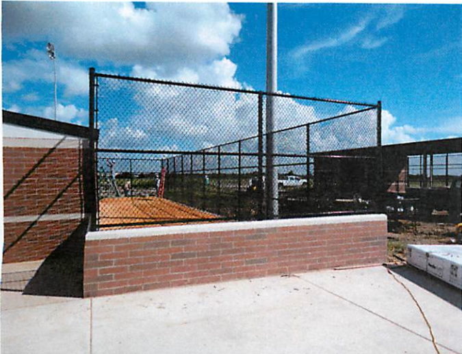
3. Fencing installed at baseball bullpen
