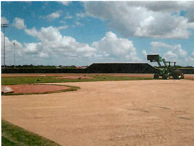
3. Turf installation at baseball field
