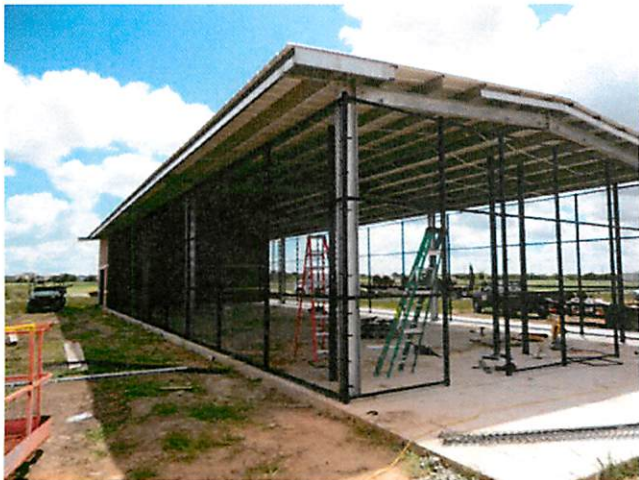
5. Fencing installation at batting cages
