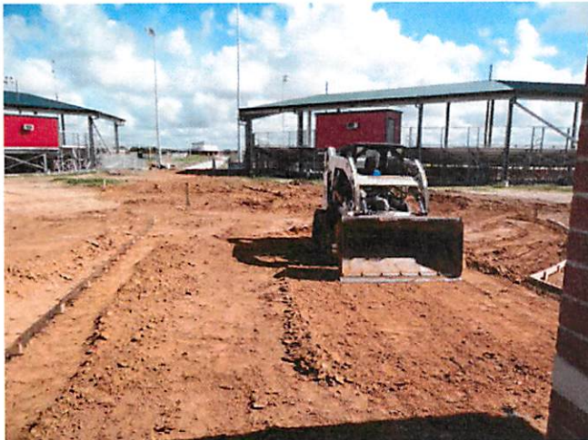
9. Concrete paving prep at commons area
