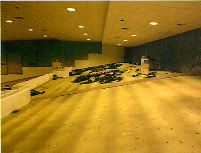
3. Auditorium seating demolition
