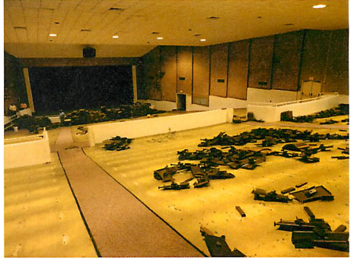
2. Auditorium seating demolition
