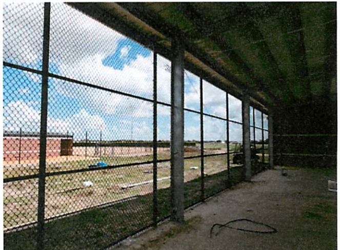
4. Fencing installation at batting cages
