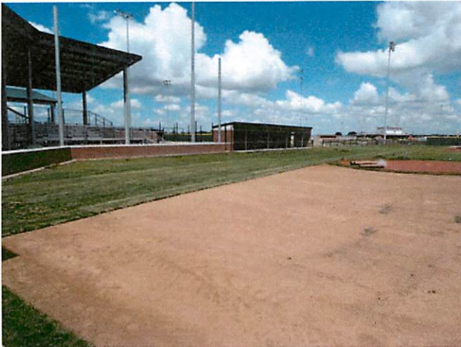
1. Turf installation at baseball field
