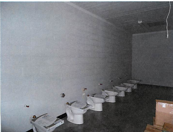
5. Plumbing fixture installation at Womens Restroom
