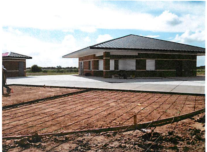
4. Concrete prep at Concession
