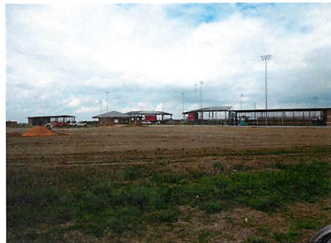
12. Rough grading at parking lot
