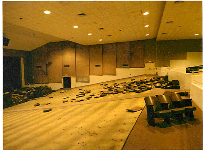
4. Auditorium seating demolition
