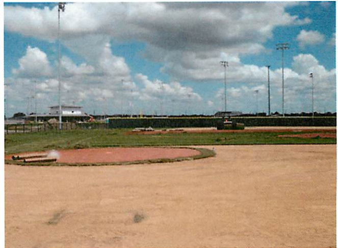
2. Turf installation at baseball field
