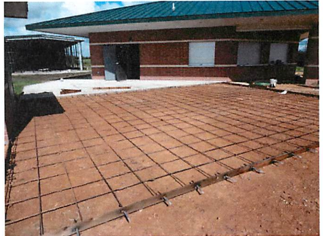
10. Concrete paving prep at commons area
