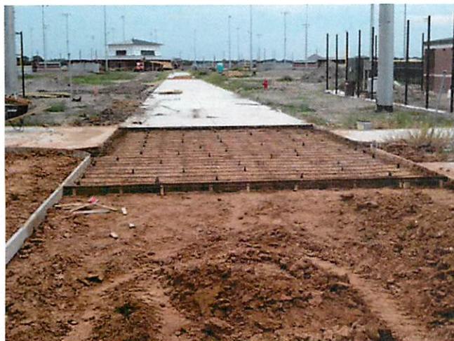
11. Concrete paving prep at main concourse
