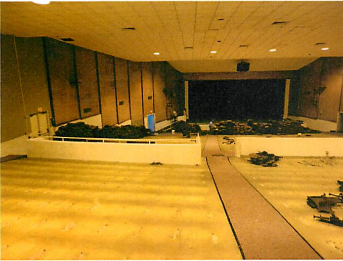
1. Auditorium seating demolition
