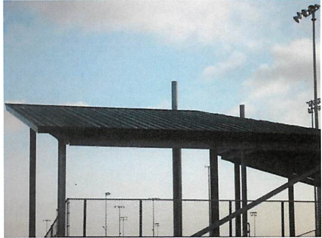
4. Bleacher cover roof system at softball field
