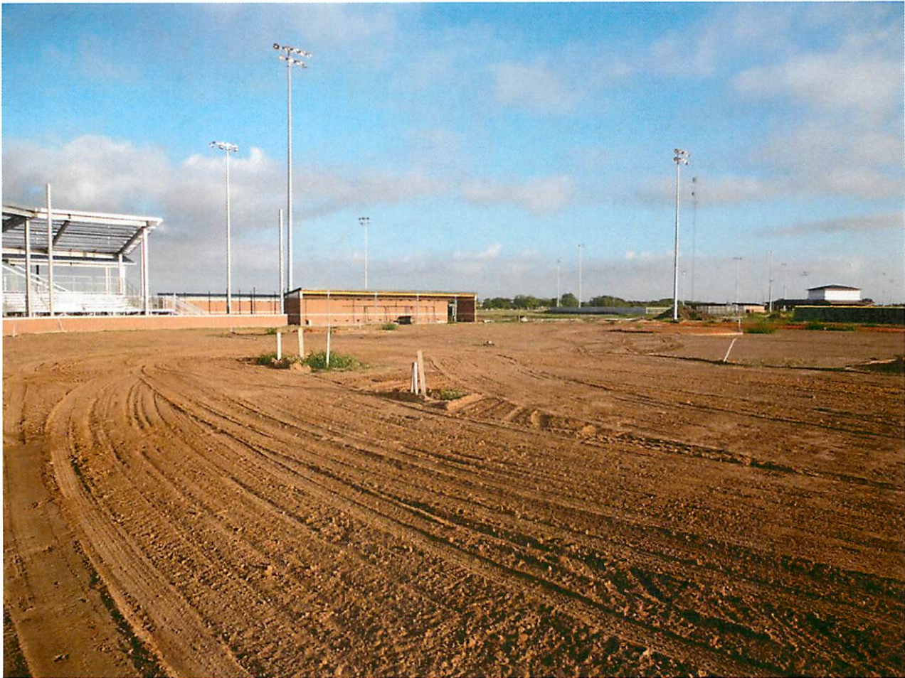
9. Top soil installation at Baseball field
