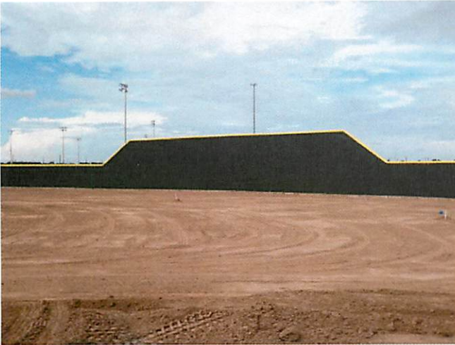
1. Metal panel outfield fence at baseball field
