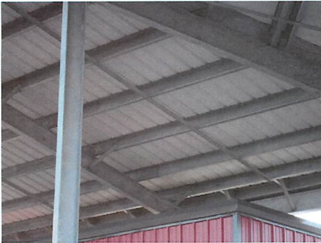
7. Bleacher cover roof system at softball field
