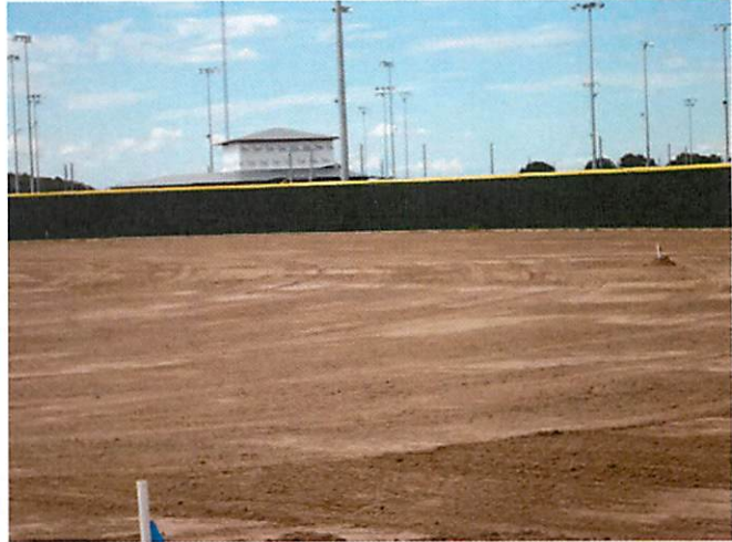
2. Metal panel outfield fence at baseball field
