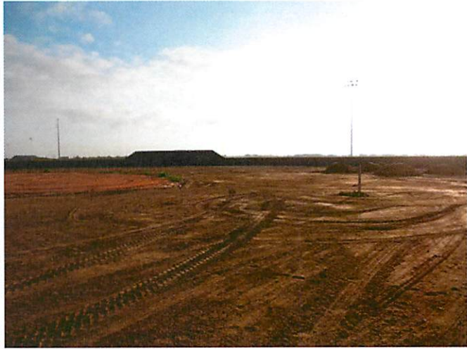
8. Top soil installation at Baseball field
