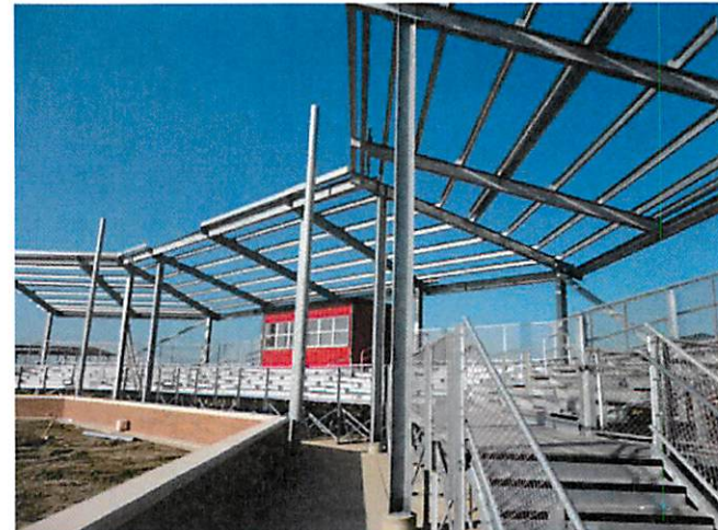
6. Bleacher cover structural framing
