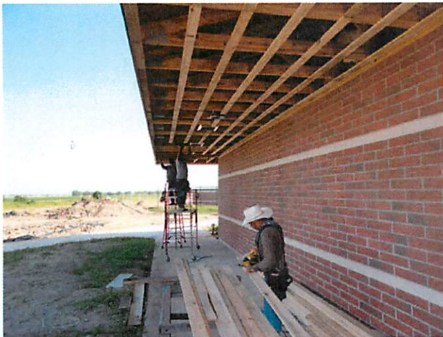
3. Concession stand soffit framing
