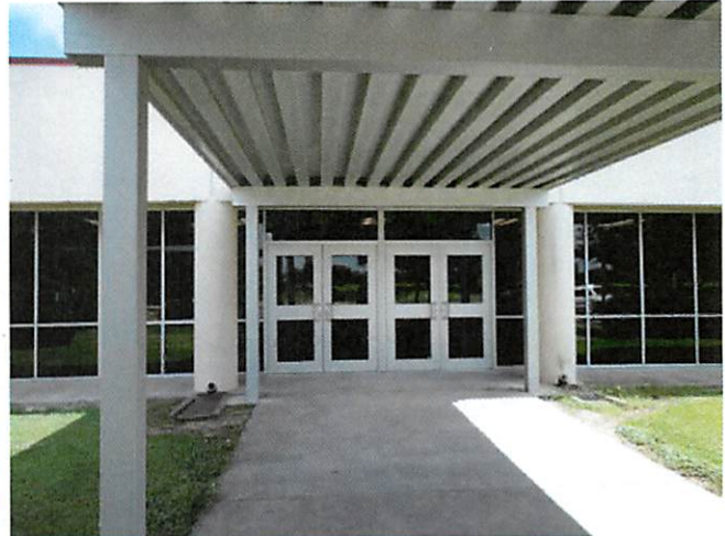
8. Myatt: Main entry storefront
