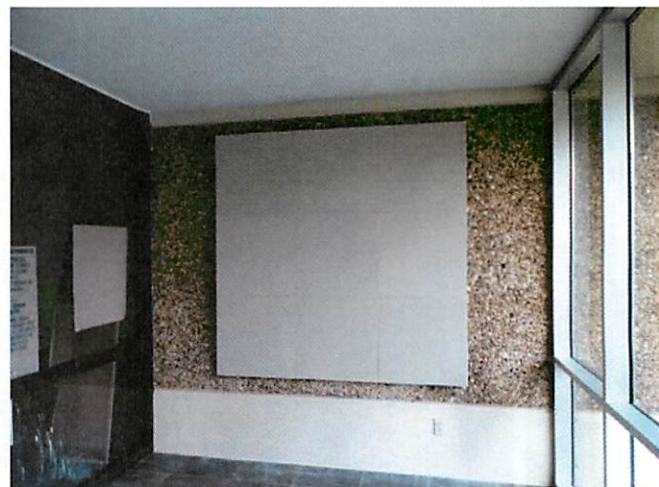
12. Myatt: Acoustical wall panel at vestibule
