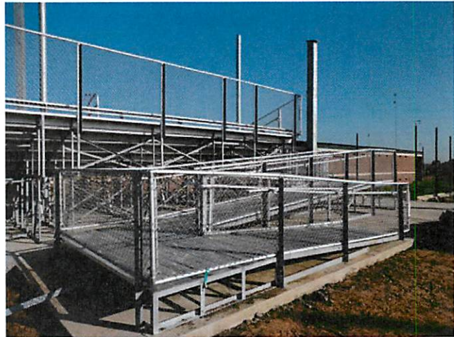
4. Entrance ramp to softball bleachers
