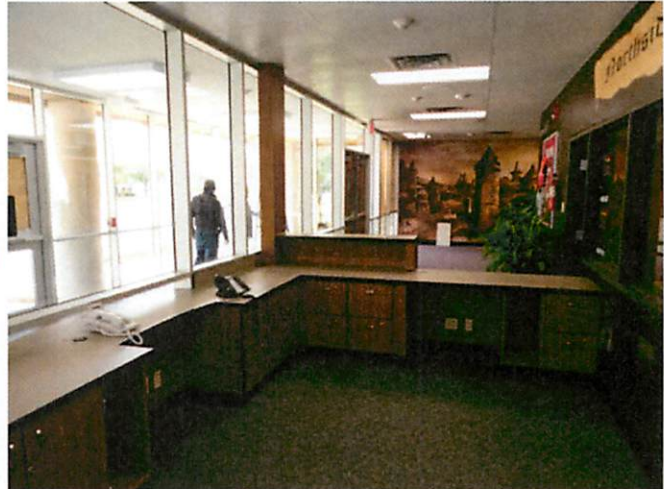
4. Northside: Reception casework at administration side
