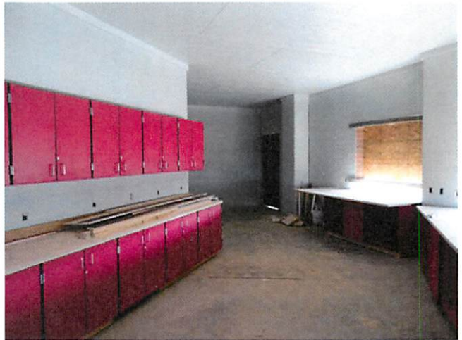
2. Concession stand casework installation
