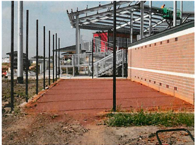
4. Installation of special soils at bullpen
