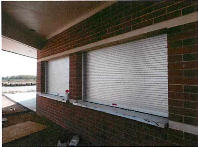
12. Rolling counter doors at Concession building
