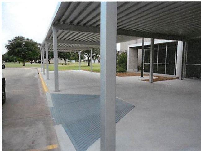
9. Northside: Concrete walks at handicap ramp
