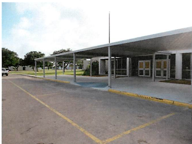
11. Northside: Aluminum canopy & concrete walks
