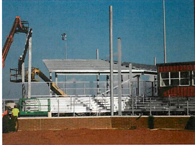
10. Bleacher cover erection at softball field
