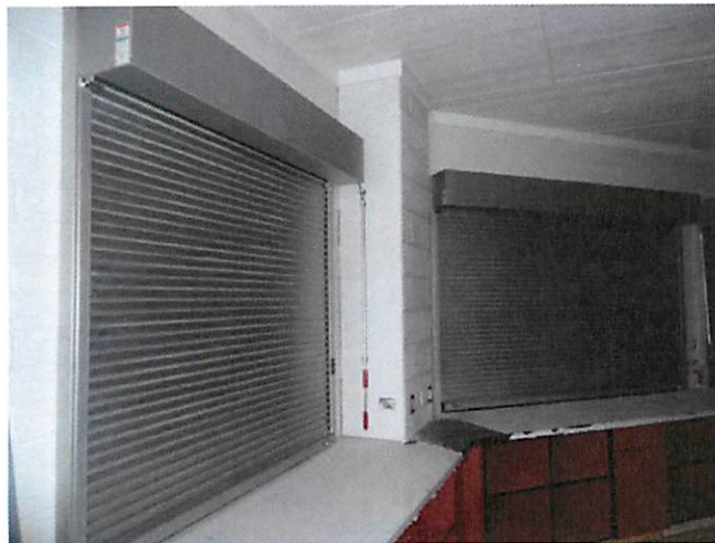
11. Rolling counter doors at Concession building
