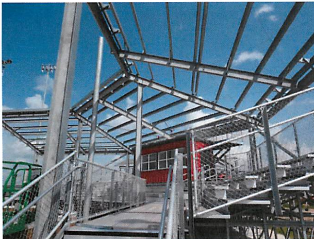
9. Covered bleacher structure at Softball field
