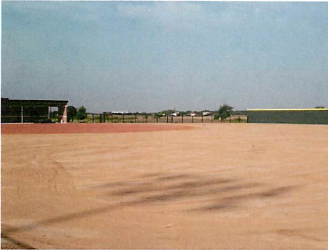
1. Softball field final grade at outfield
