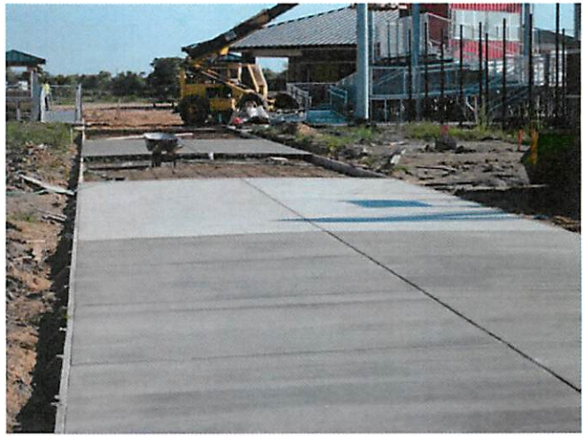
8. Concrete walks at main concourse
