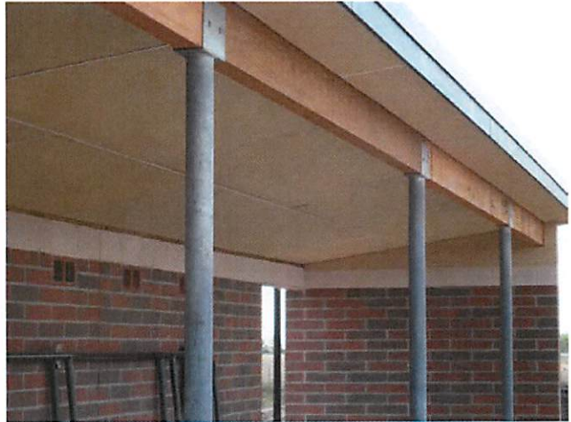
8. Hardie ceilings at dug-outs
