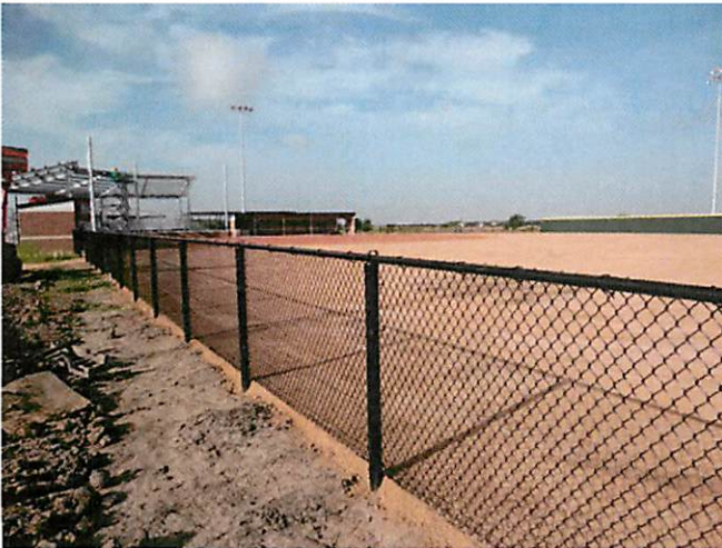
3. Vinyl coated chain link fence at Softball Field
