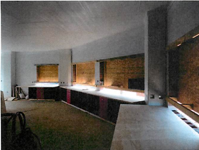
1. Concession stand casework installation
