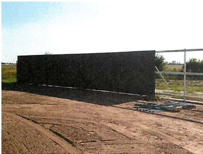
11. Outfield metal panel fence at softball field
