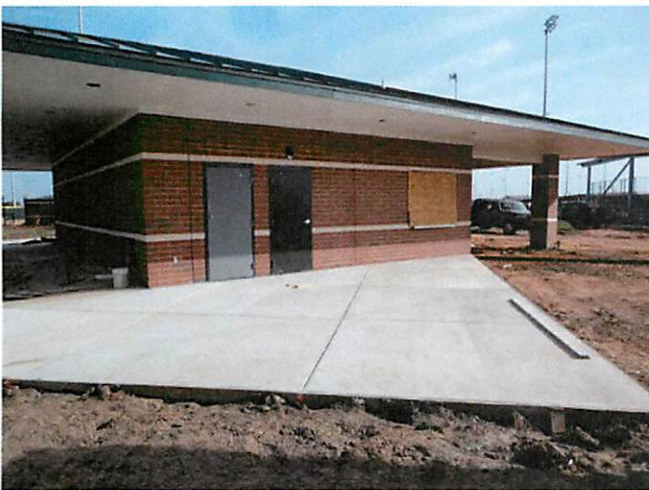
5. Concrete paving at concession area
