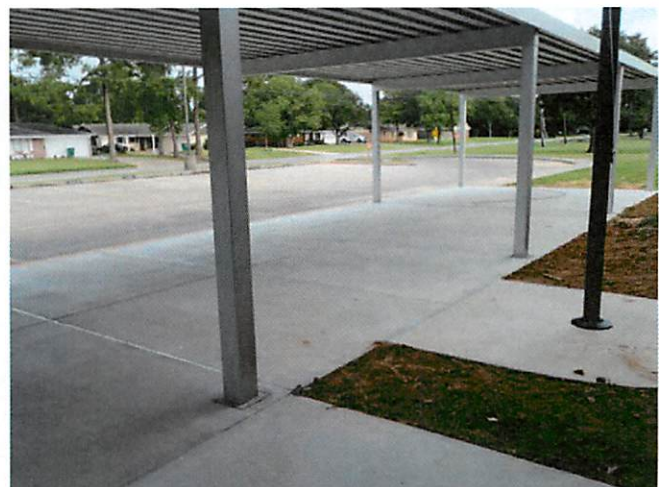
10. Northside: Concrete walks at handicap ramp
