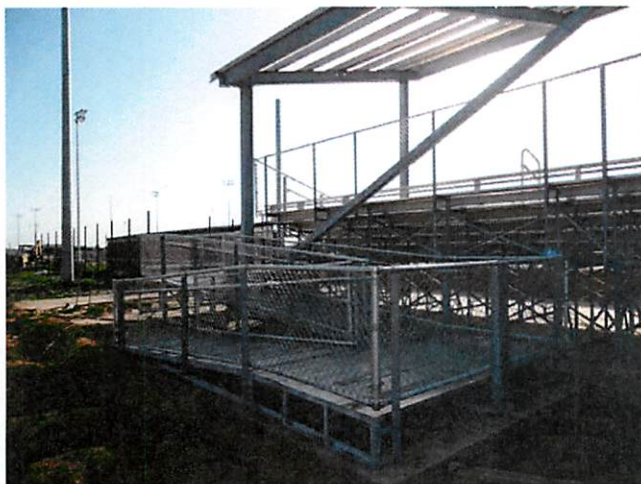
5. Entrance ramp to baseball bleachers
