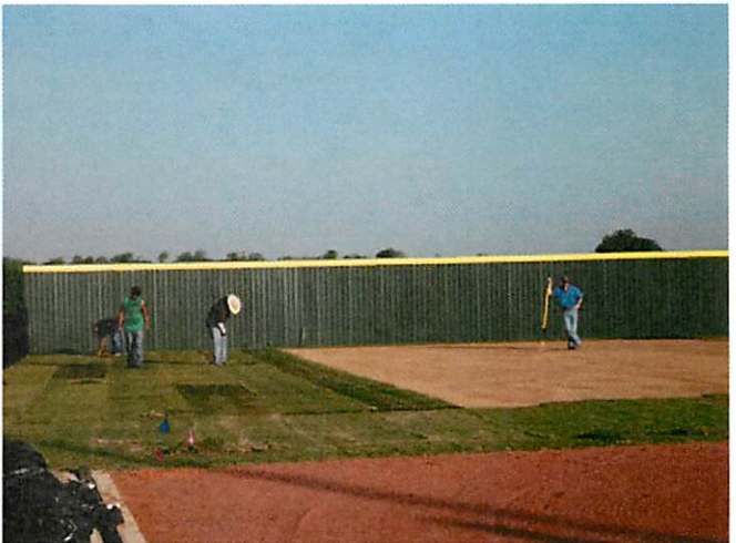
6. Turf installation at softball outfield
