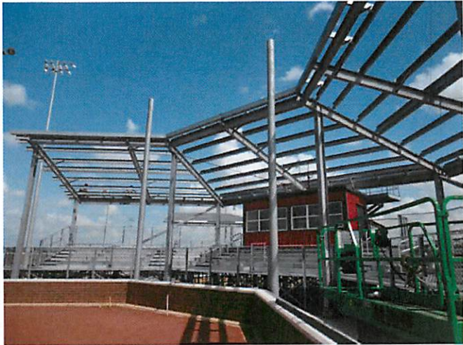
10. Covered bleacher structure at Softball field
