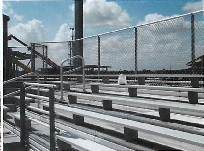
4. Softball bleacher installation
