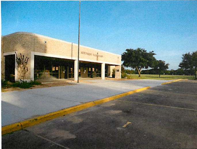
3. Concrete walks at front entry
