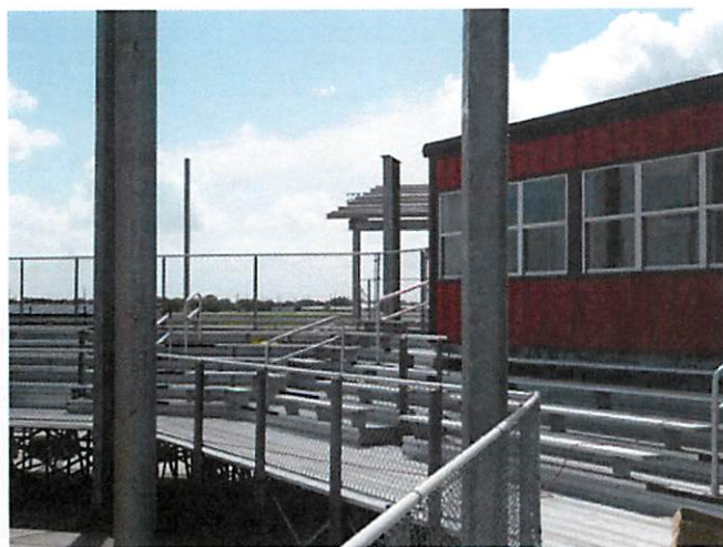
5. Softball bleacher installation
