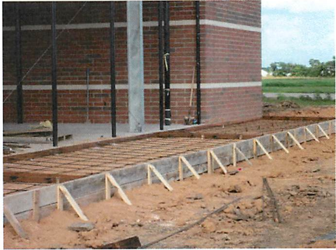
2. Concrete sidewalk at baseball batting cage
