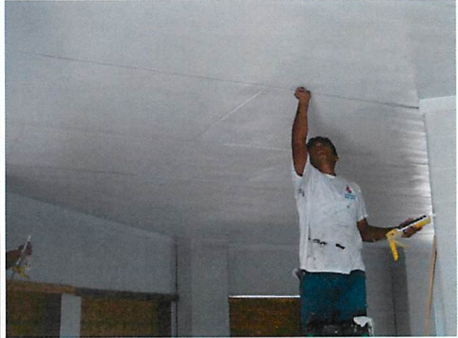
2. Interior painting at concession building
