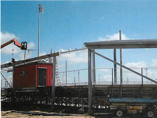
1. Baseball bleacher cover erection
