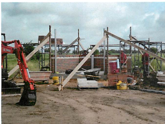
11. Masonry partitions at dumpster enclosure
