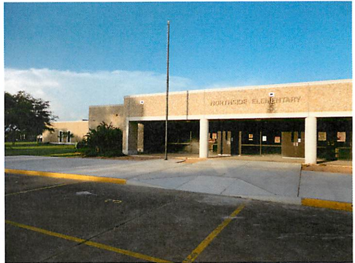
4. Flagpole reinstallation complete
