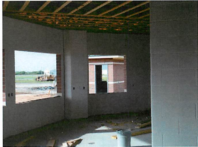
10. Block fill interior partition at concession building
