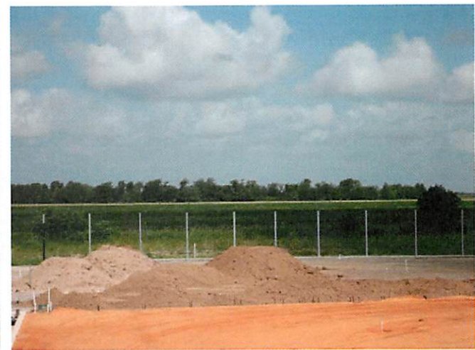
6. Topsoil installation at softball field
