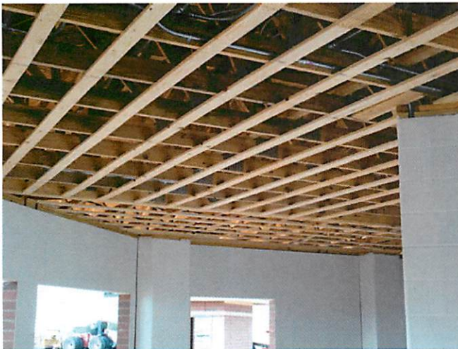
9. Ceiling framing at concession building
