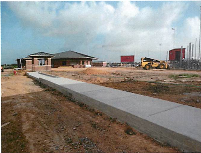
3. Concrete walks adjacent to parking area
