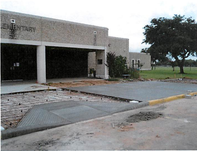
1. Concrete paving at front entry
