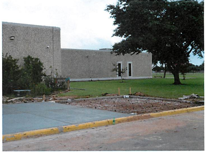
2. Concrete paving at front entry sidewalks
