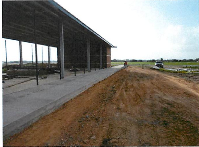
4. Concrete walks at baseball batting cage
