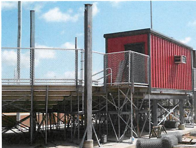
3. Softball bleacher installation
