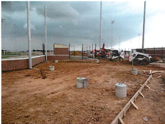
3. Concrete formwork at softball bleacher area
