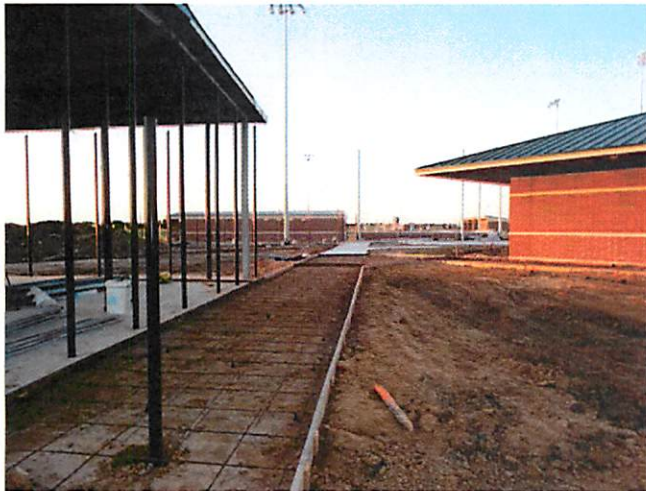
15. Concrete prep at walks, softball batting cage
