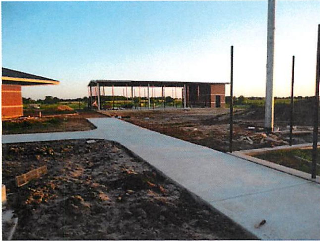
13. Concrete walks at softball area
