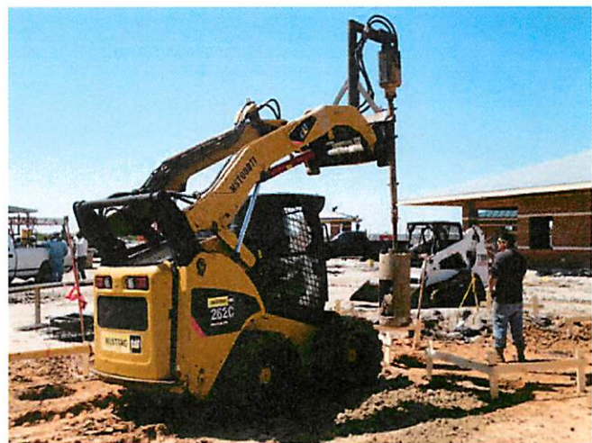
4. Drilled footing installation at baseball bleacher cover
