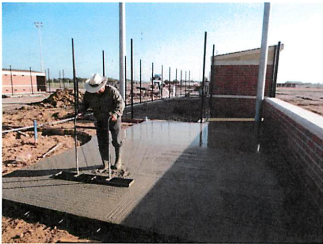
11. Concrete walks / paving at baseball bleacher area
