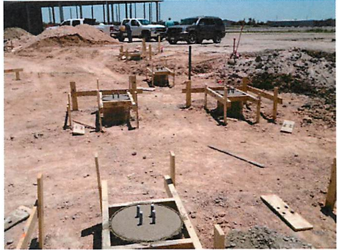
8. Elevated concrete piers at pressbox
