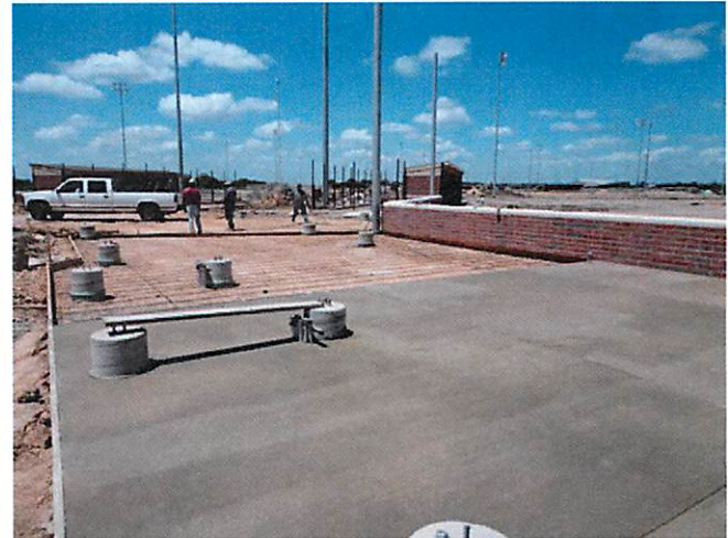
16. Concrete paving at bleacher area baseball field
