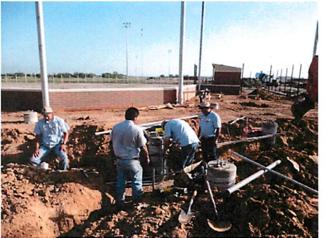
12. Underground electrical / sound to pressbox
