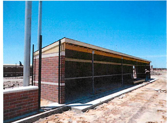
10. Roof structure and desk at dugout
