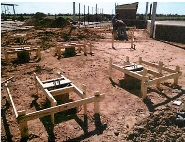
5. Concrete form work / anchor bolts at softball bleacher
