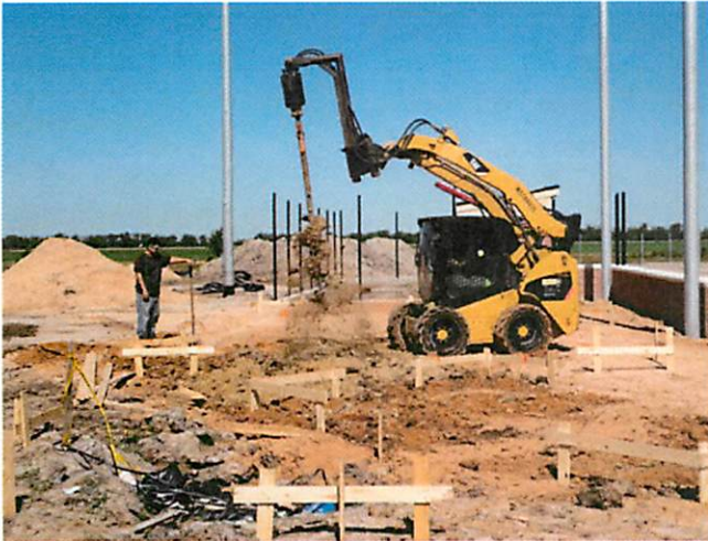
1. Drilled footing installation at softball bleacher cover
