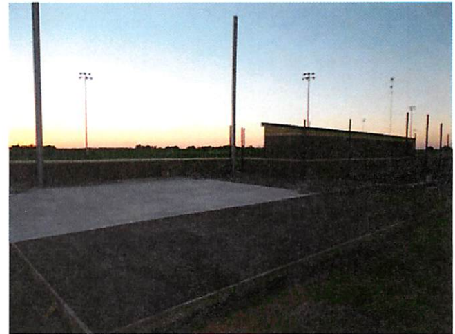
4. Concrete paving at softball bleacher area
