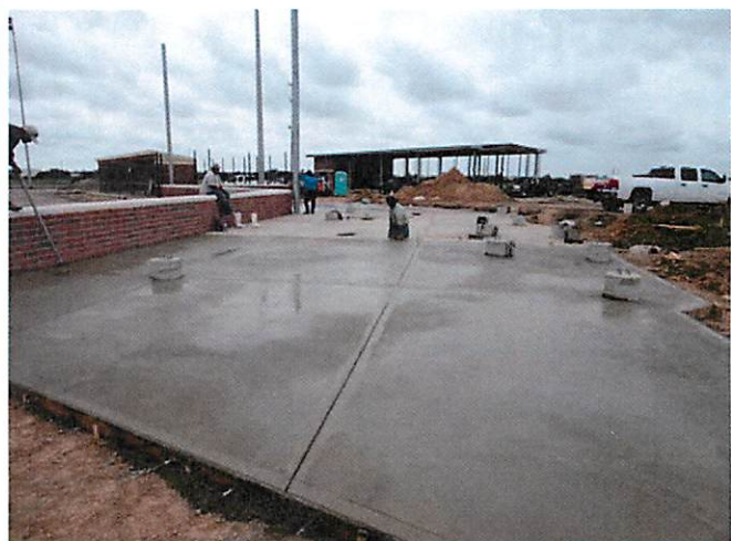
18. Concrete paving at bleacher area baseball field
