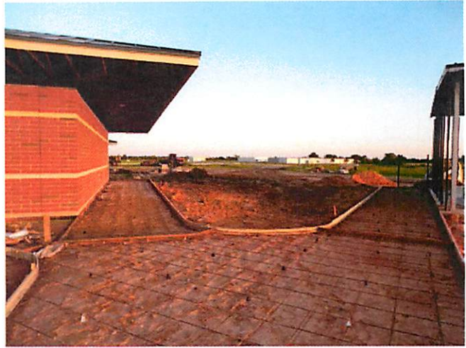
14. Concrete prep at walks, softball batting cage
