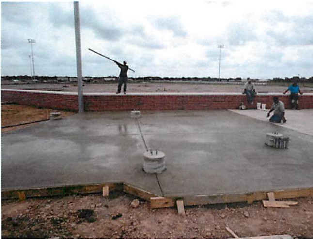
19. Concrete paving at bleacher area baseball field
