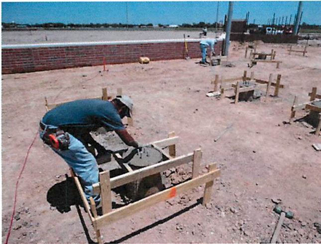
7. Concrete piers at baseball bleachers
