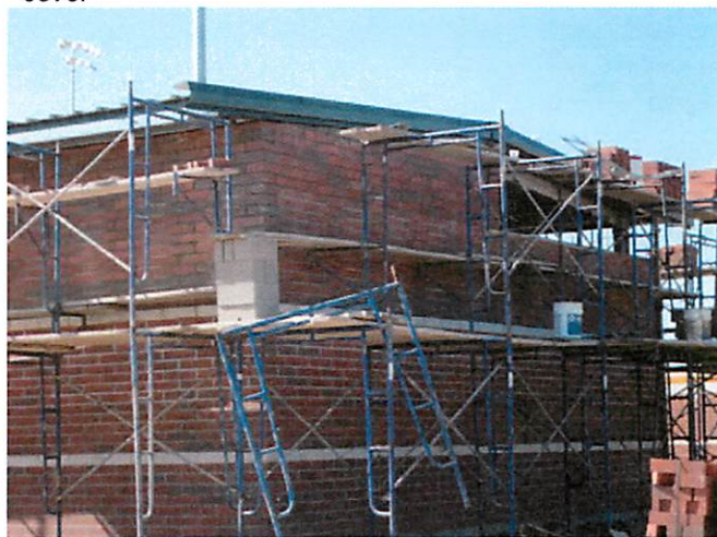
6. Masonry at softball storage building
