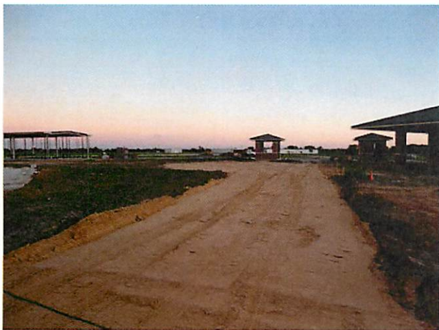
5. Select fill at main concourse
