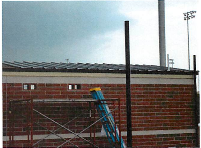
2. Dug-out roofing at softball field
