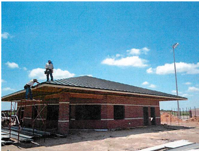
17. Metal roofing at concession building
