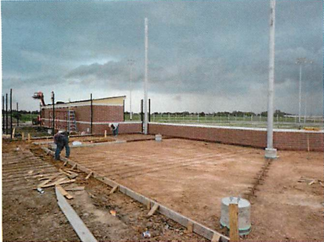
1. Concrete prep at softball bleacher area
