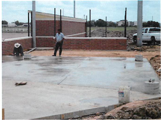
20. Concrete paving at bleacher area baseball field
