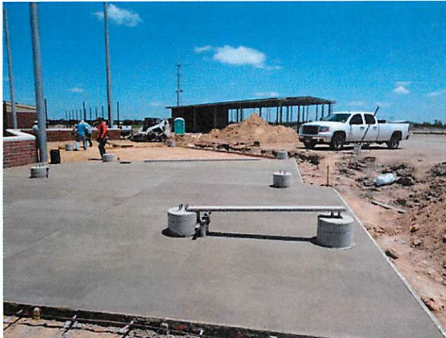
15. Concrete paving at bleacher area baseball field
