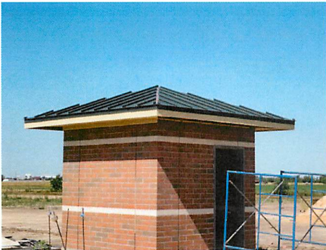
3. Metal roof at Ticket Booth
