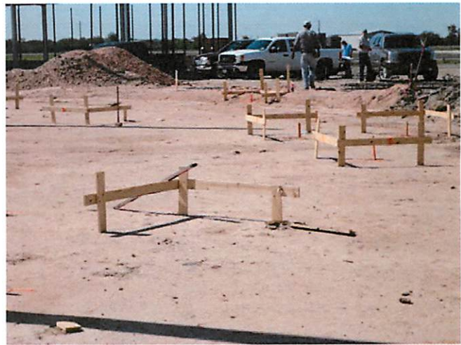
2. Drilled footing layout at baseball cover
