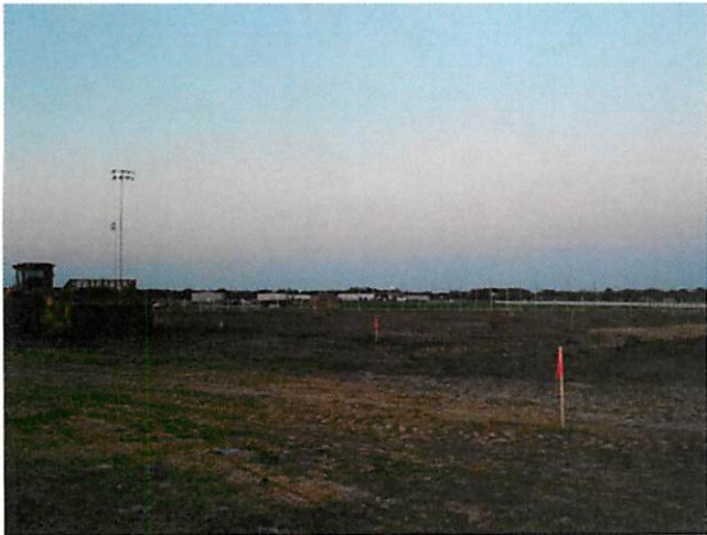
1. Final subgrade prep at baseball field
