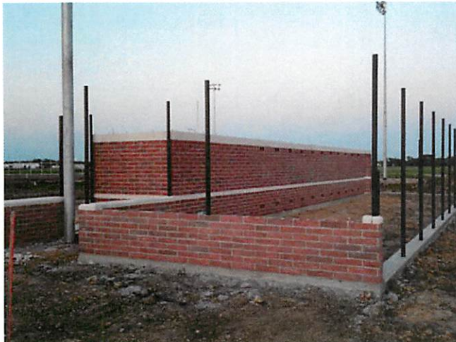
3. Masonry partition at bullpen / dugout
