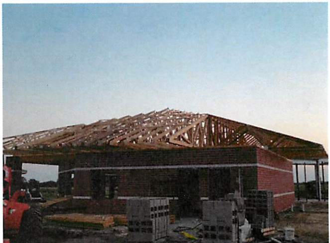
6. Wood trusses at Concession Building
