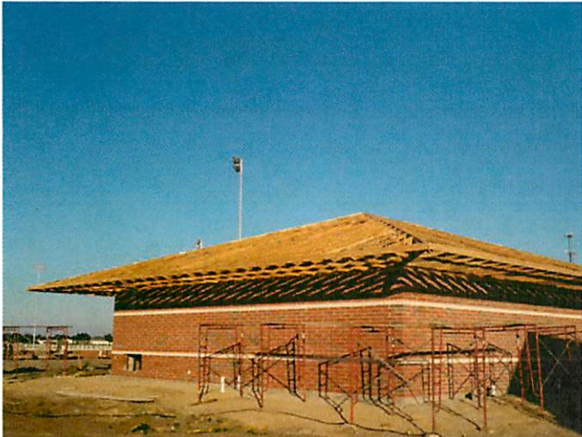
9. Wood truss installation at Concession Building
