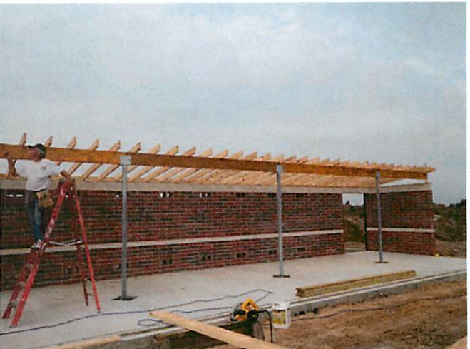
6. Roof framing at softball dugout
