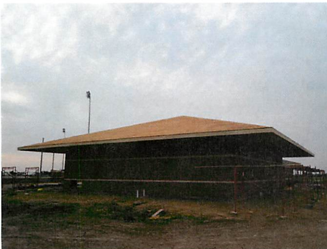
5. Roof Deck at Concession building
