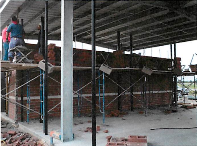
4. Masonry storage building at baseball batting cage
