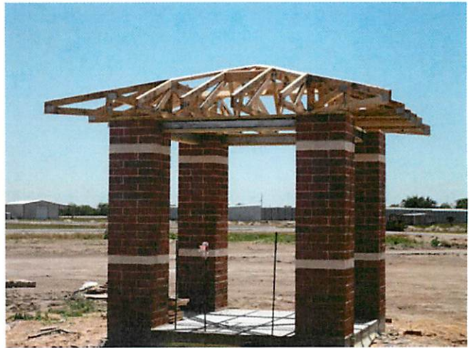
2. Wood trusses at entry pavilion
