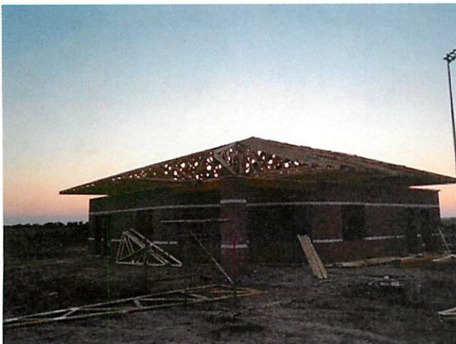
5. Wood trusses at Concession Building
