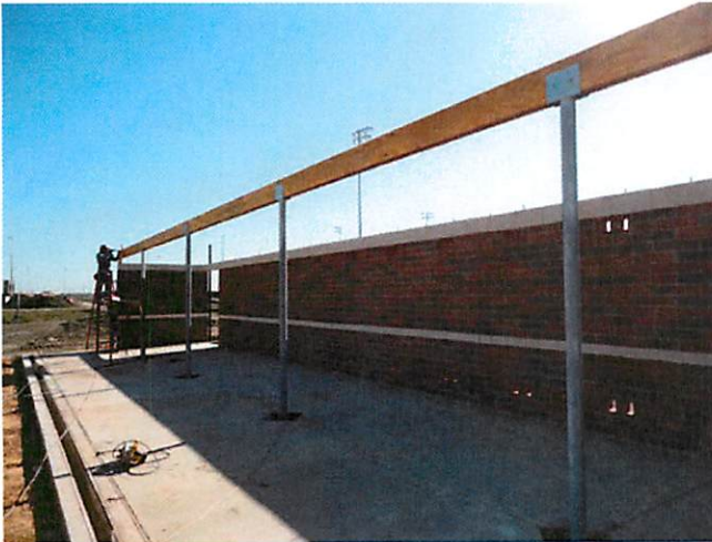
1. Dugout columns and support beam at softball field
