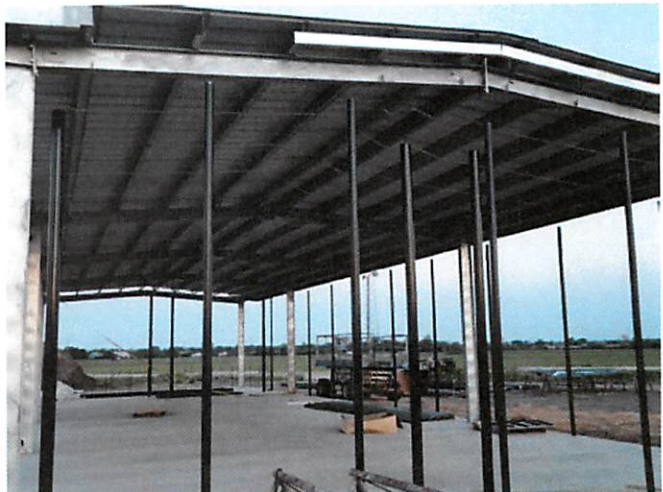
4. Metal roofing at baseball Batting Cage
