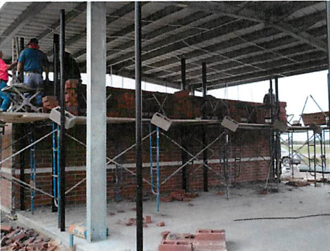
3. Masonry storage building at baseball batting cage
