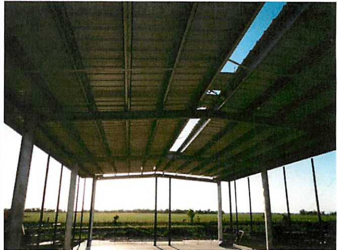
8. Metal roofing at Batting Cage
