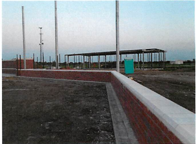
2. Masonry backstop at baseball field
