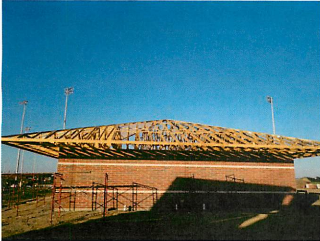
7. Wood truss installation at Concession Building
