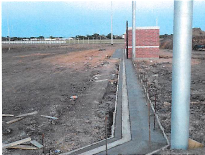
3. Concrete / Trench drain foundation at baseball field
