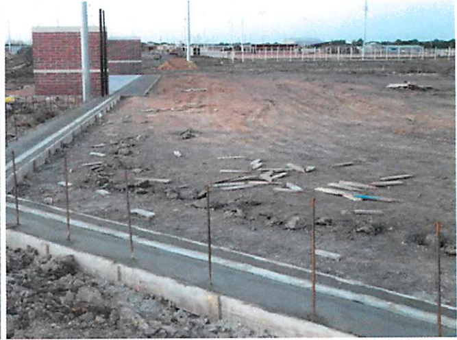
4. Concrete / Trench drain foundation at baseball field
