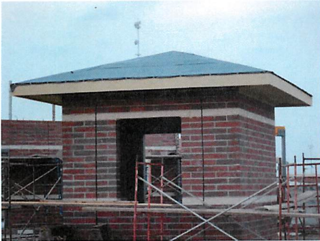
7. Roof underlayment and cornice
