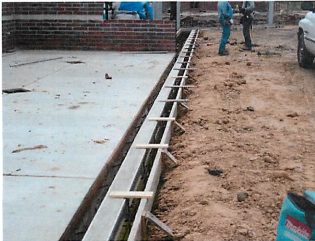
9. Trench drain installation at softball field
