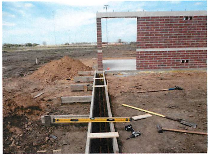
6. Concrete prep at softball field bull pen perimeter
