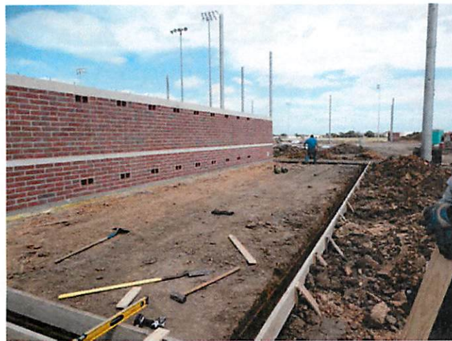
5. Concrete prep at softball field bull pen perimeter
