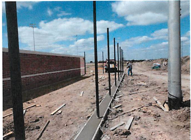
10. Concrete beams / fencepost installation at softball field bullpens.
