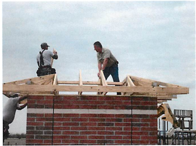
2. Ticket Booth roof framing
