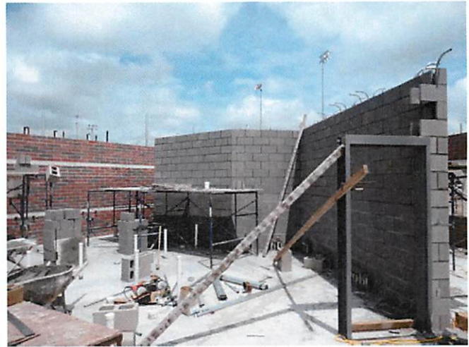
10. Interior CMU partitions at Concessions Building
