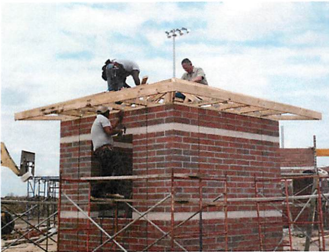
1. Ticket Booth roof framing
