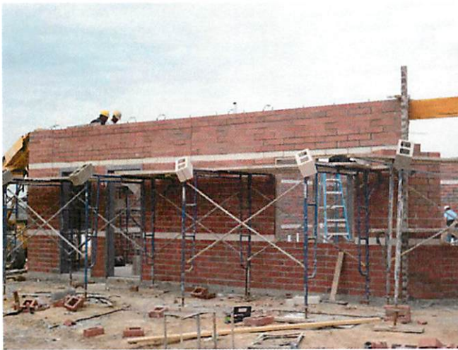
3. Masonry partitions at Concession Building
