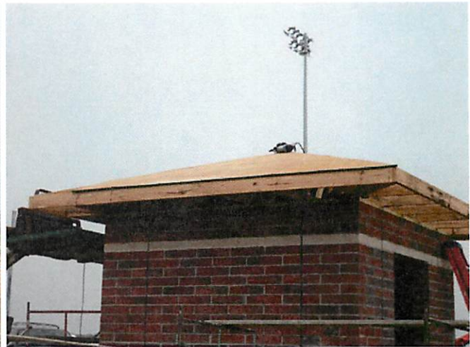
6. Roof deck at Ticket Booth
