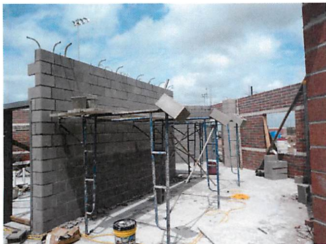
11. Interior CMU partitions at Concessions Building
