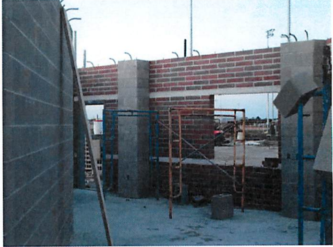
2. Interior masonry at concession building
