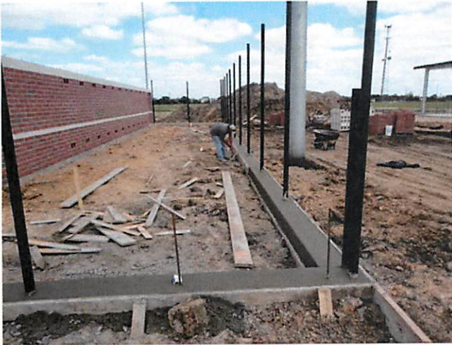
7. Concrete beams / fencepost installation at baseball field bullpens.
