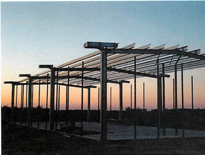
1. Softball batting cages main framing in place
