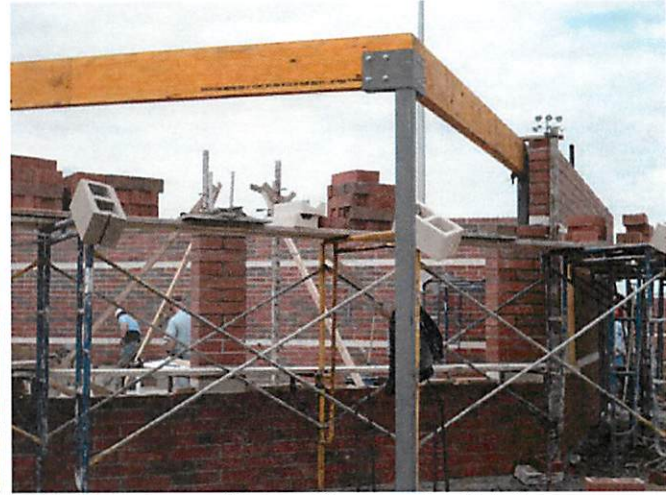
4. Masonry partitions at Concession Building
