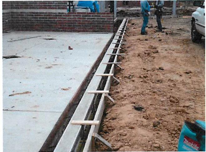
8. Trench drain installation at softball field
