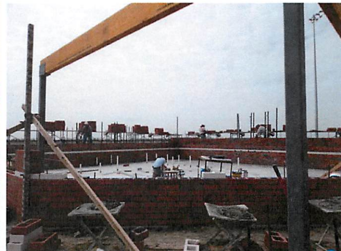
12. Masonry partitions at concession building
