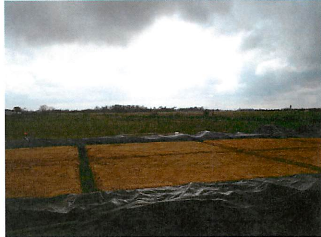
16. Softball batting cage grade beam excavation
