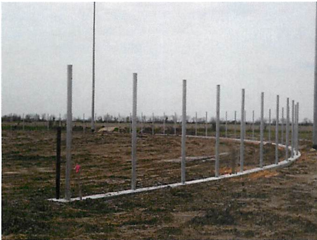
9. Concrete beam at outfield fence
