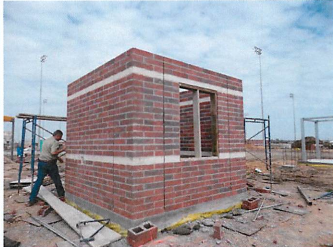
10. Masonry partitions at ticket booth
