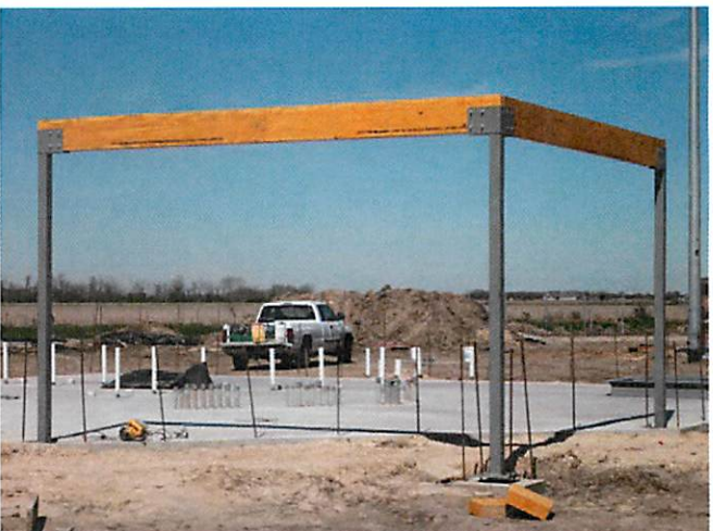
6. Structural columns & beams at concession bldg.
