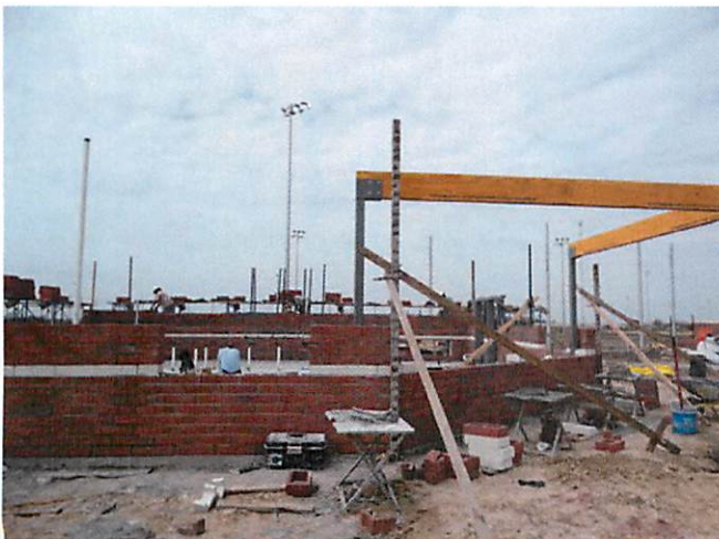
11. Masonry partitions at concession building
