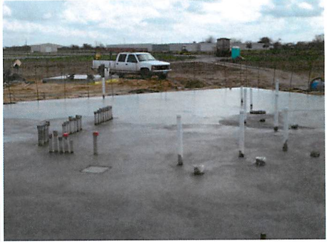
2. Concrete foundation at Concessions
