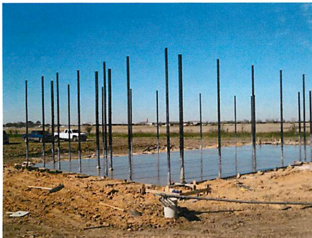
5. Softball batting cage concrete foundation
