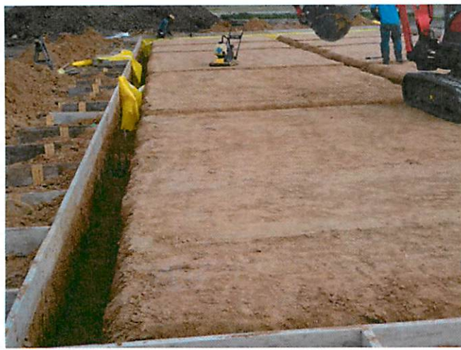
5. Grade beam excavation at baseball batting cage
