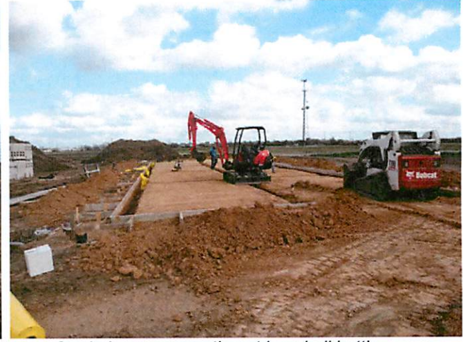
4. Grade beam excavation at baseball batting cage
