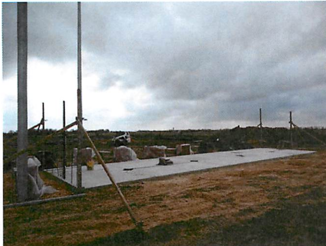
15. Masonry prep at softball dugouts
