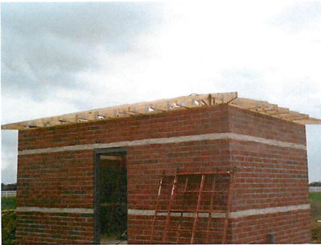
7. Irrigation building roof framing
