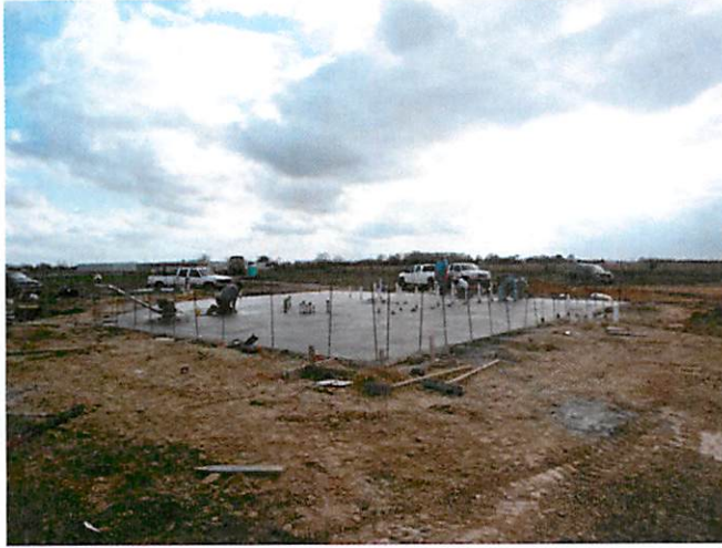
3. Concrete foundation at Concessions
