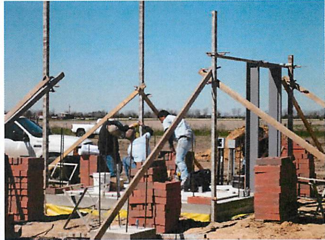
8. Ticket booth masonry prep
