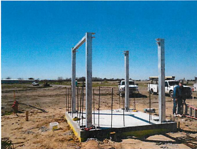
7. Structural columns at entry pavilion
