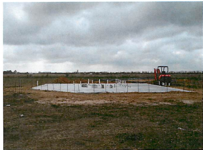
12. Concession stand concrete foundation
