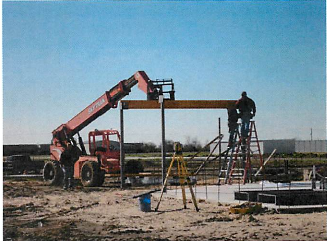
4. Structural columns & beams at concession bldg.
