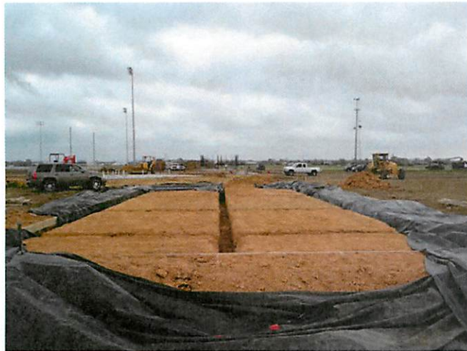
17. Softball batting cage grade beam excavation
