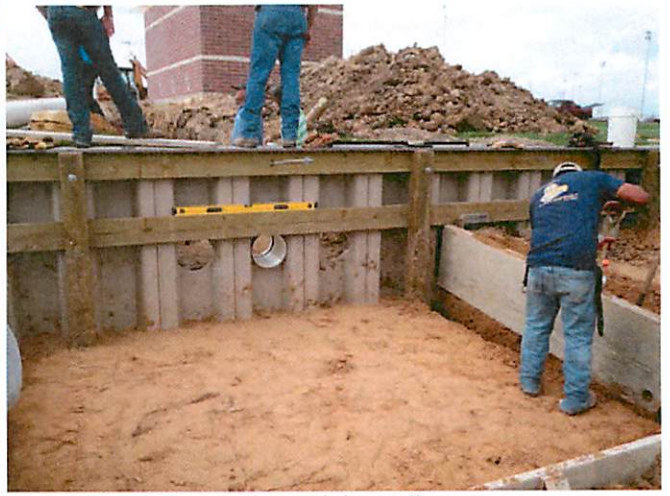
6. Wet well installation at lake wall
