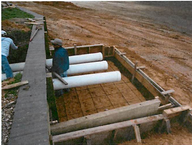
11. Concrete bulkhead at irrigation intake piping
