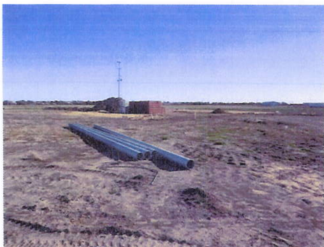
5. Backstop netting support columns
