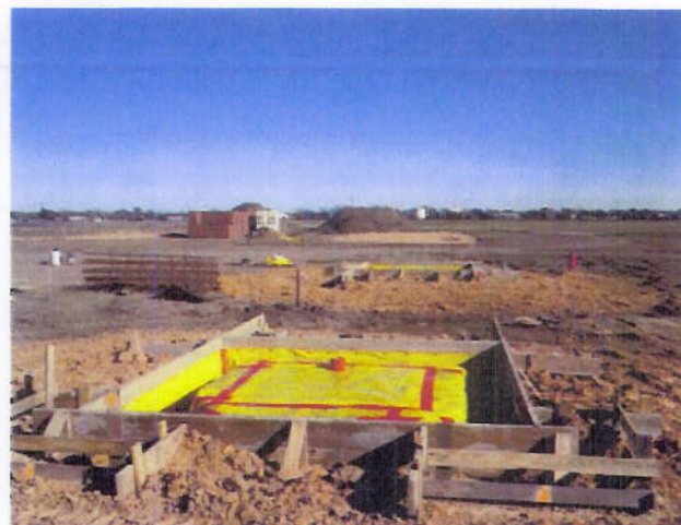
4. Front entry concrete preparation
