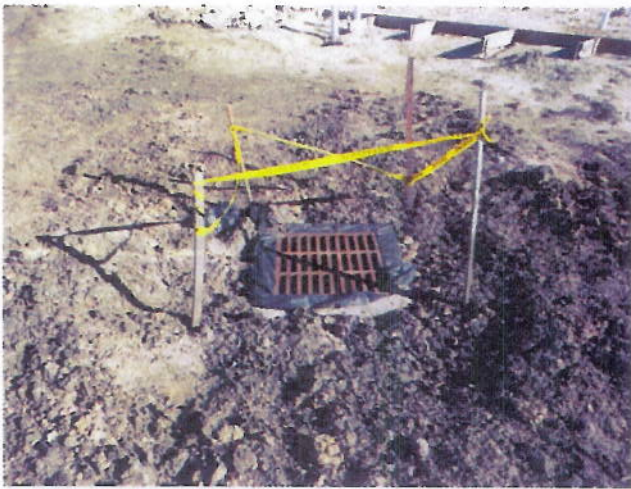
7. Site drainage catch basin
