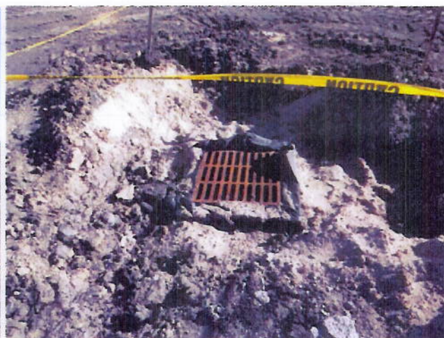
6. Site drainage catch basin
