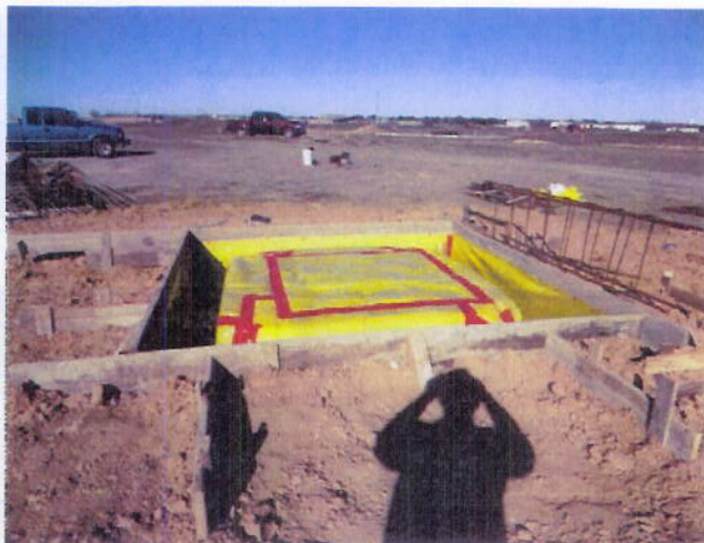
2. Pavilion foundation preparation
