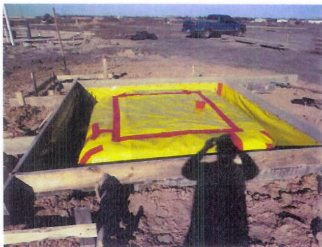
3. Ticket Booth foundation preparation
