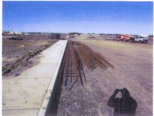
8. Foundation steel fabrication
