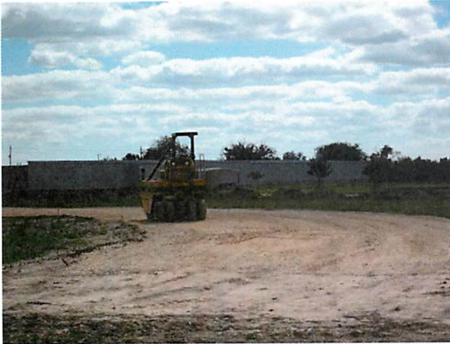
7. Limestone base material at access drives
