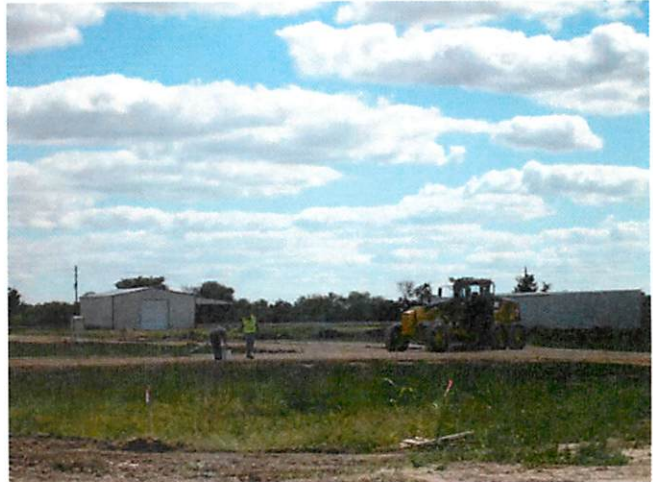
8. Limestone base material at access drives
