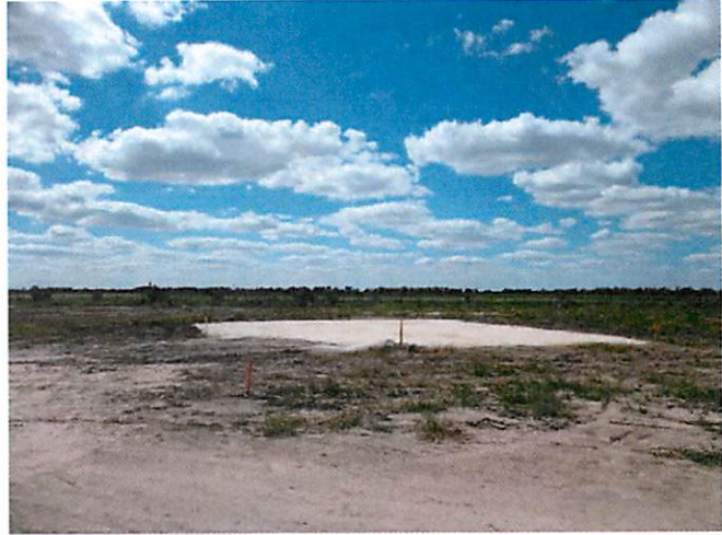
4. Select fill installation at concessions
