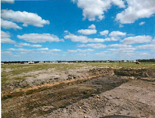
3. Excavation at baseball field dugouts
