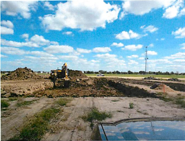
1. Excavation at baseball batting cage
