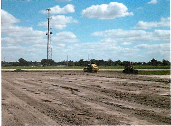
6. Preparation of subgrade at parking area
