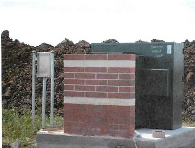
9. Masonry Mock-up
