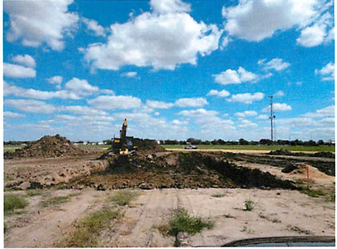
2. Excavation at baseball batting cage
