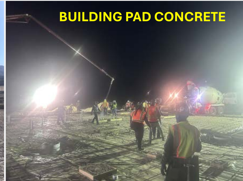
PLACING CONCTETE FOOTINGS
