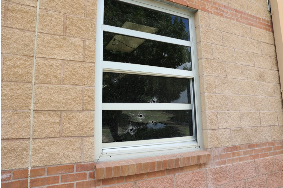
Figure 7. Exterior Classroom Window
