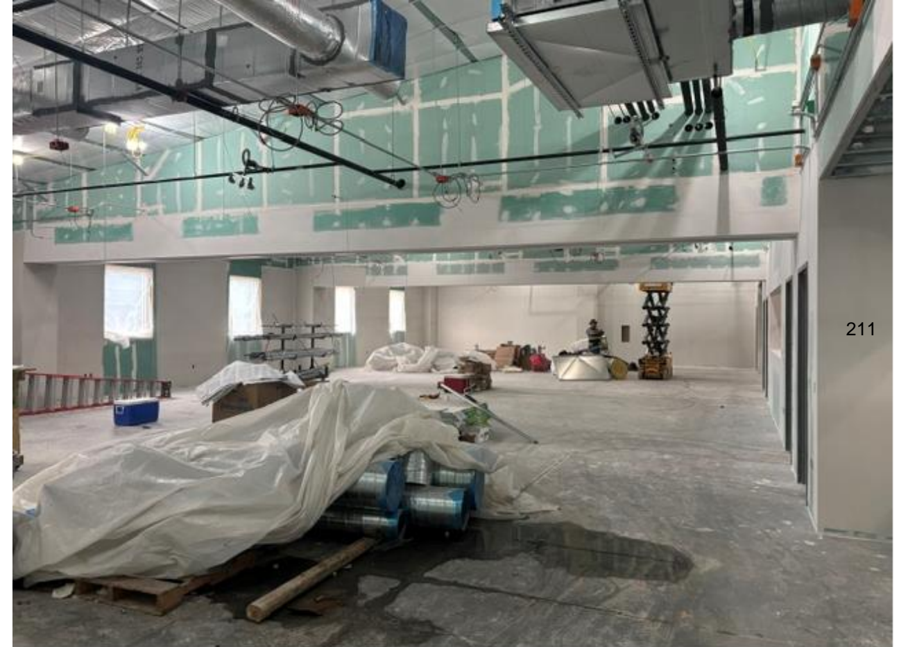
Primer coat of paint being applied at the Ag Science Center
