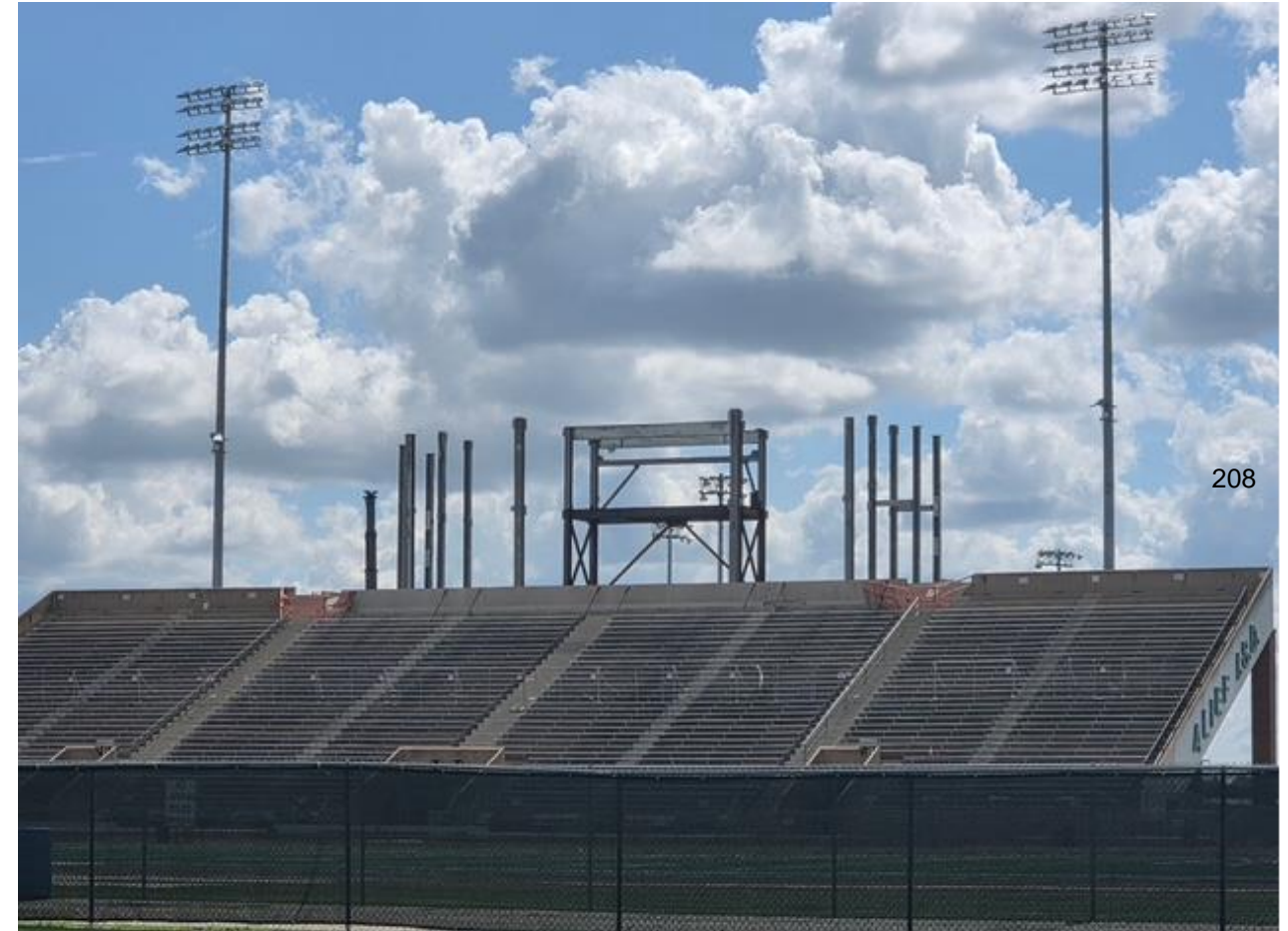
New stadium lights have been installed
