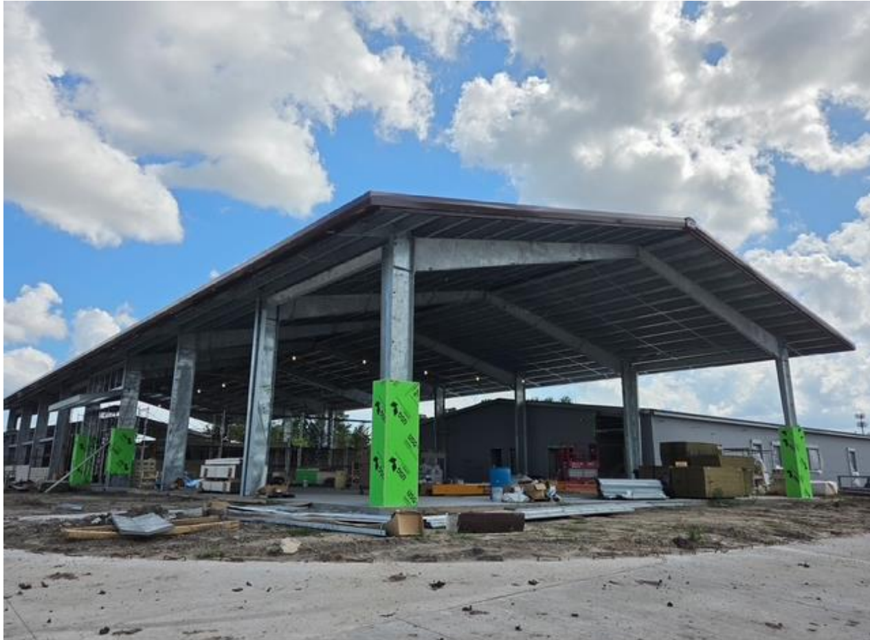
Exterior sheathing being installed at columns – Show Arena
