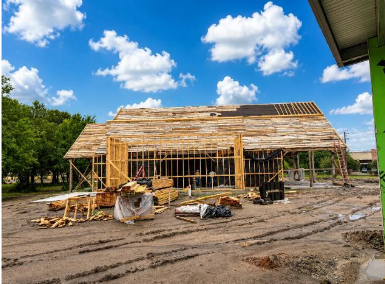
Framing out of restrooms – Outdoor Learning Building
