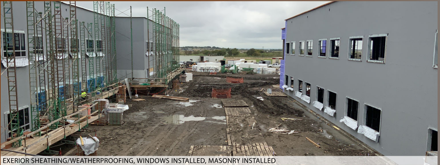
EXTERIOR SHEATHING/WEATHERPROOFING, WINDOWS INSTALLED, MASONRY INSTALLED
