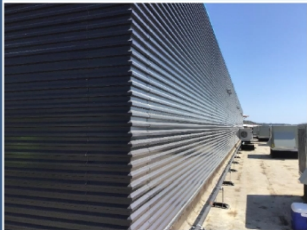
Area G Metal Wall Panels
