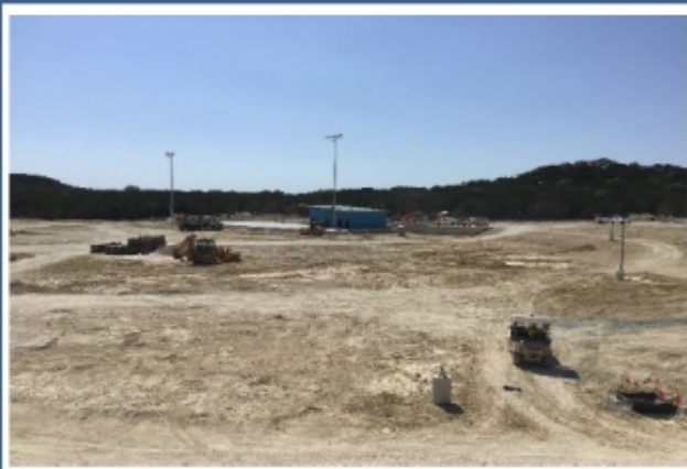
Football Field Concessions Looking South
