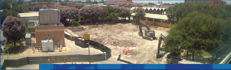
Topping Out for the H-E-B Black Box Theater (Watson Fine Arts Center)
