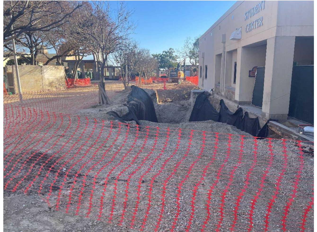
Trench collapse on east side of building
