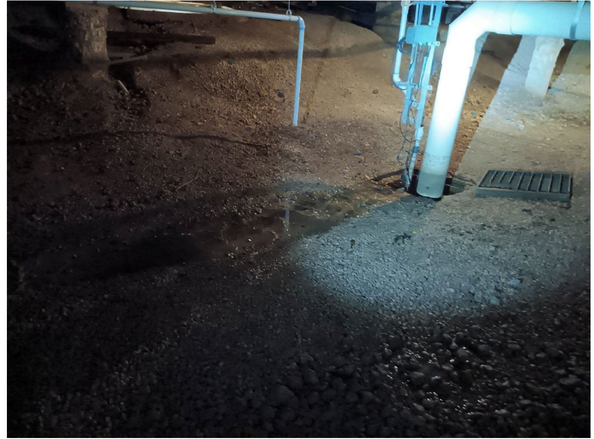
UNDERFLOOR SUMP PUMP LOCATION
