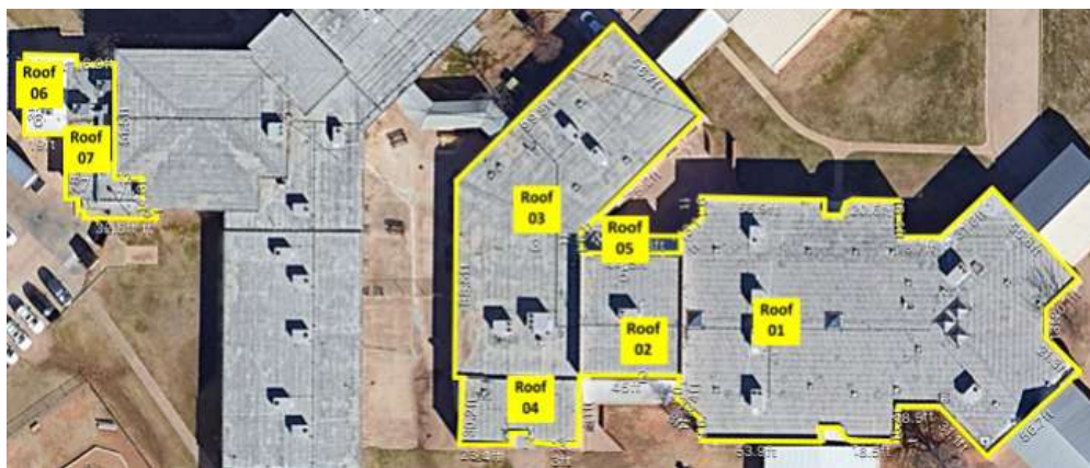
Cunningham Elementary School Wichita Falls, TX
