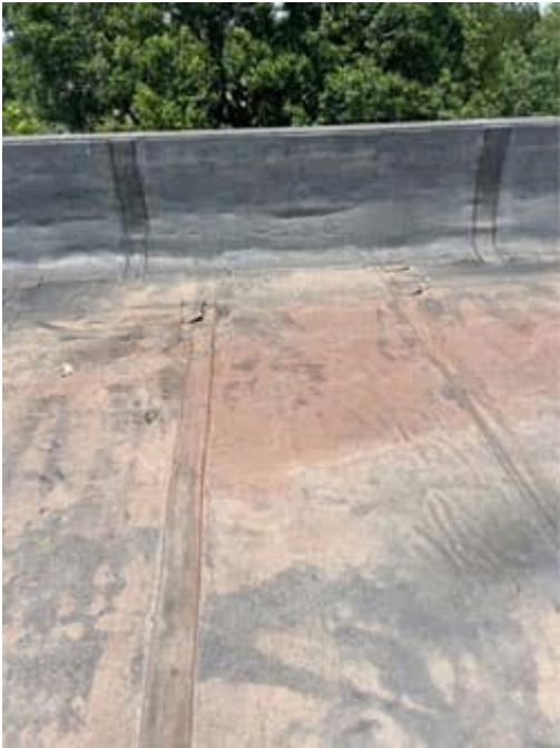
Ponding/shrinking
