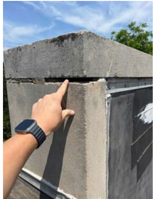
Opening in masonry
