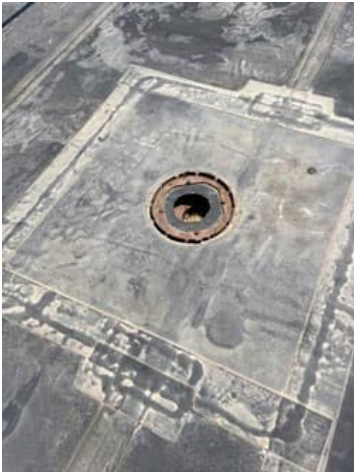
Exposed drain
