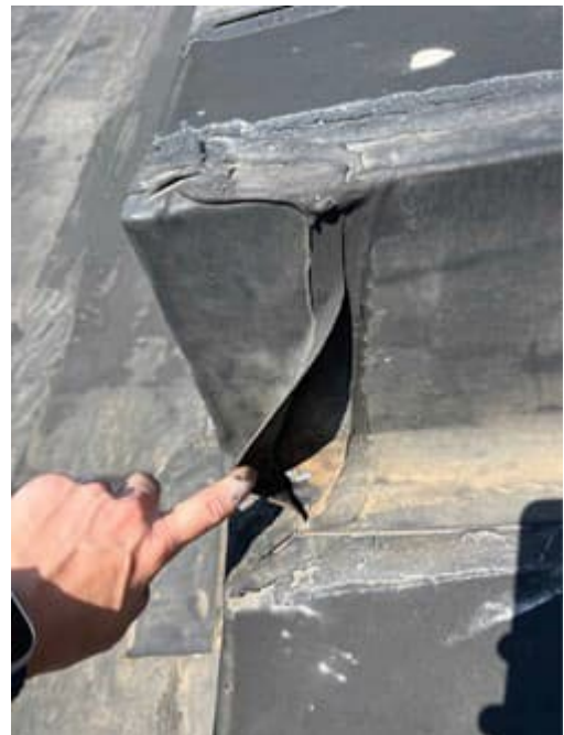
Opening on parapet
