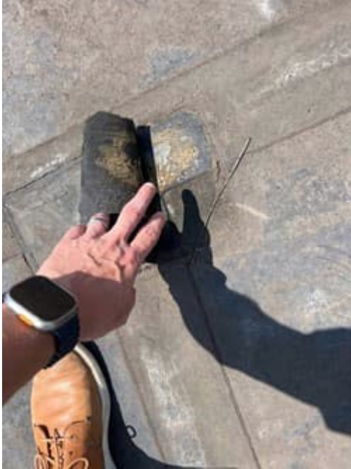
Failing Lap
