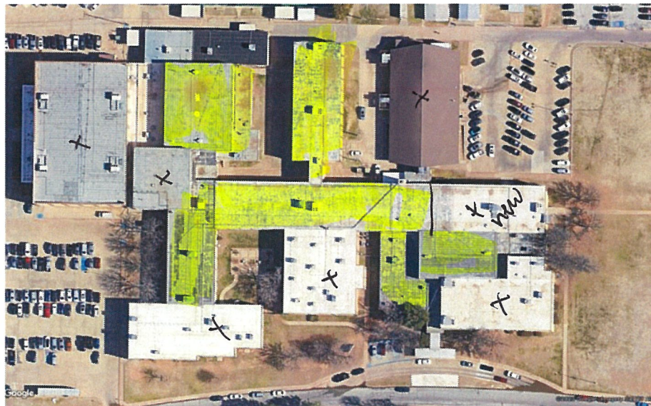
Wichita Falls ISD – Rider High School Wichita Falls TX-Roofs 1-10
