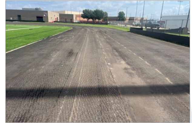
Travis HS Track Resurfacing
