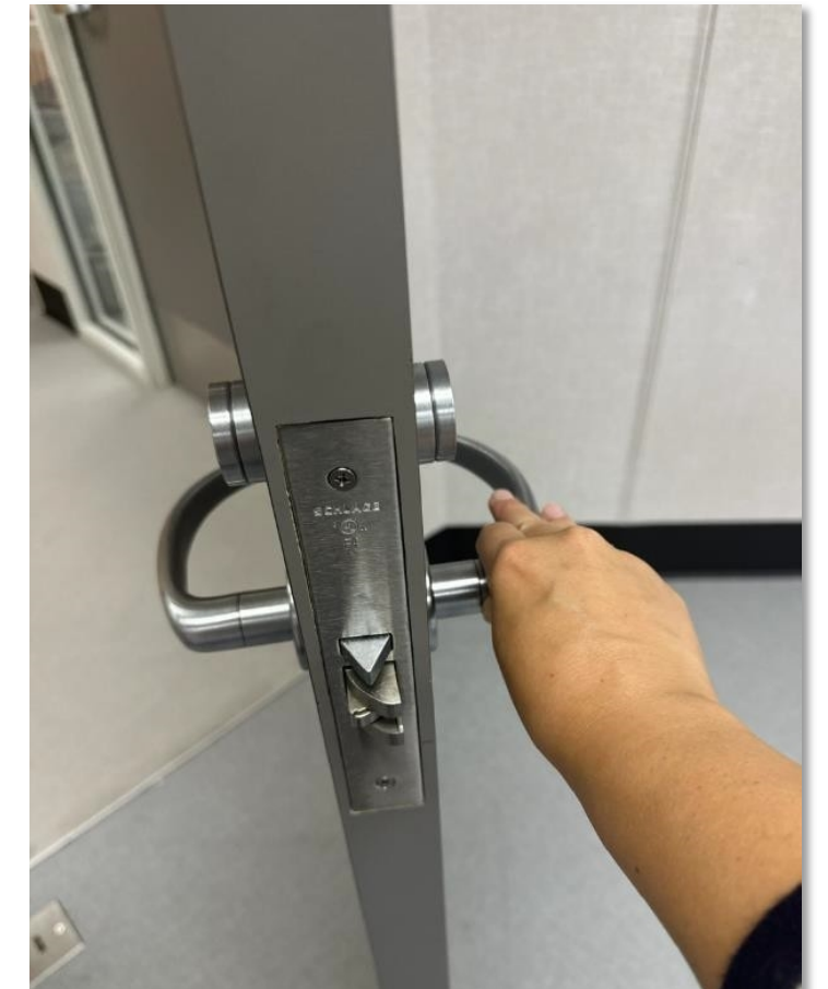
Images of Major Building Systems Captured during Assessments
