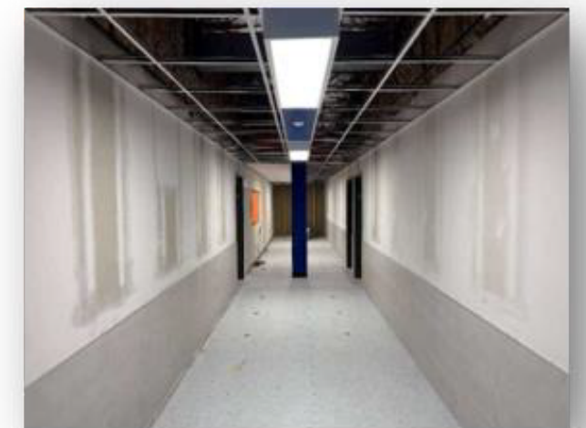
Construction Progress at Lantern Lane ES, Receiving Improvements from 2023 Bond
