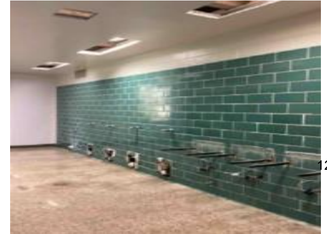
BP027 Restroom Renovations
