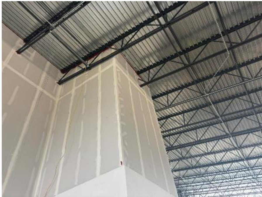
Drywall Installation
