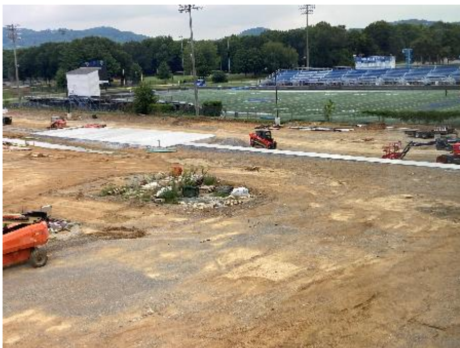
Multi-purpose Field Sidewalk and Bleacher Pad
