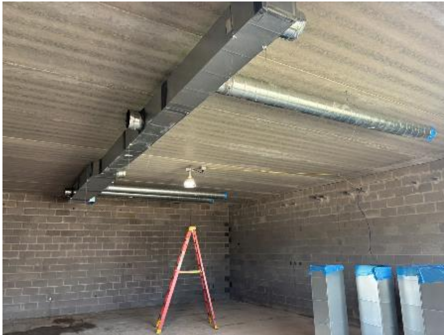
Duct installation
