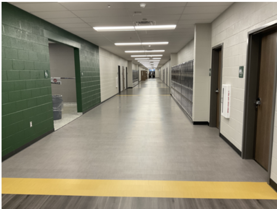
1 st Floor Corridor
