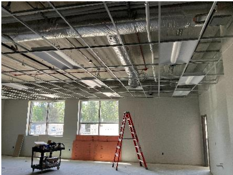
Ceiling Grid and Lighting
