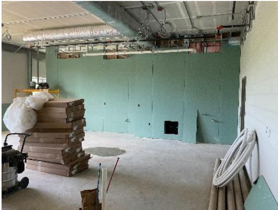
Third floor drywall installation
