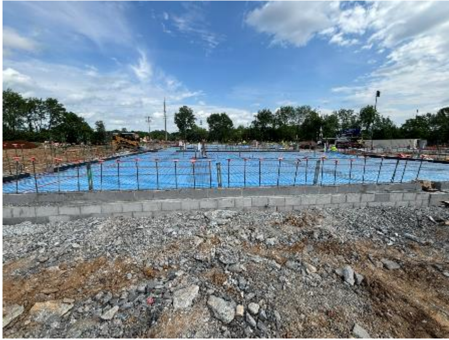
Concrete Slab Prep
