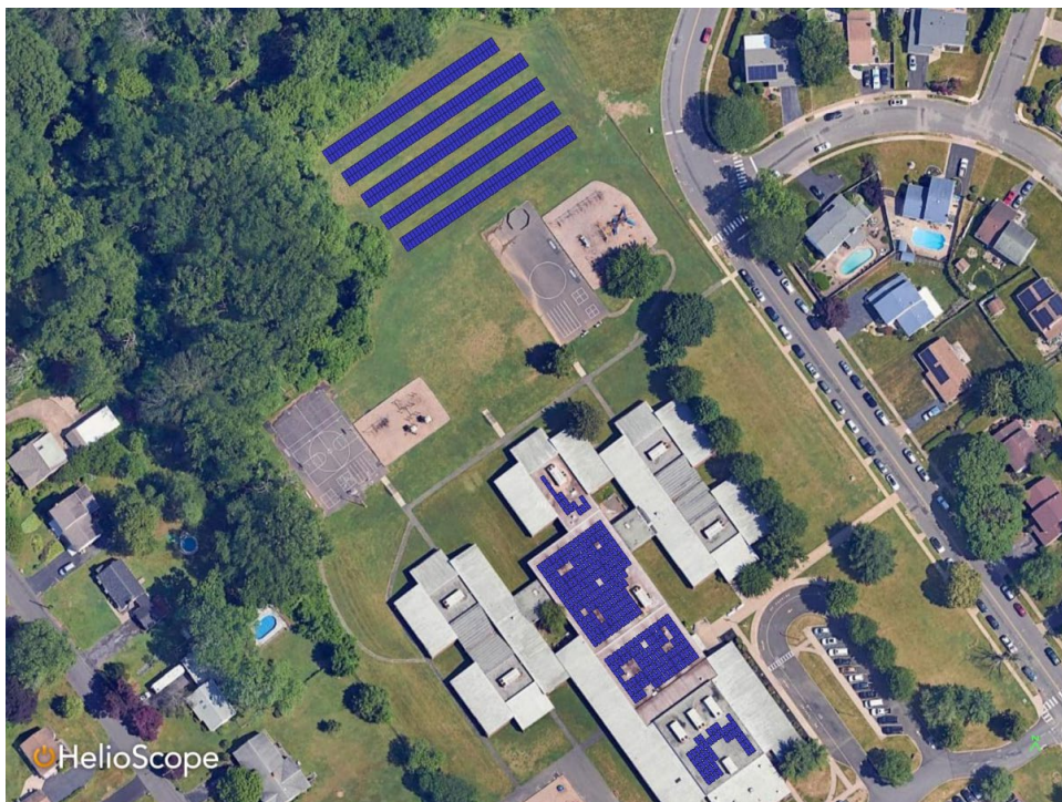
Belmont Elementary Ground 322 kW (3%)
