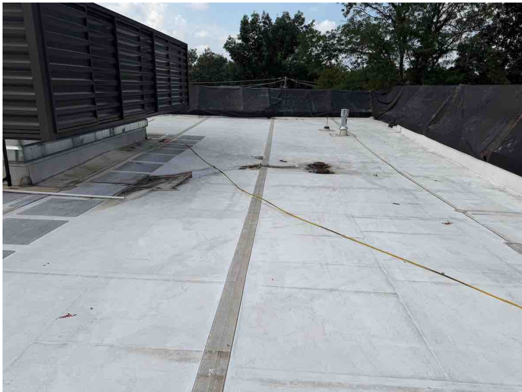
#28 -- Section A: Overview of section facing west. [2601301R0028.jpg]
