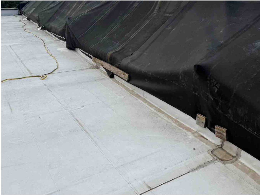
#15 -- Section A: Overview showing west perimeter parapet tarped off for facade repair. Note, tarp fastened through the base flashing, will need repair. [2601301R0015.jpg]
