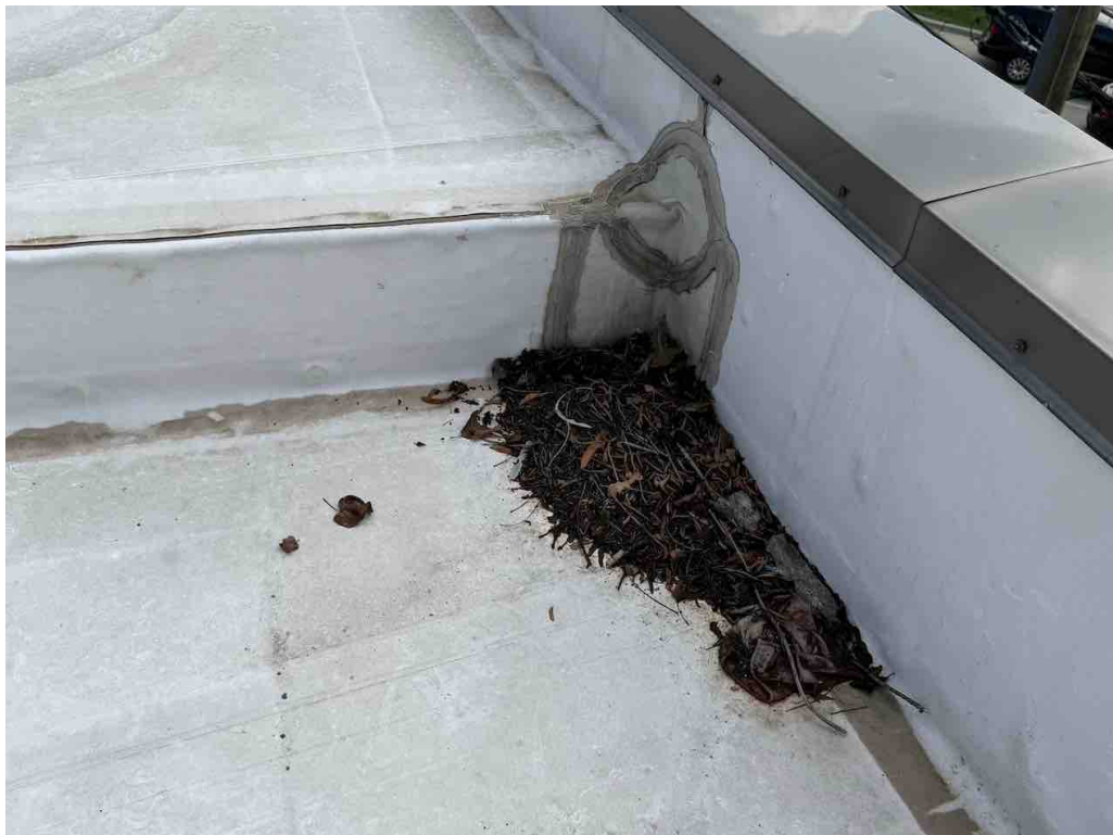
#20 -- Section A: Overview showing some tree debris in the corner. [2601301R0020.jpg]
