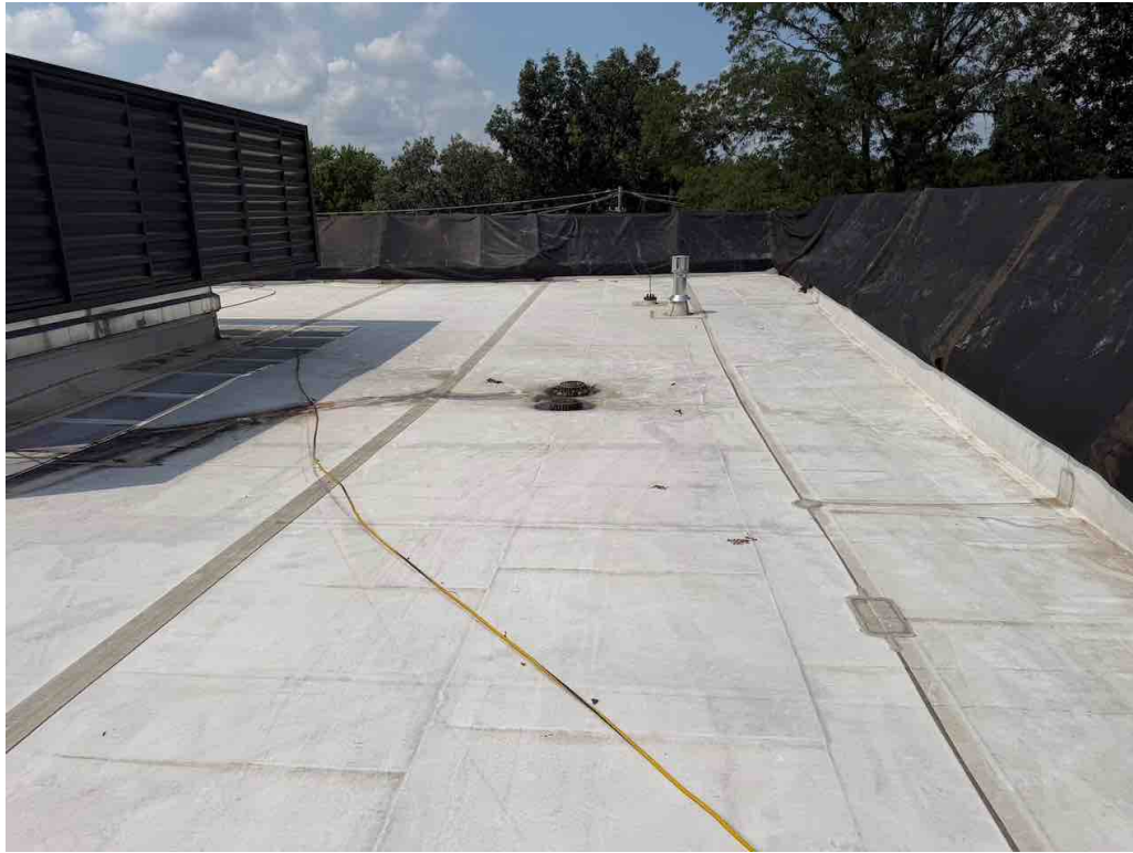
#7 -- Section A: Overview of section facing west. [2601301R0007.jpg]
