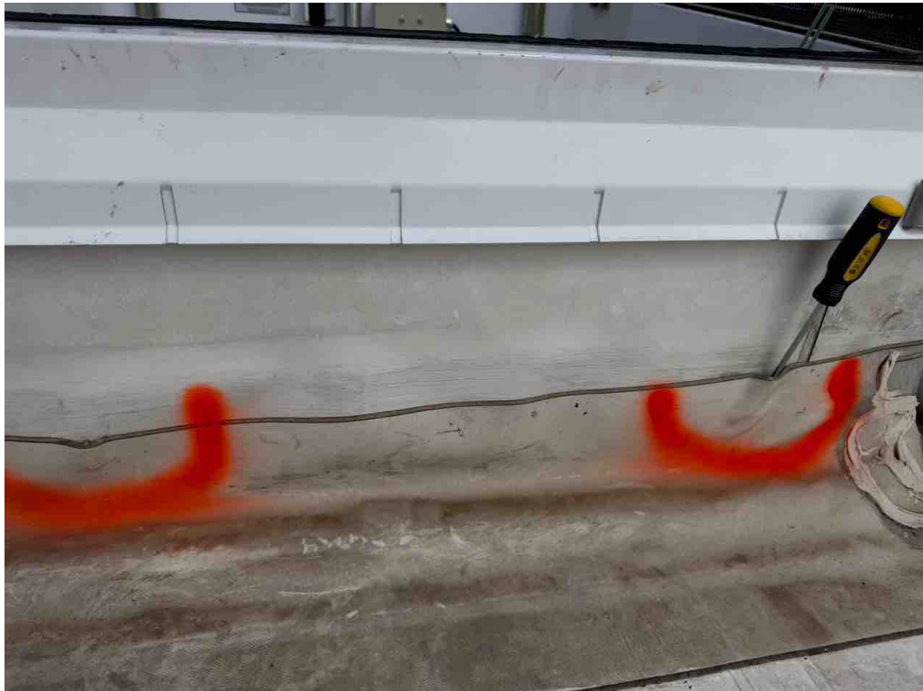
#10 -- Section A: Close-up showing roof hatch flashing open at the top. [2601301R0010.jpg]
