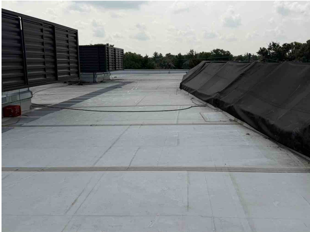
#13 -- Section A: Overview of section facing south. [2601301R0013.jpg]
