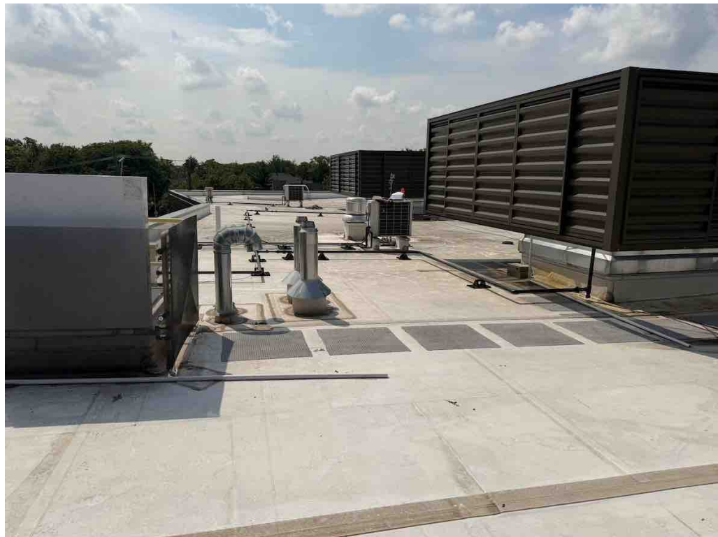
#6 -- Section A: Overview of section facing south. [2601301R0006.jpg]
