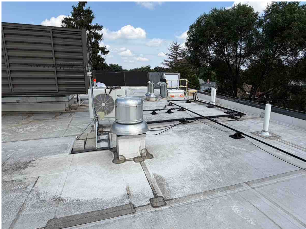
#24 -- Section A: Overview showing membrane patches and equipment. [2601301R0024.jpg]
