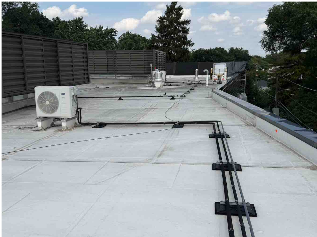
#22 -- Section A: Overview of section facing north. [2601301R0022.jpg]
