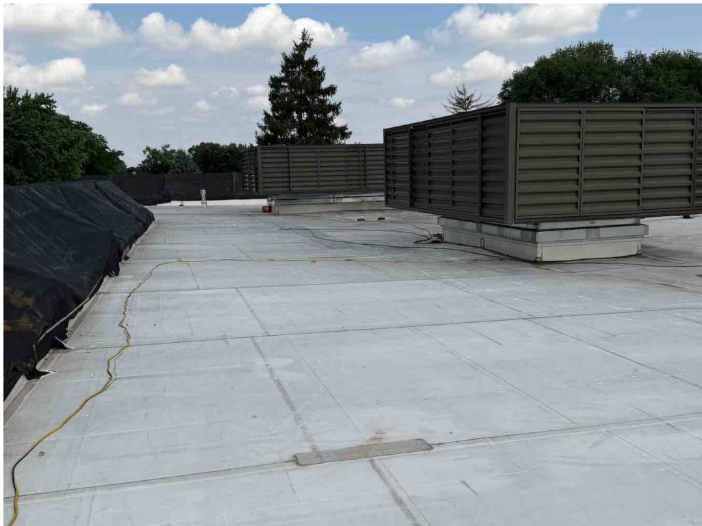
#16 -- Section A: Overview of section facing north. [2601301R0016.jpg]
