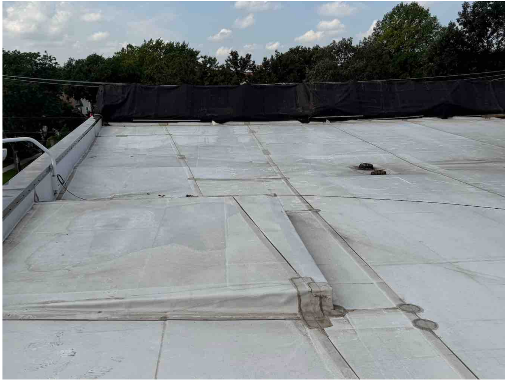
#21 -- Section A: Overview of section facing west. [2601301R0021.jpg]
