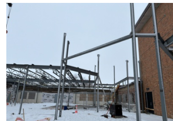
Figure 7 Steel at the new entrance
