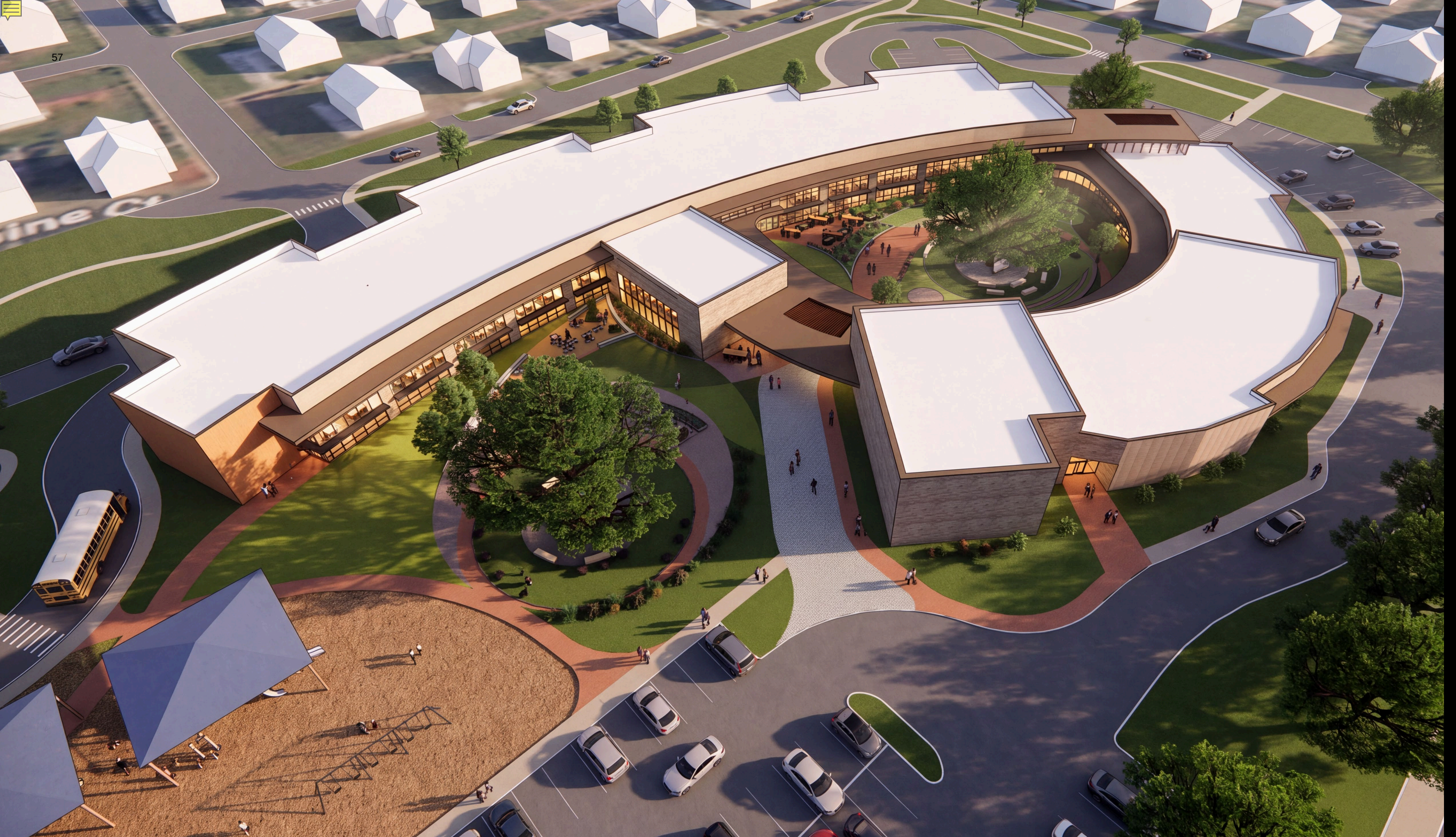
BACK ENTRY AERIAL
