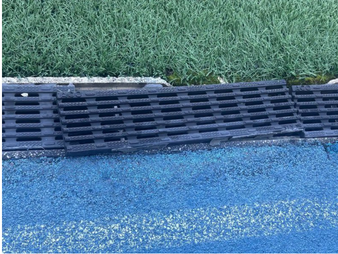
Existing stadium drainage
