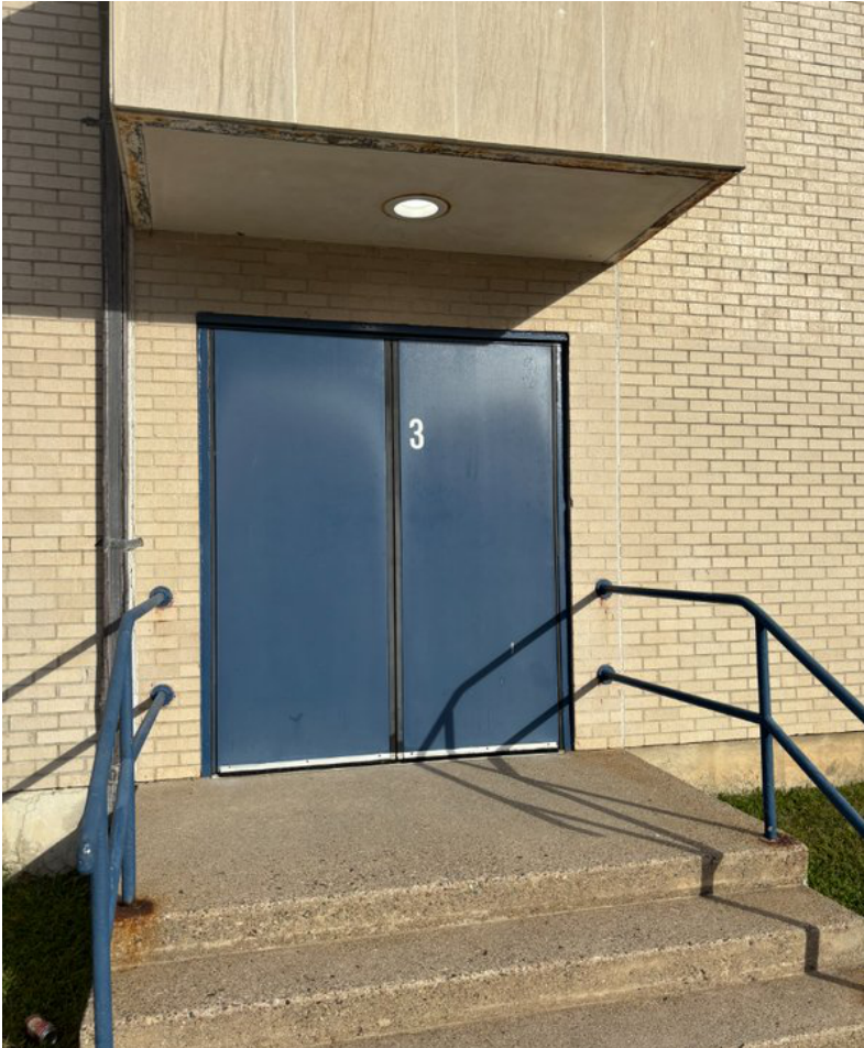
Existing exterior door condition
