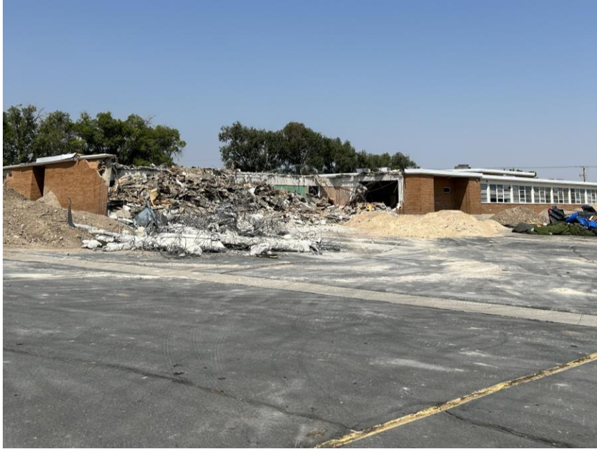
Start of demolition
