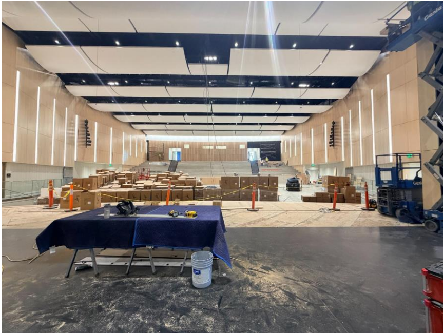
Auditorium paneling progress
