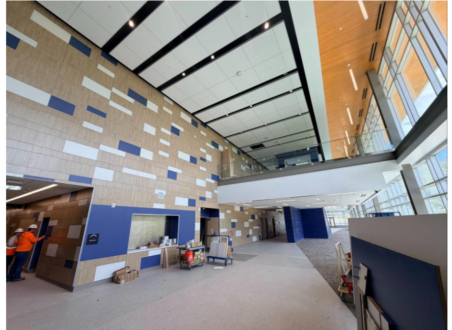
Performing Arts entry progress
