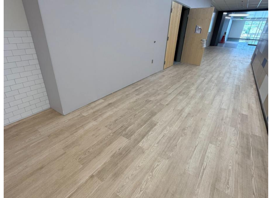
Corridor LVT progress
