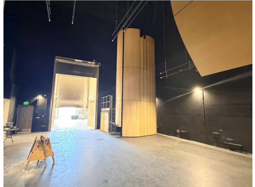
Fly Loft orchestra shell installation
