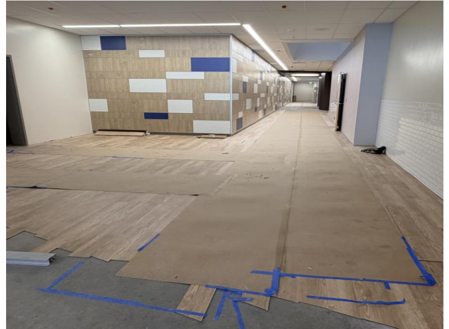
Corridor LVT being installed and protected
