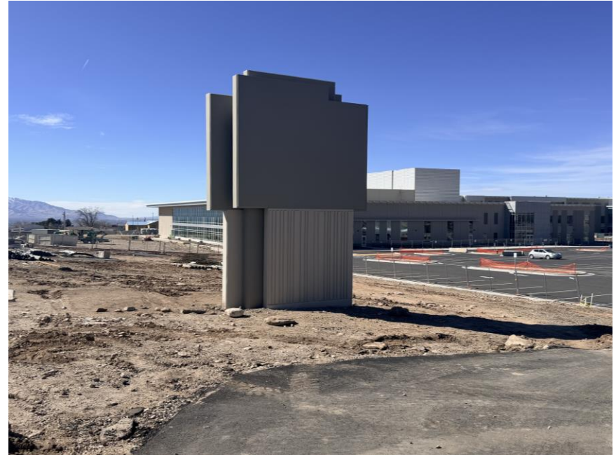
Marquee painted, power & fiber being installed
