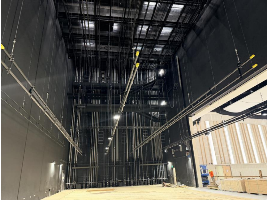
Stage rigging complete
