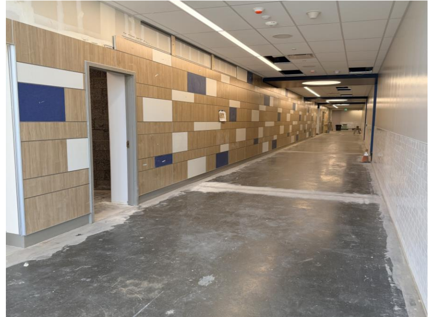
Auditorium corridor wood paneling installation
