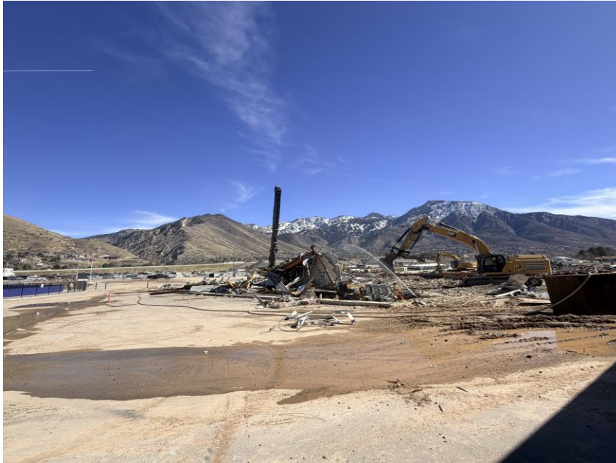
Old Performing Arts demolition complete
