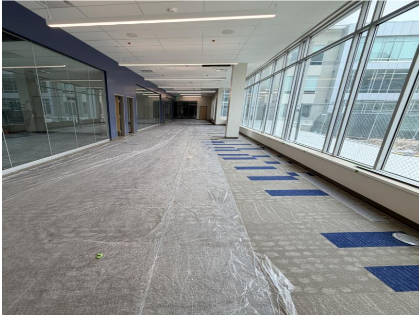
Area H Classroom Pods nearly complete
