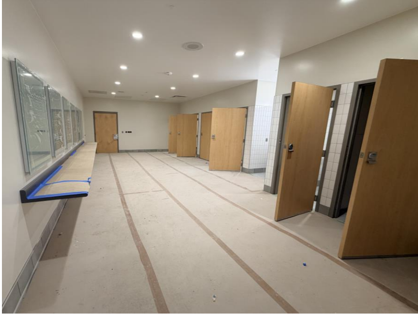
Dressing Room countertops installed
