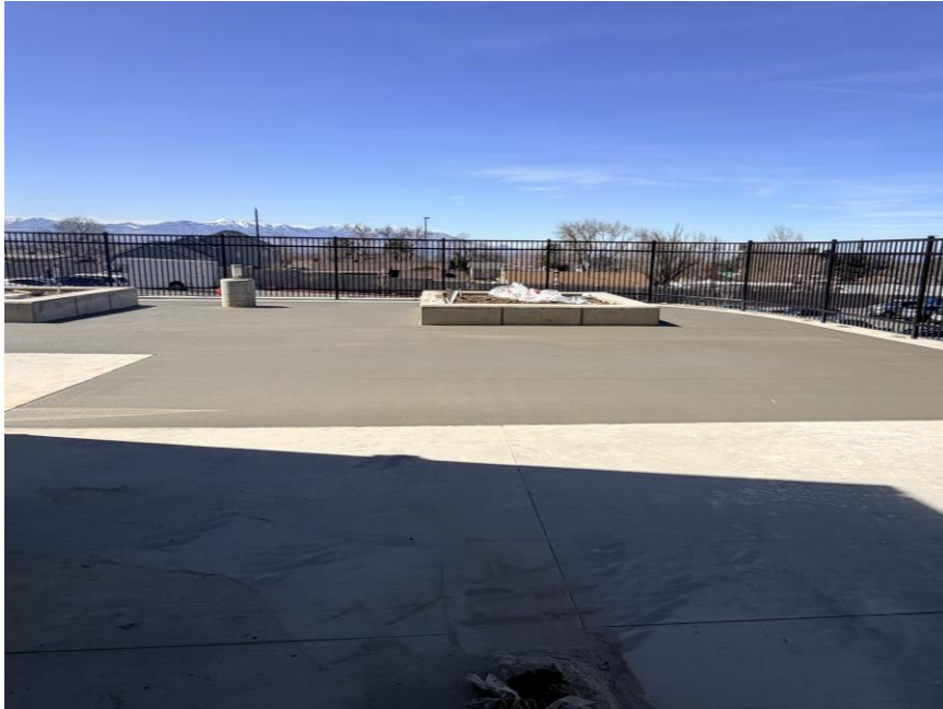
Patio concrete replaced where Air Handler-12 was removed 24
