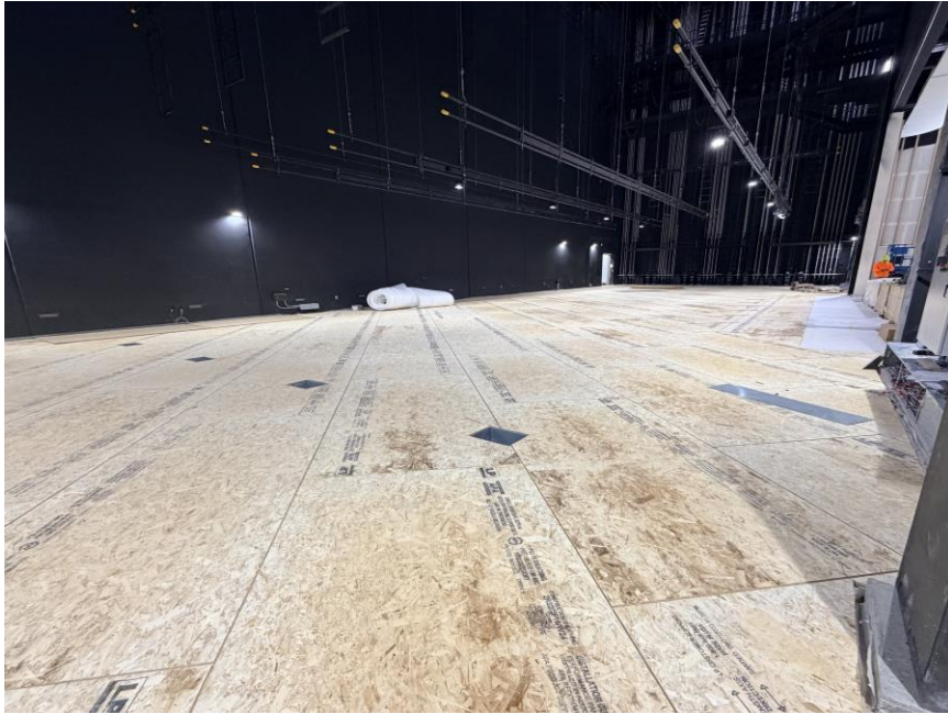
Stage floor installation
