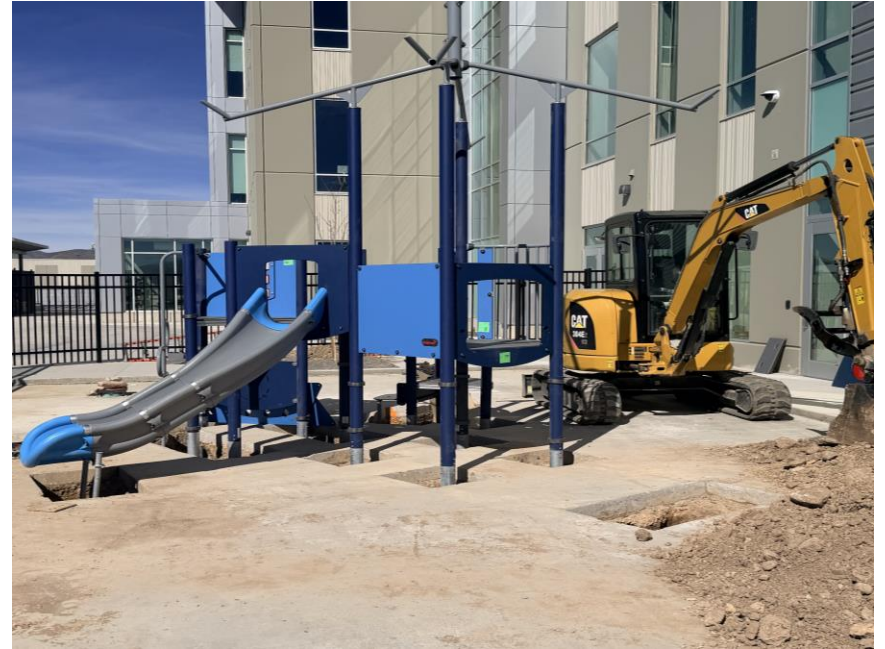
Preschool playground equipment installed
