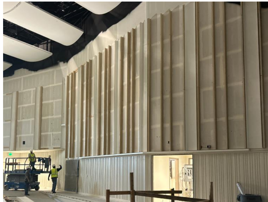
Auditorium west wall
