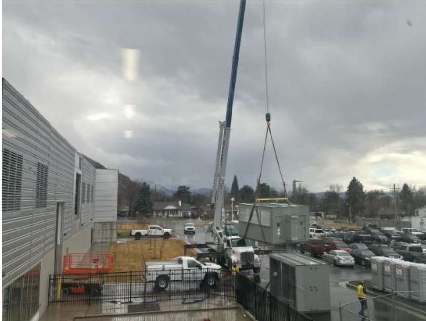
Air handler being moved into place
