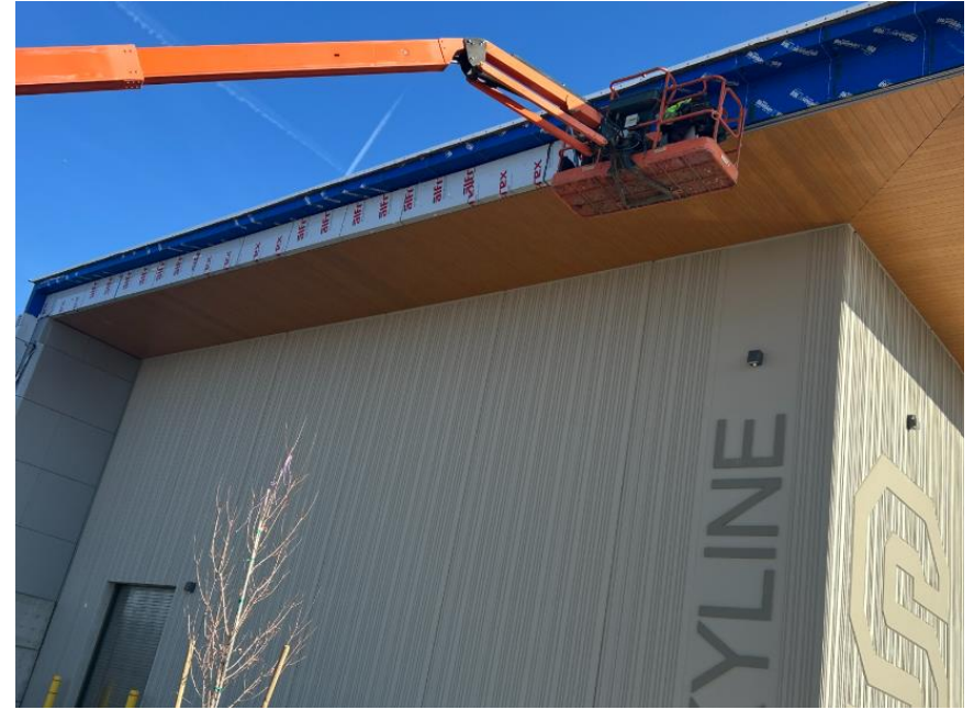
Auditorium southwest elevation progress
