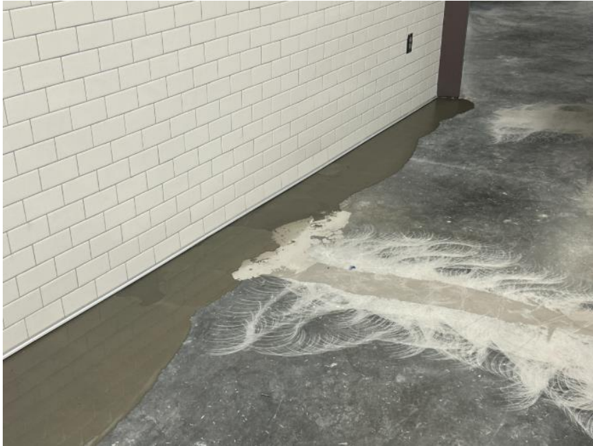
Floor prep griding, patching, and leveling
