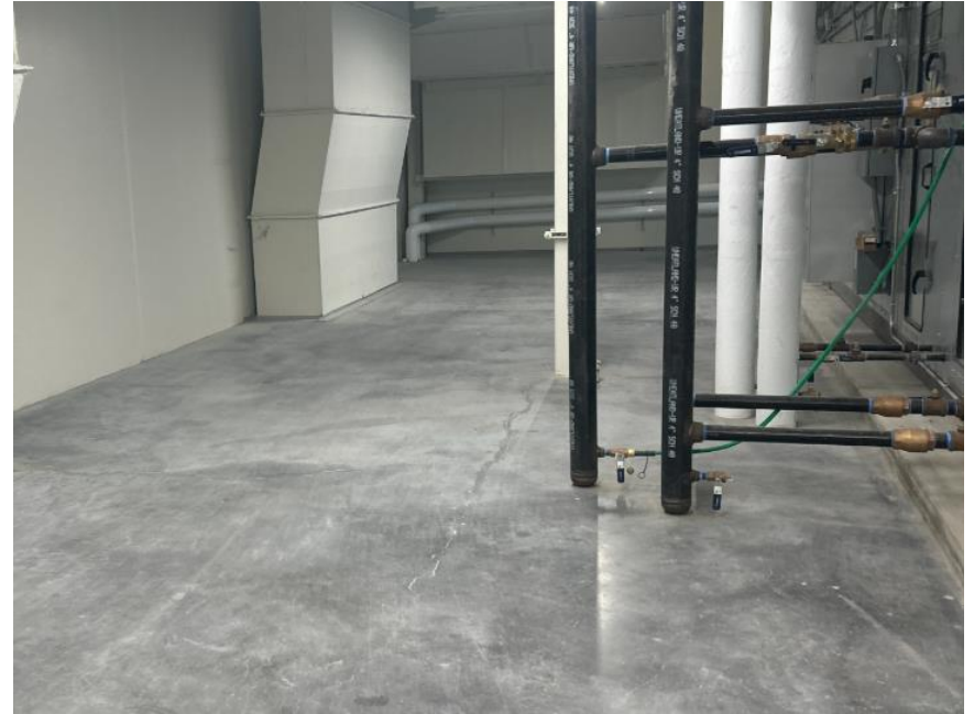
Mechanical Room concrete floor cleaned
