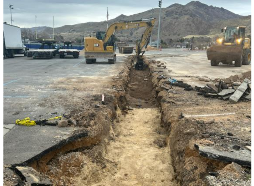
Water line installation
