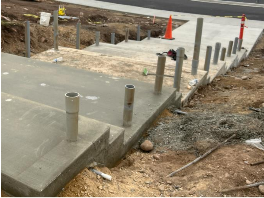
Concrete stair progress
