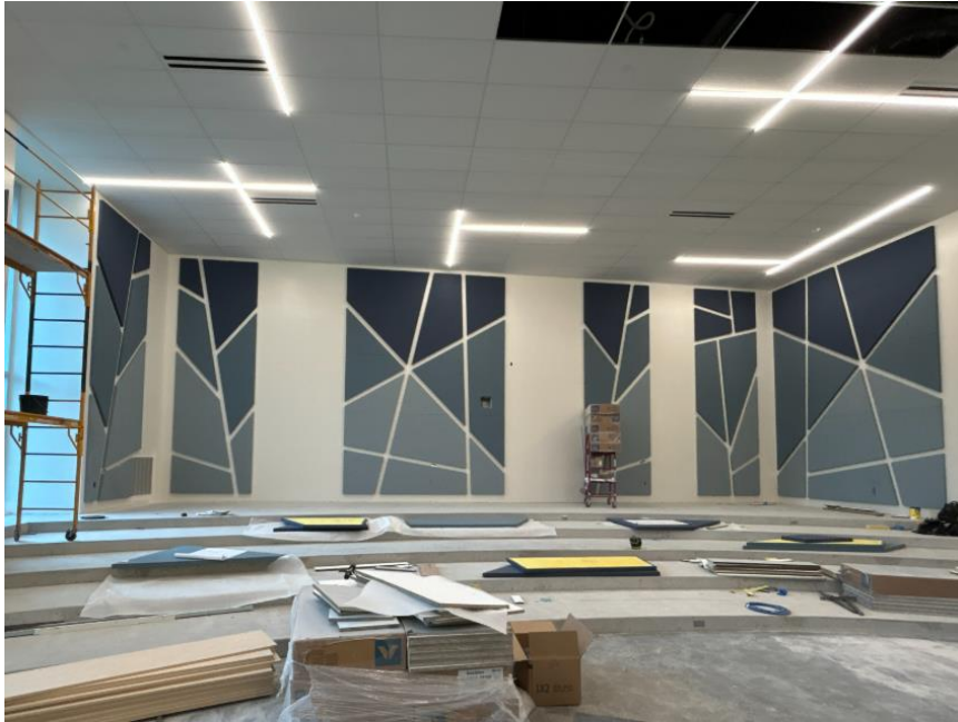
Choral Room progress
