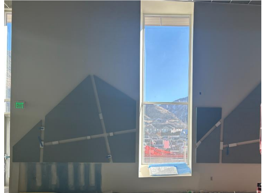
Band Room progress
