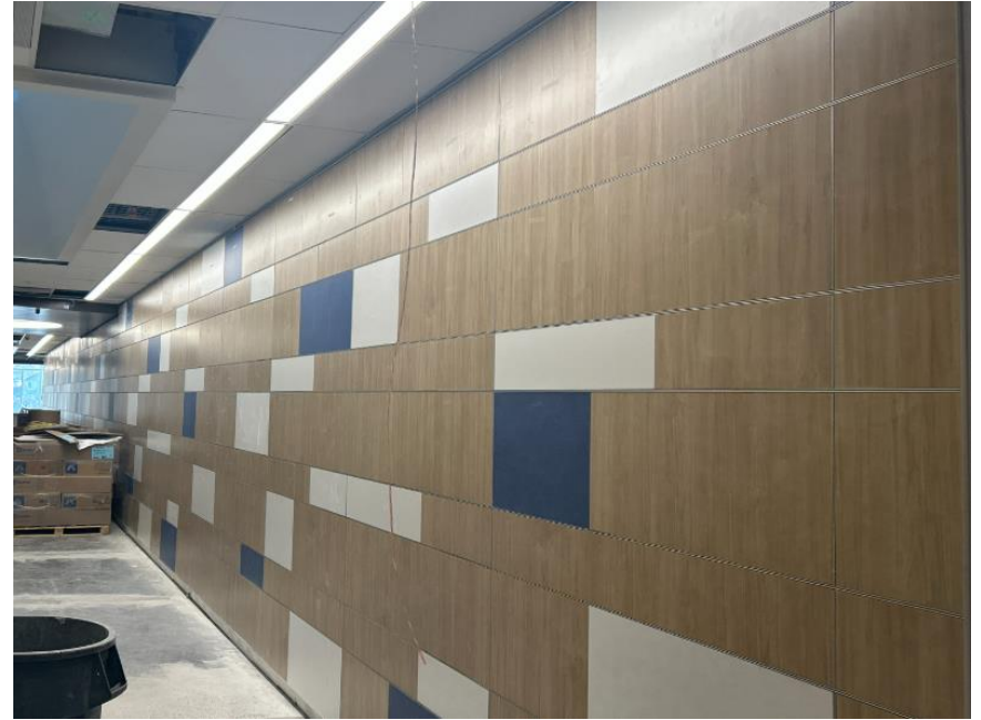
Corridor paneling installation
