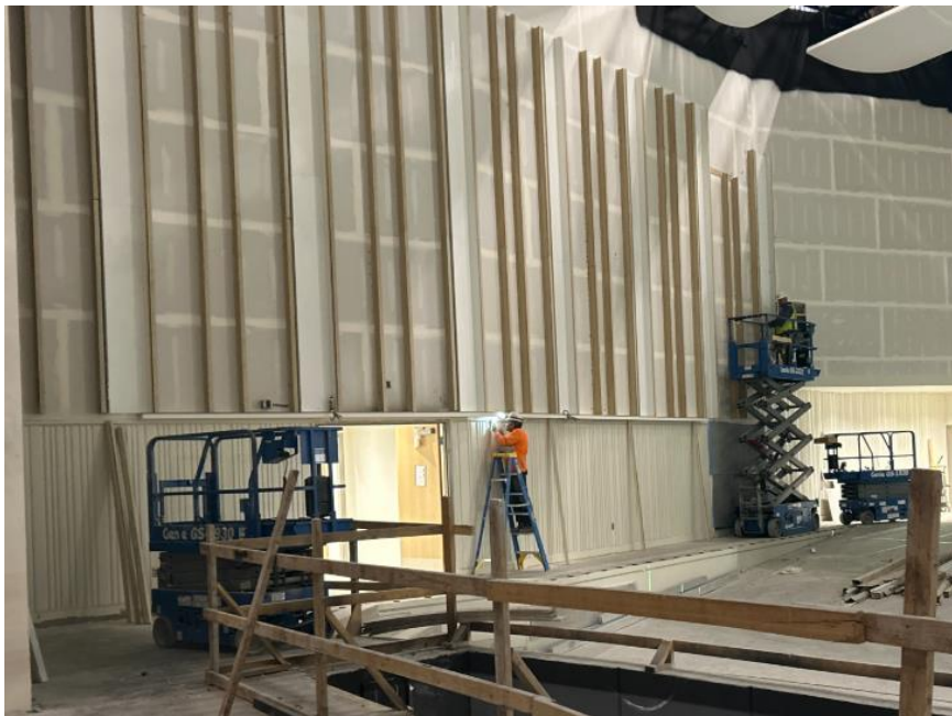
Auditorium east wall
