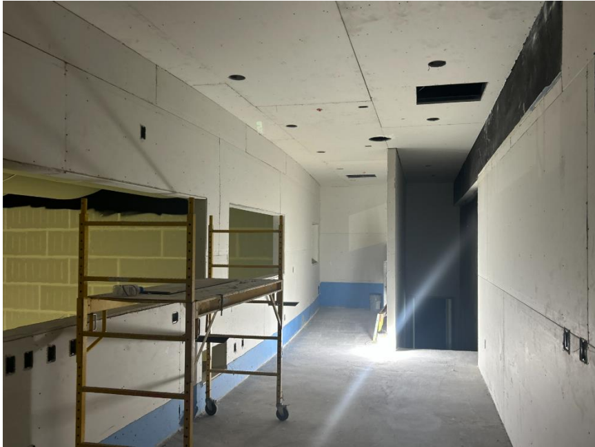
Auditorium Observation Room progress
