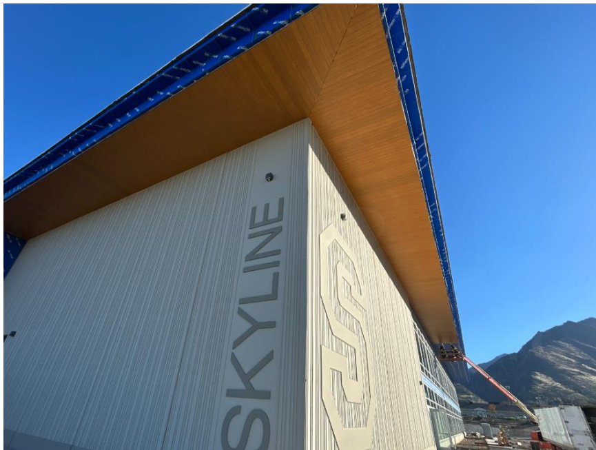
Soffit material installation
