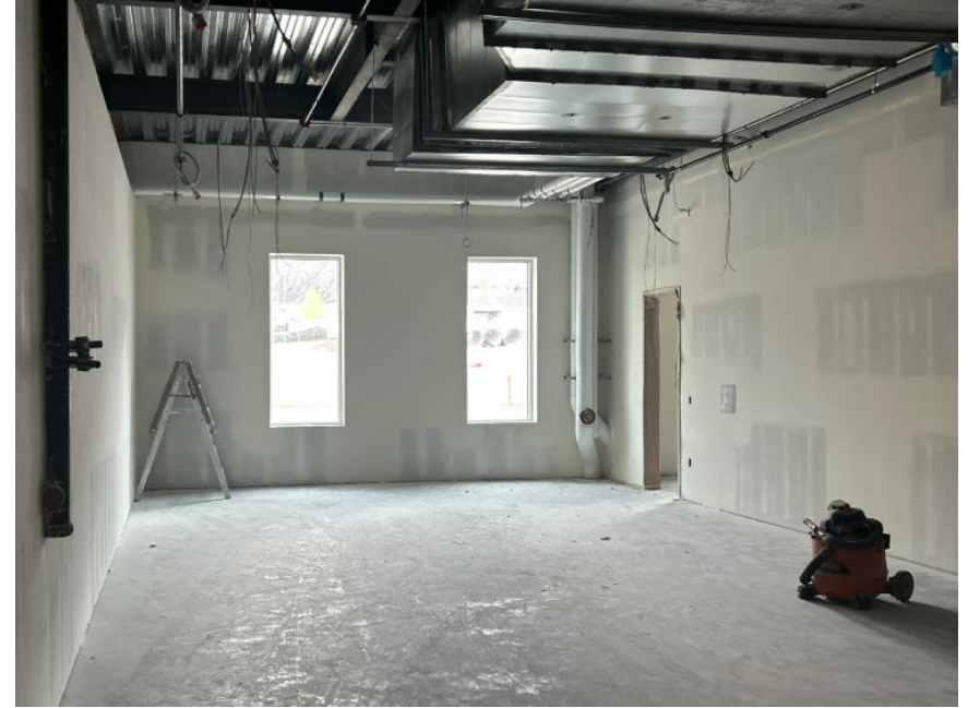
Instrument Room drywall progress
