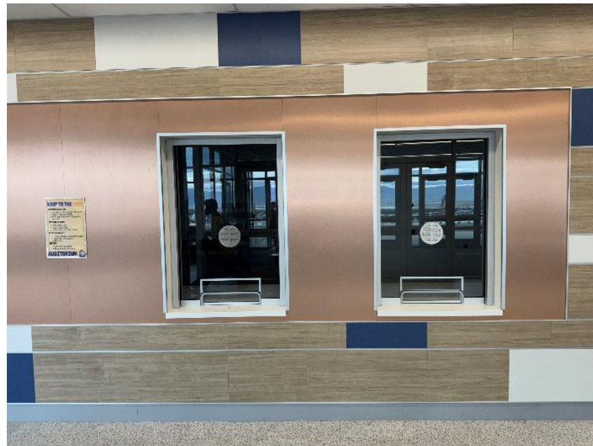
Performing Arts ticket booth windows installed
