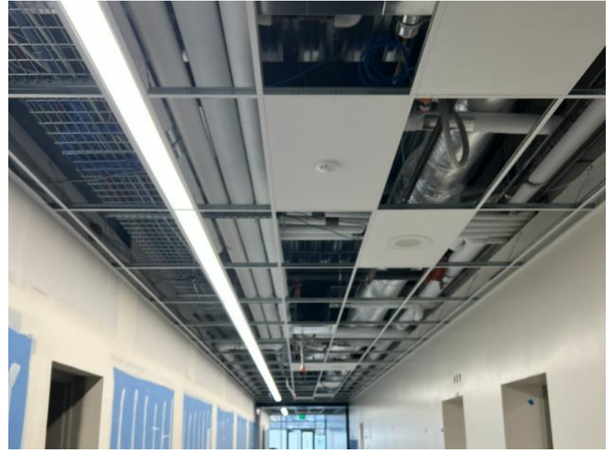
Ceiling light installation
