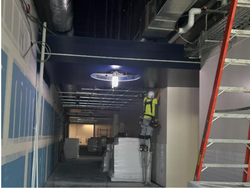
Ceiling grid installation progress
