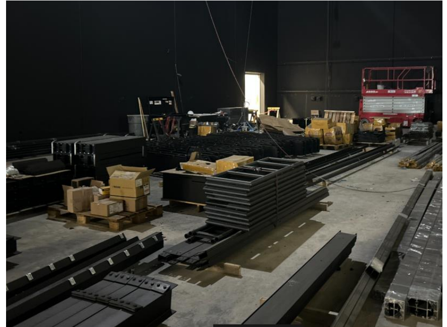
Fly Loft rigging delivery and installation
