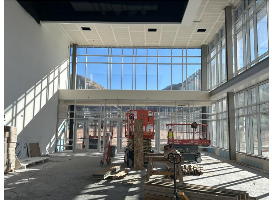
Auditorium East Entrance progress
