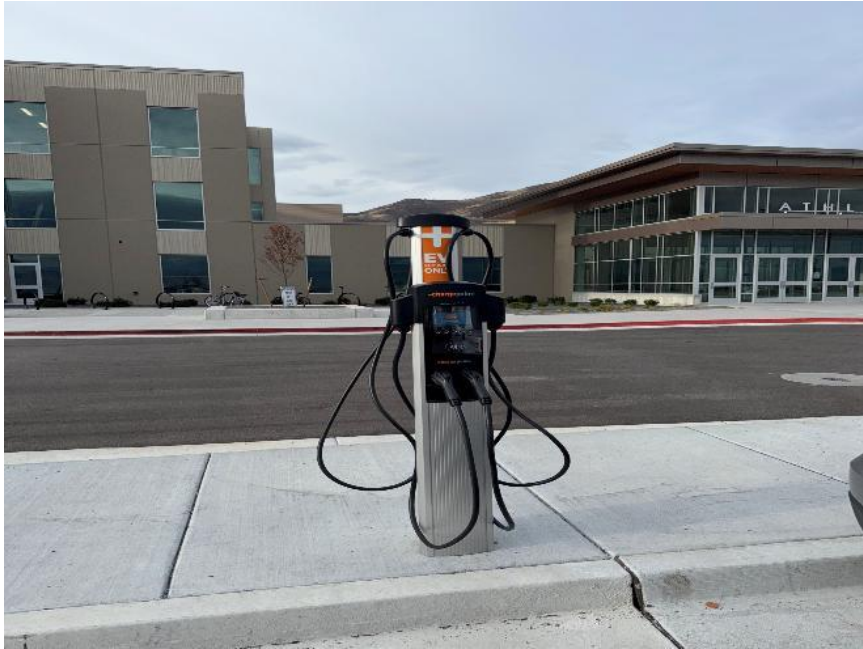
Electric vehicle charging station by GSD
