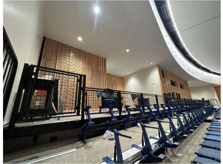
Handrail and carpet installed for the Auditorium Balcony
