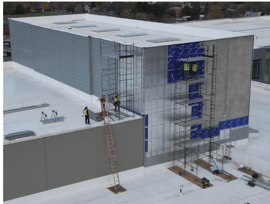
Exterior material installation progress
