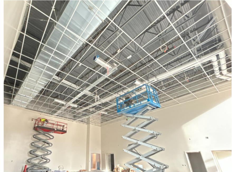
Choir Room ceiling grid install
