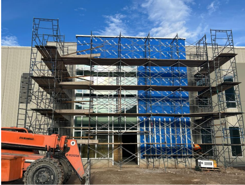
East Entrance elevation scaffolding
