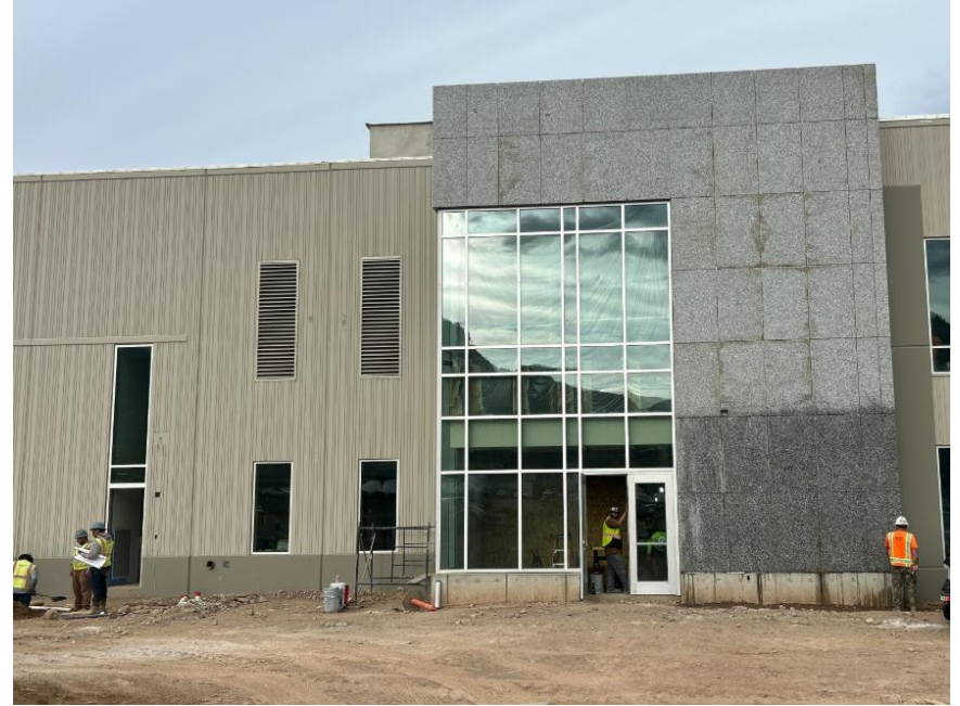
East Entrance elevation clean up
