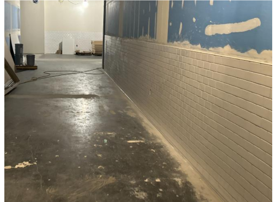
Wall tile progress
