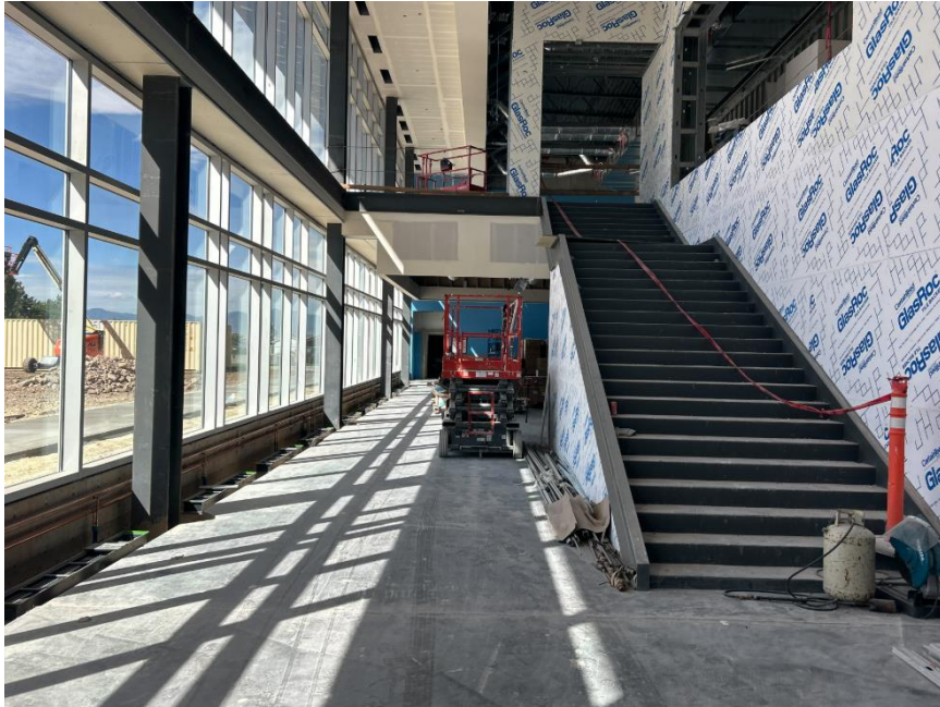
Auditorium stair progress
