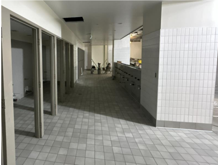
Restroom tile progress
