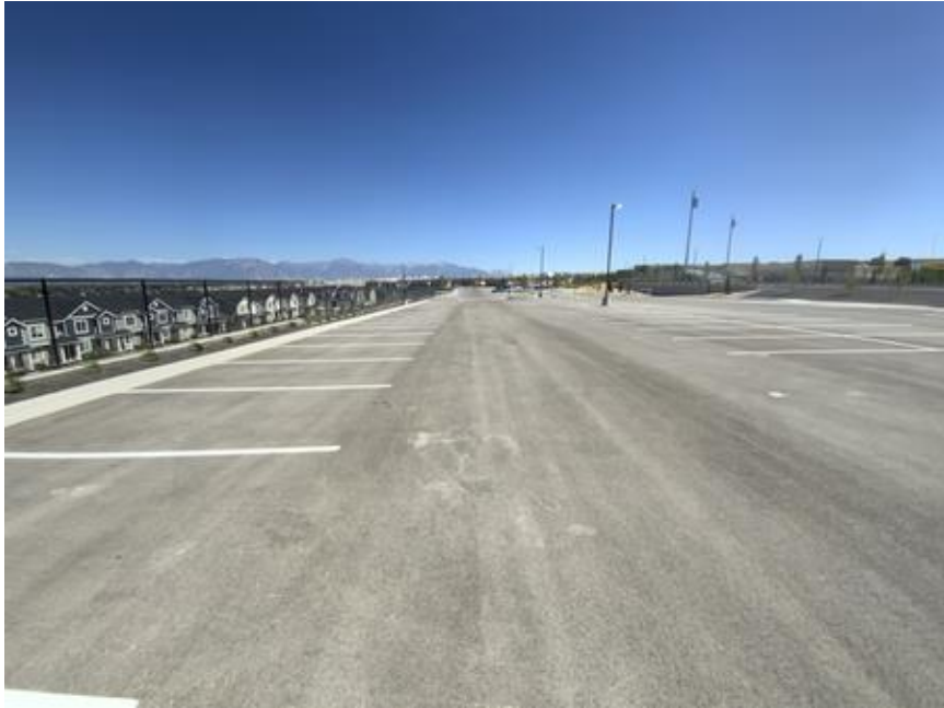
Parking lot striping
