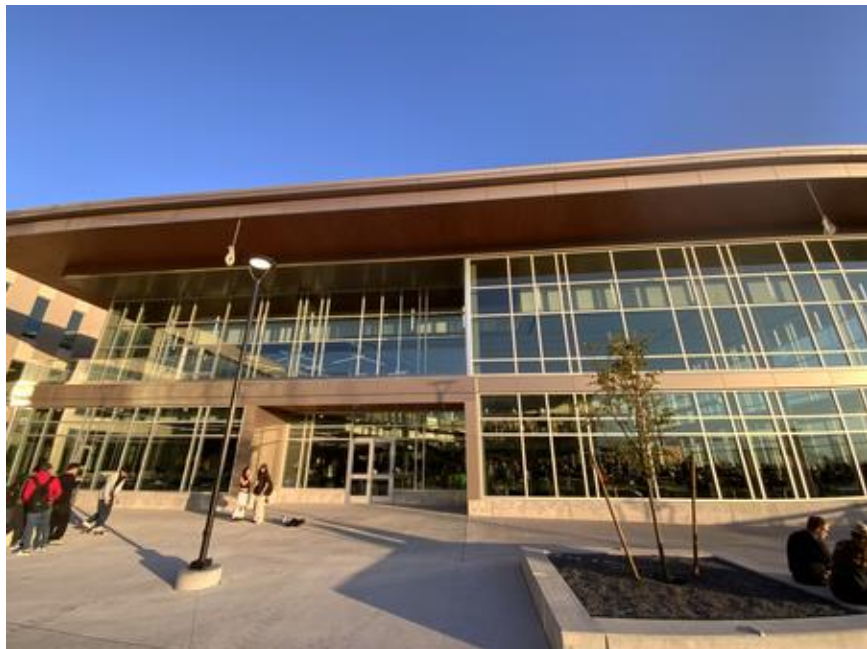
Exterior metal panels outside the Commons
