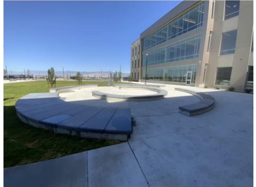
Precast seating in Courtyard
