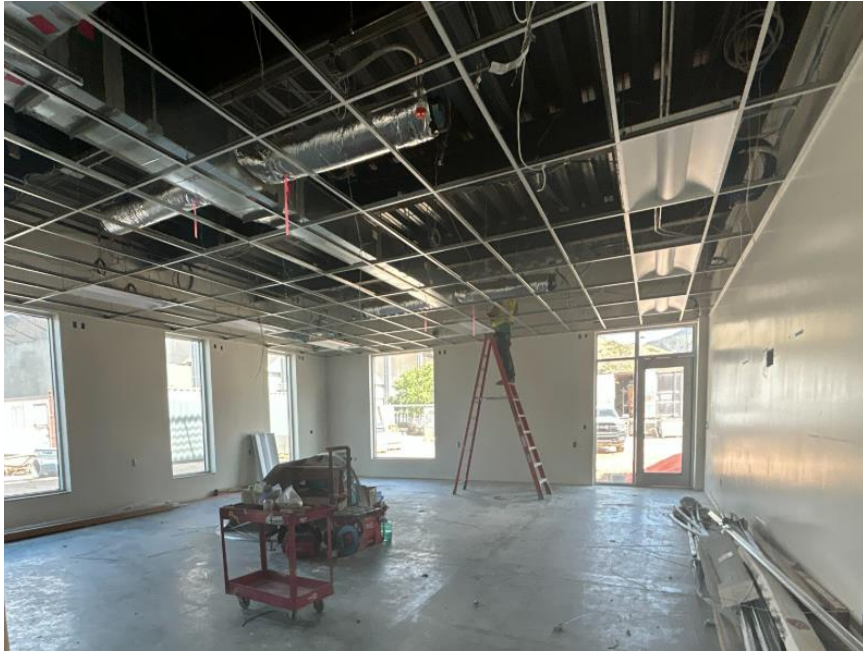
Classroom ceiling grid and light install
