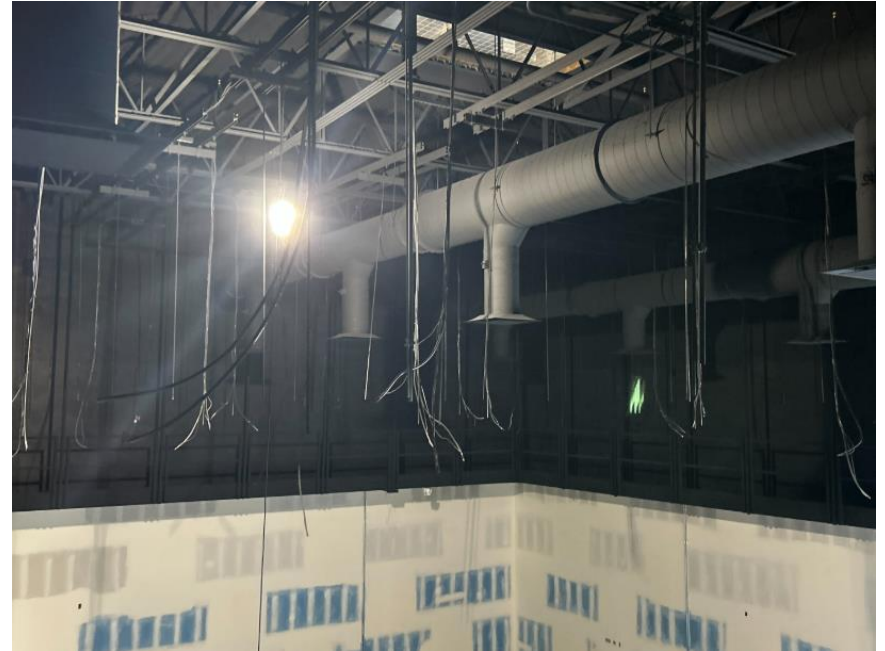
Black Box Theater progress
