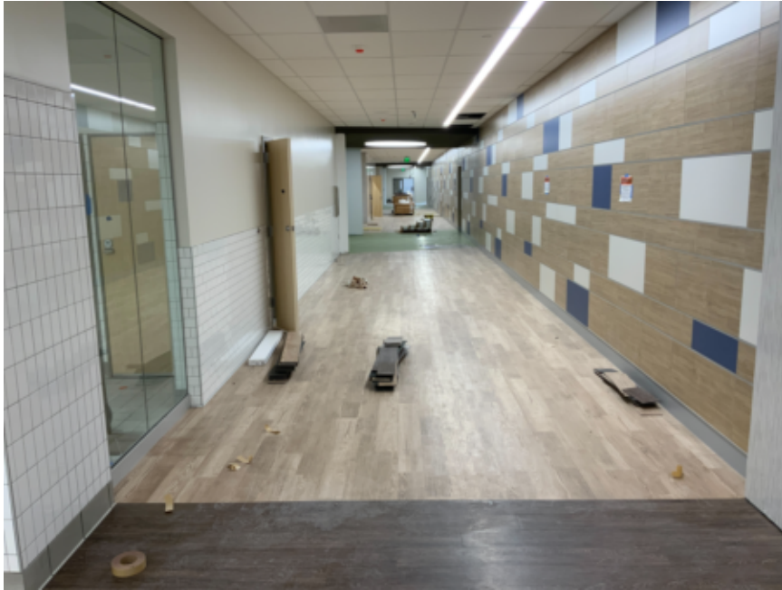
Flooring on Level 3
