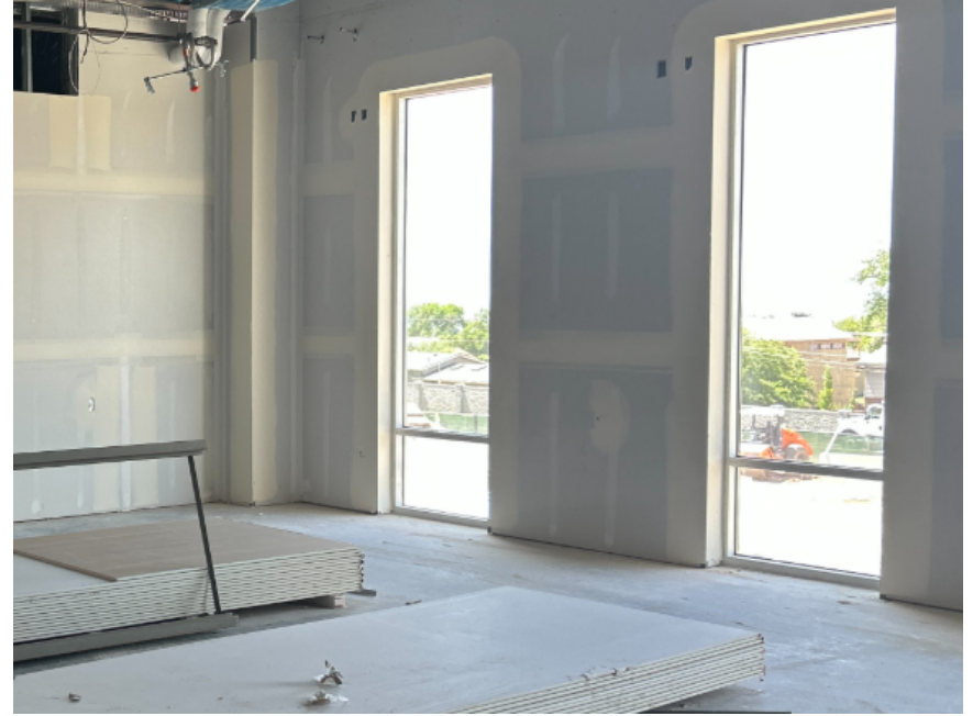
Drywall mud / tape progress
