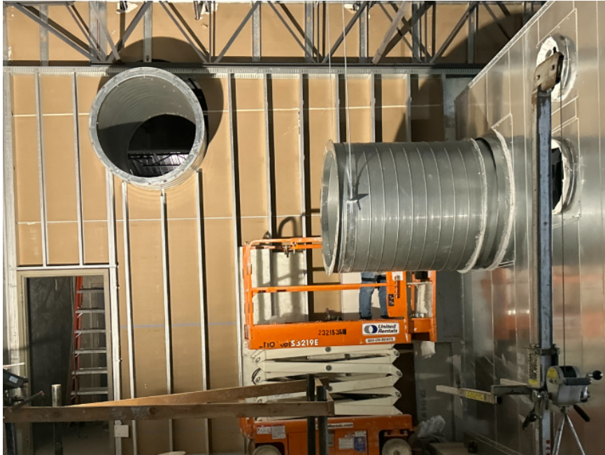
AHU 16 ductwork installation
