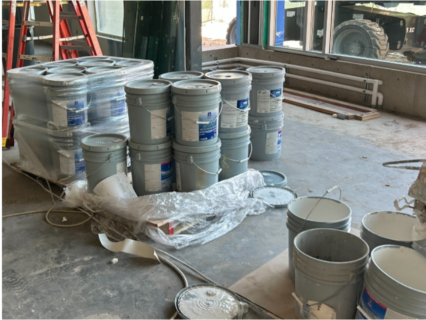
Painting material delivered to the project
