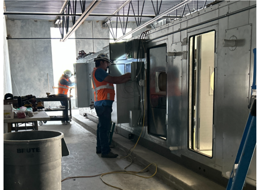
Crews wiring up AHU 17
