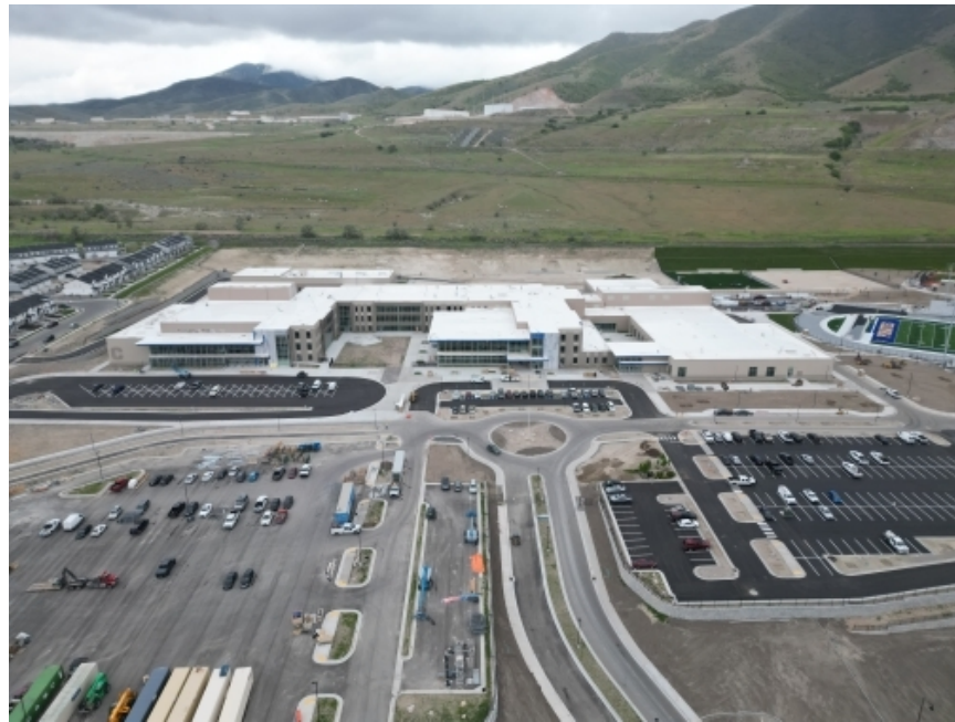
Parking lot striping
