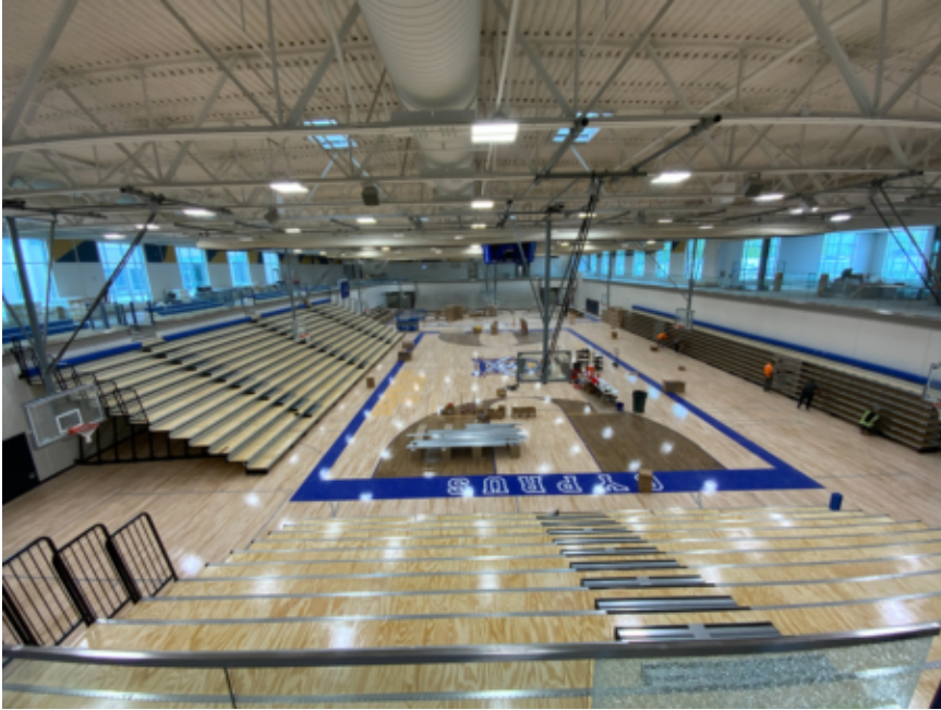
Basketball Court bleachers
