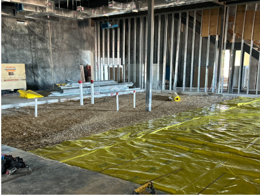
Sub-rough plumbing and interior concrete progress
