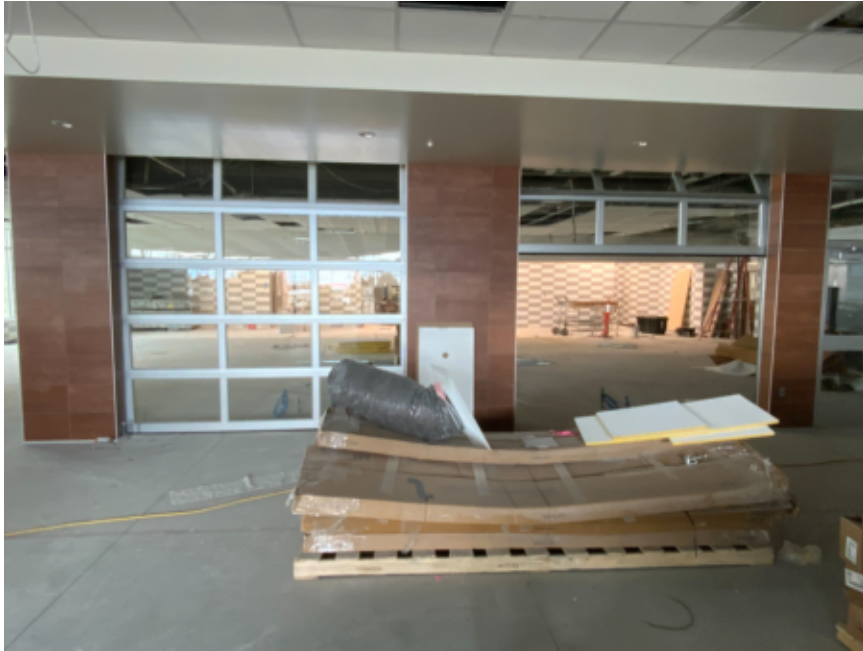
Roll-up doors in Serving Area
