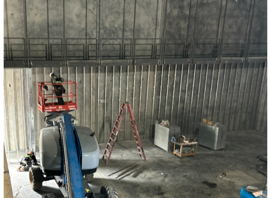
Metal stud installation progress
