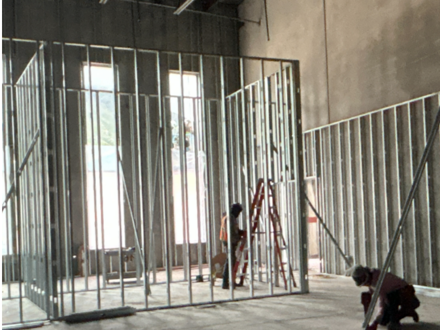
Metal stud installation progress
