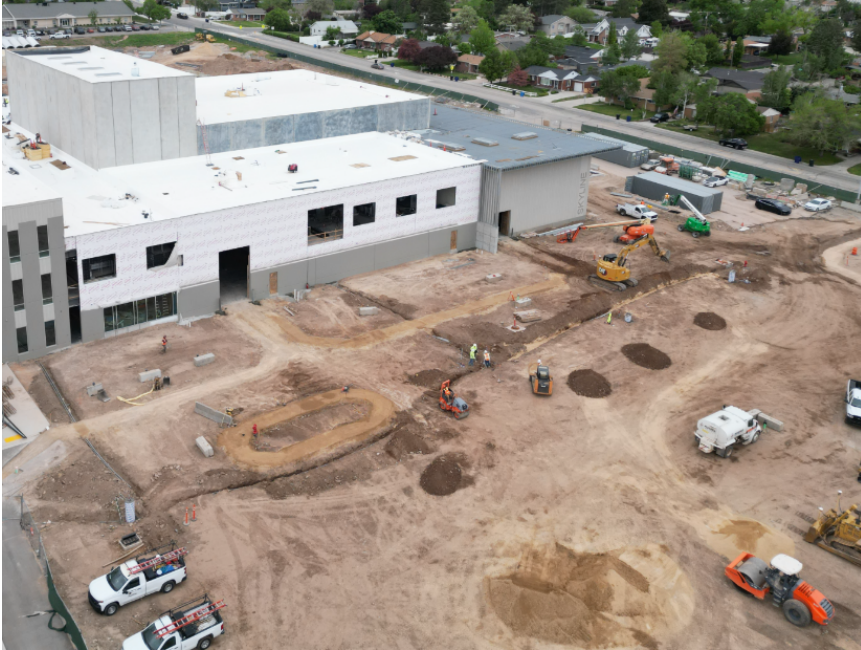
Site work progressing
