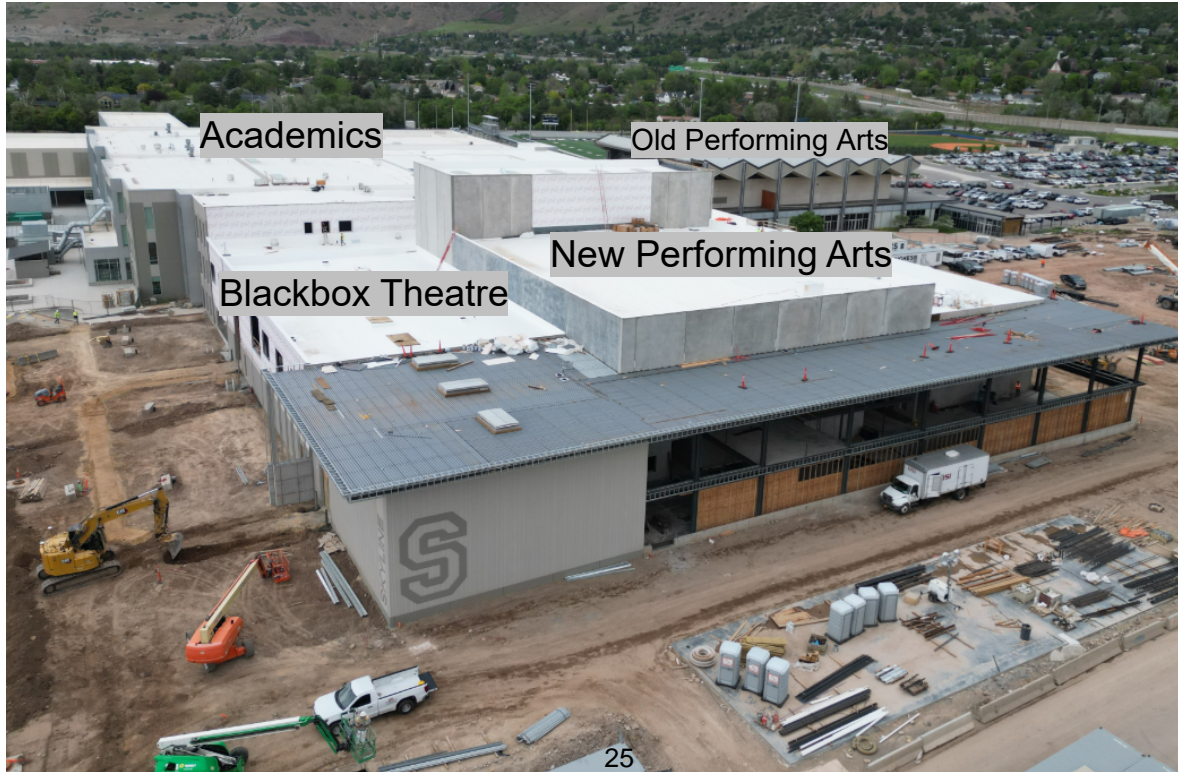
Performing Arts aerial photo May progress
