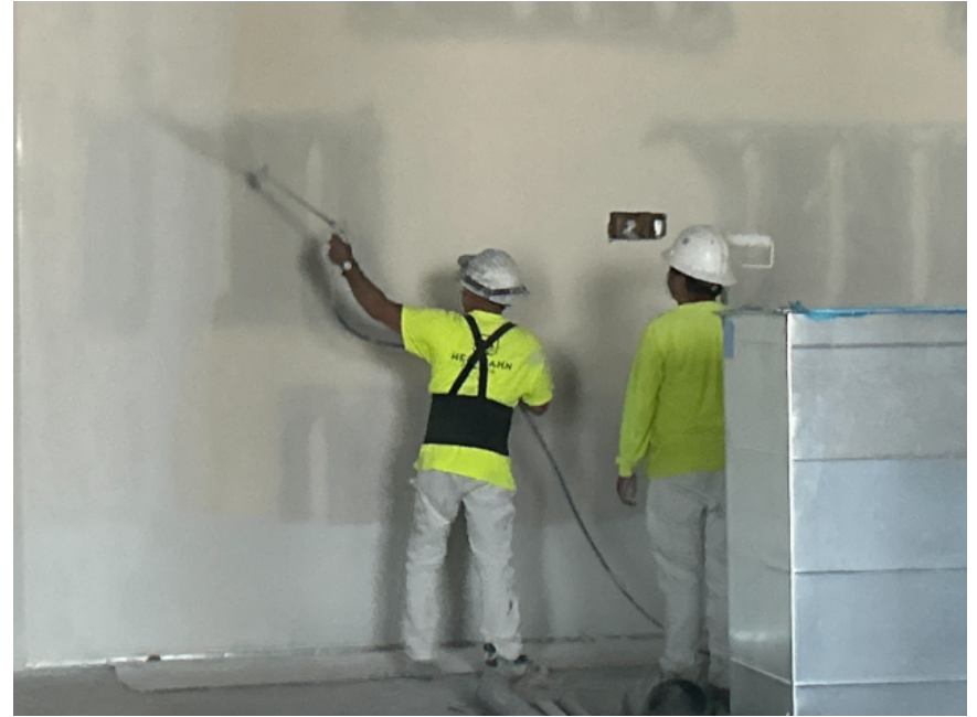
Prime coat install
