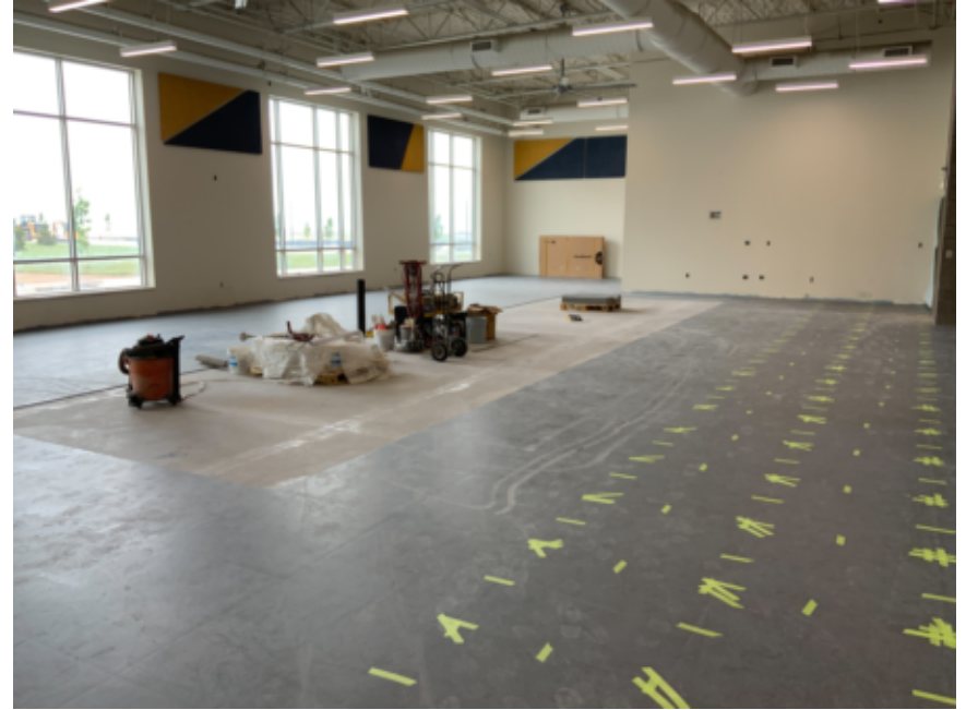
Weight Room flooring
