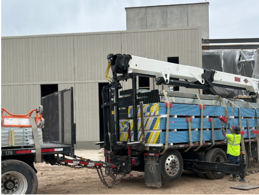
Drywall delivery to project
