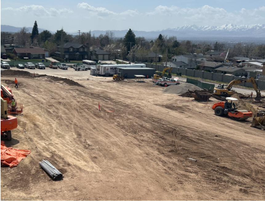
Site cleaned up
