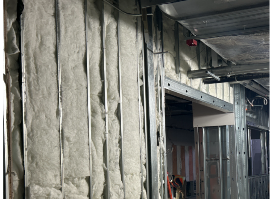
Batt insulation installed
