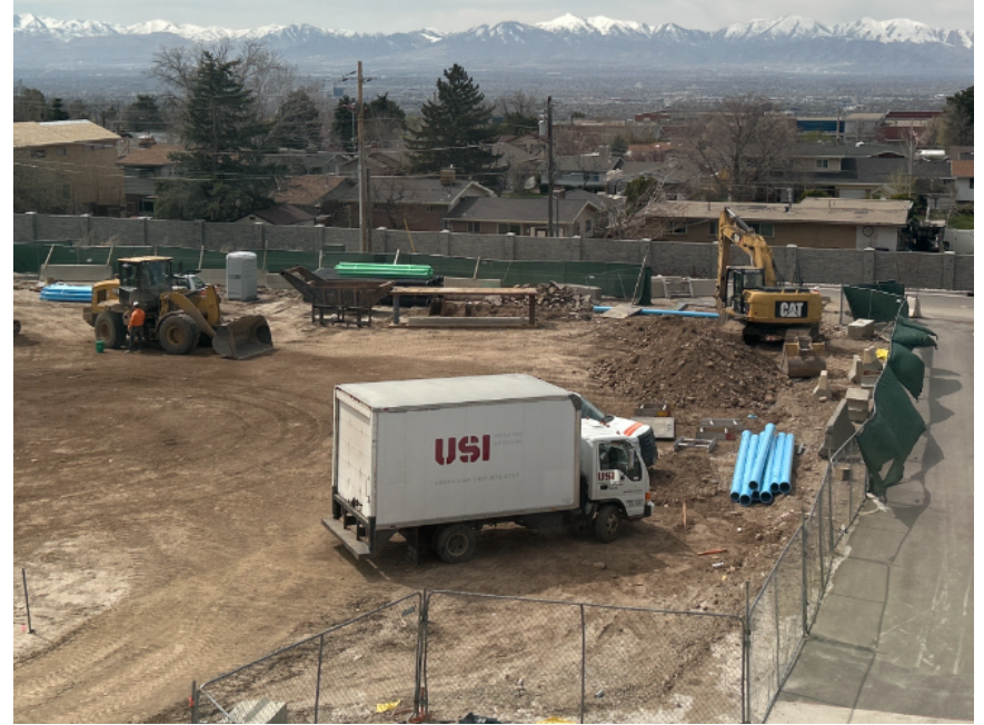
Excavation crews installing sewer and water laterals
