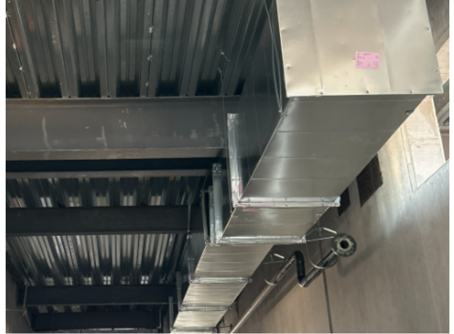
HVAC ductwork installed into place
