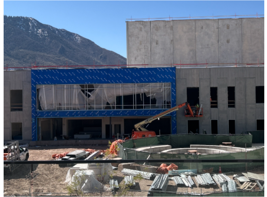
Window frame installation
