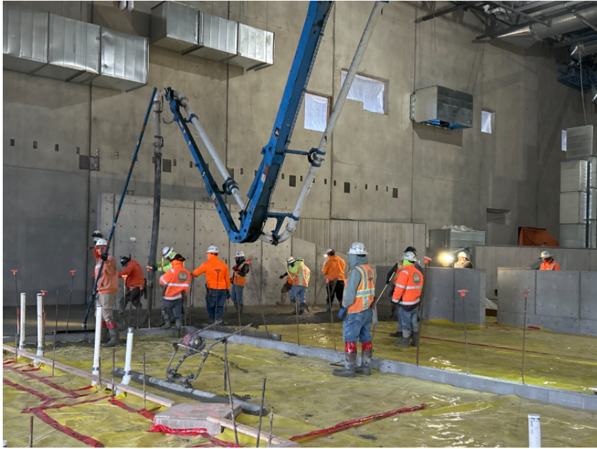
Pouring concrete in Auditorium
