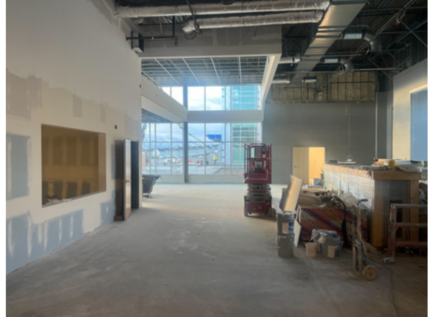
Athletics Field House drywall and ceiling grid
