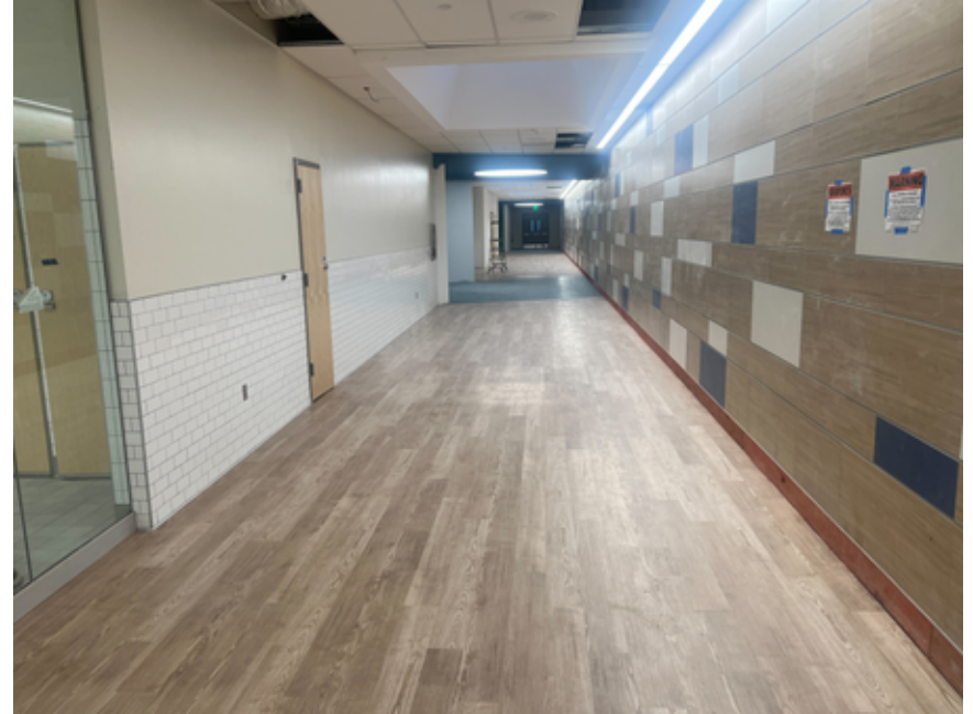
Corridor flooring Level 4 Social Studies
