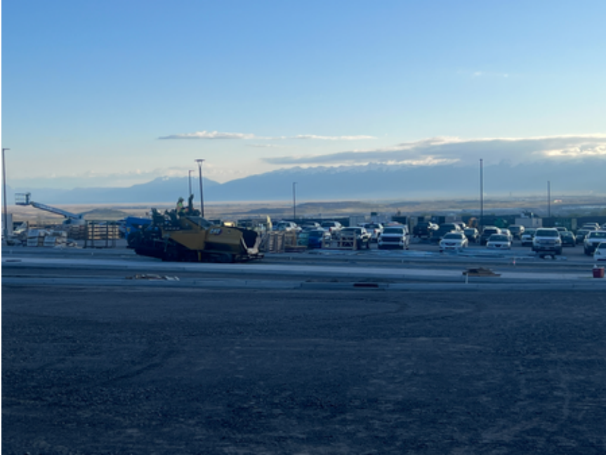
Asphalt has arrived onsite
