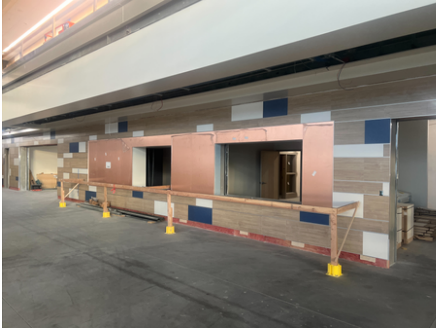
Wall paneling in the Main Entrance
