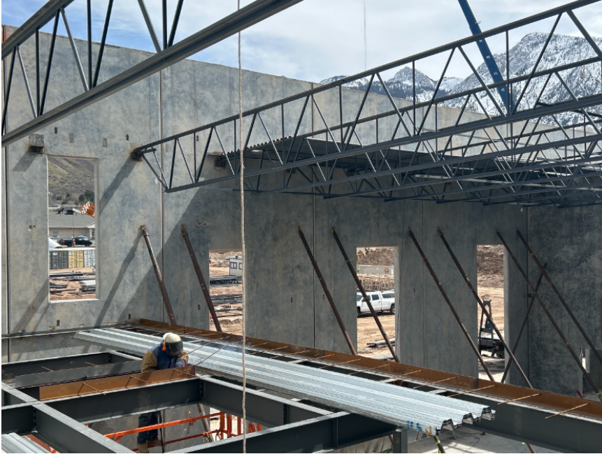
Trusses and B Decking installation
