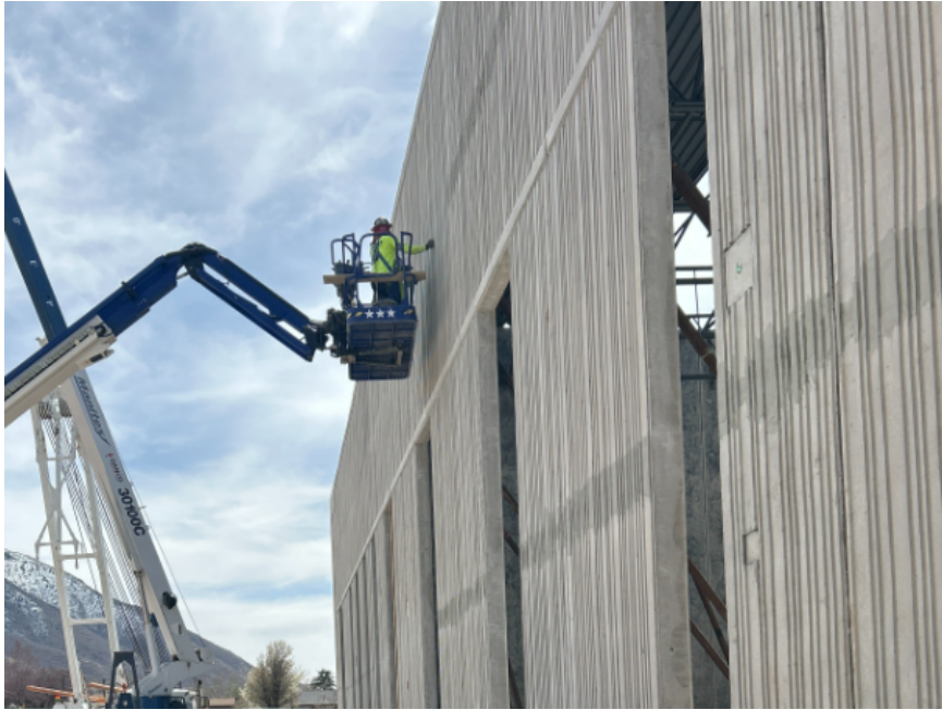
Exterior paint prep
