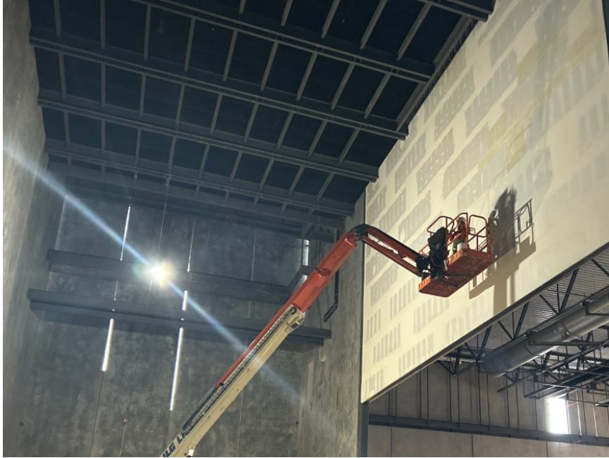
Auditorium proscenium wall fire tape progress
