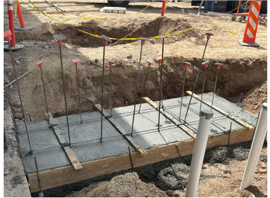
Concrete footing poured
