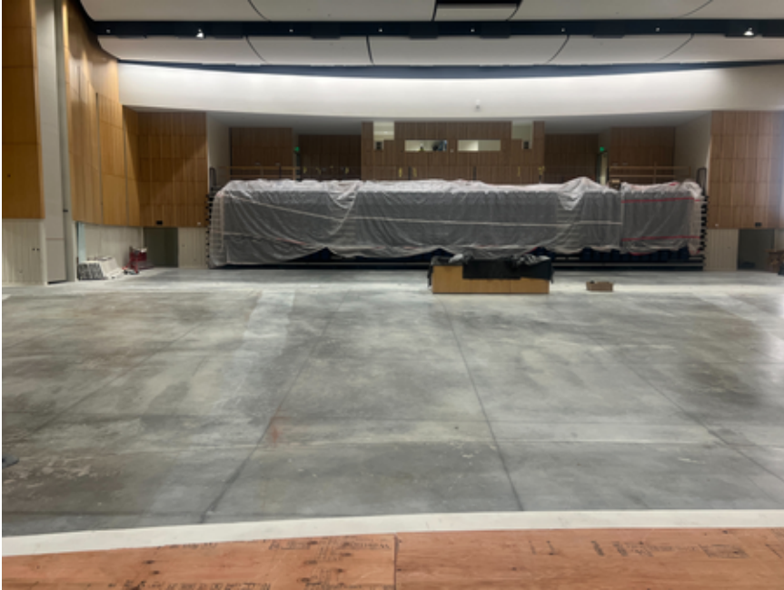
Sealed Concrete in the Auditorium
