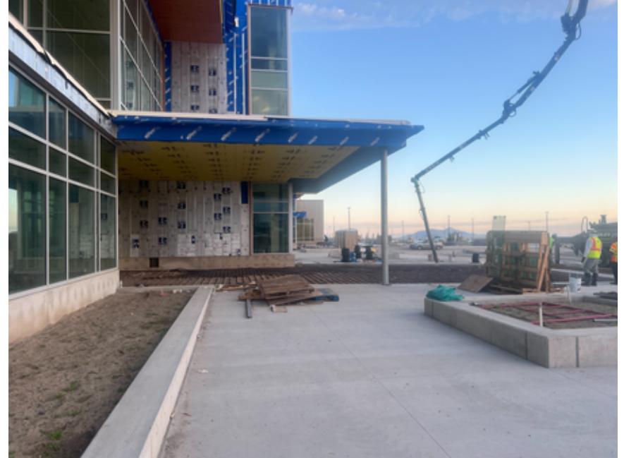
Concrete being poured on the snow melt system
