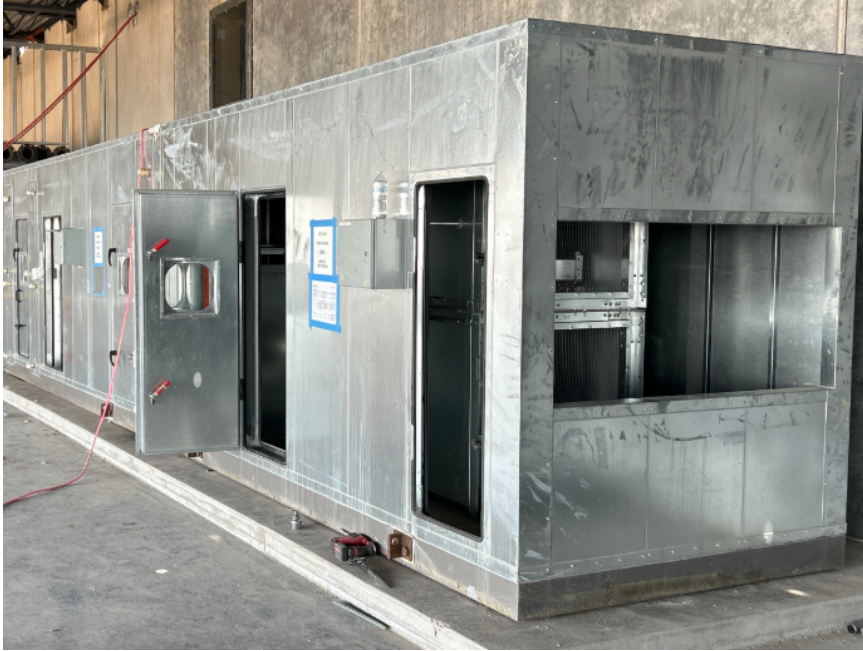
Air handler 14 lifted into place
