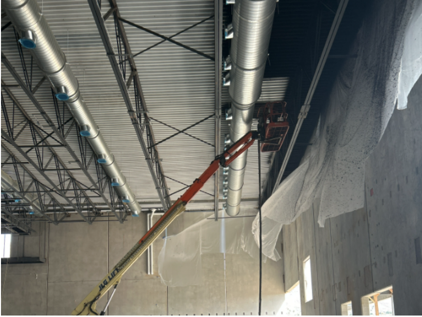
Insulation on the Auditorium ceiling installed
