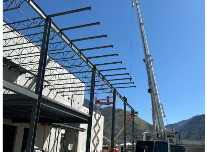
Trusses and B Decking installation
