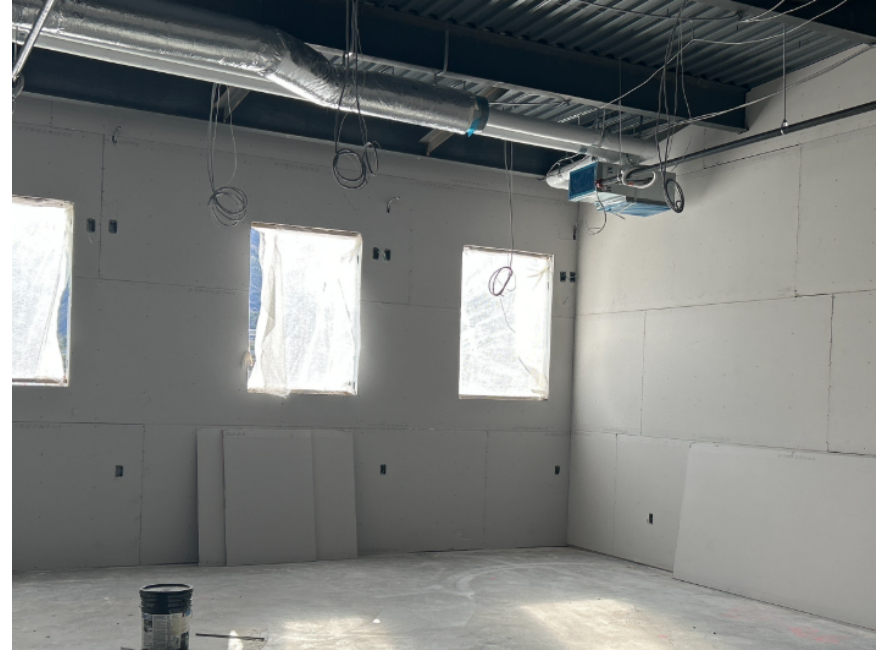
Drywall in Area H Level 4
