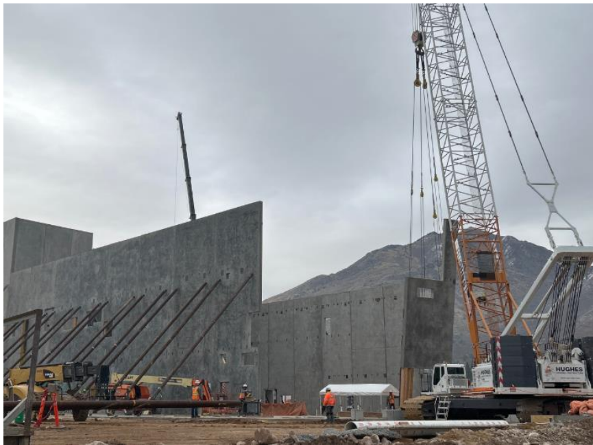
Tilt panel being placed west of the Auditorium
