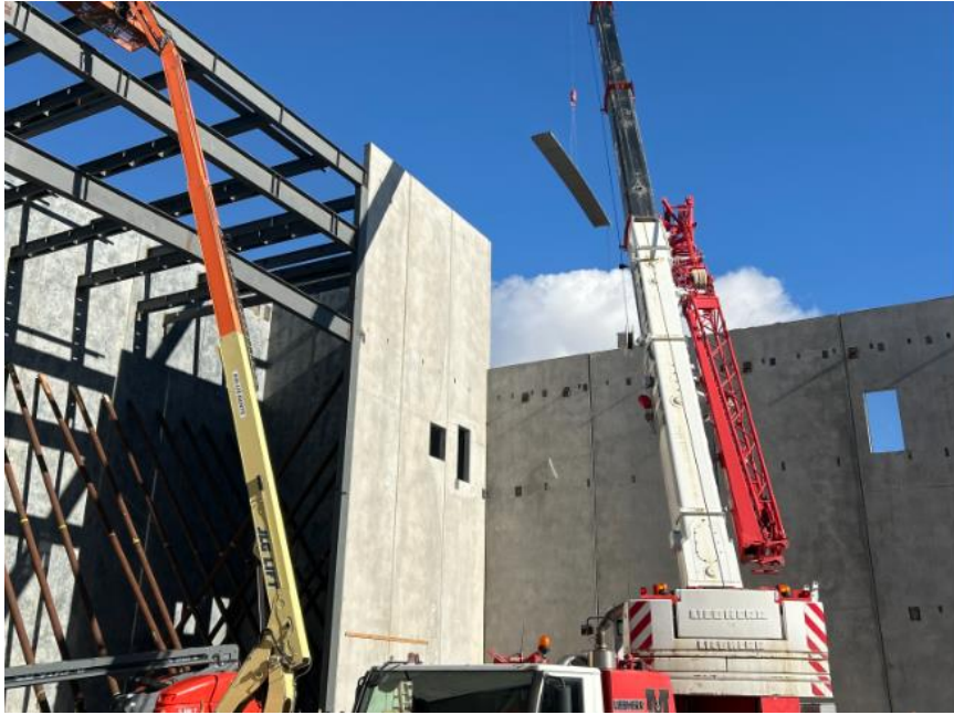
Steel beams and B decking being installed at Auditorium stage ceiling
