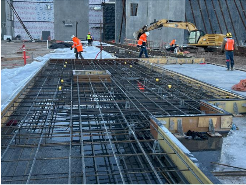
Installing rebar in tilt panels west of the Auditorium
