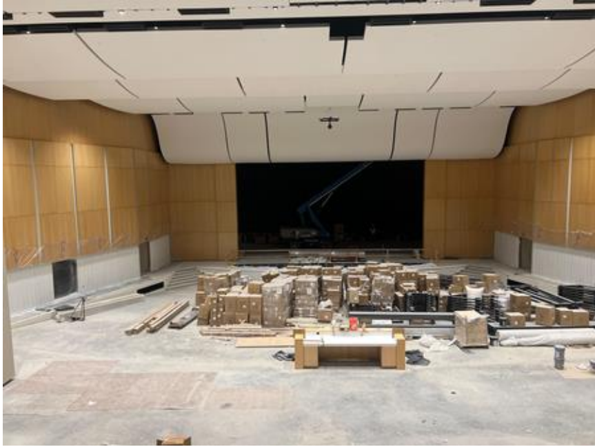
Wood paneling in the Auditorium
