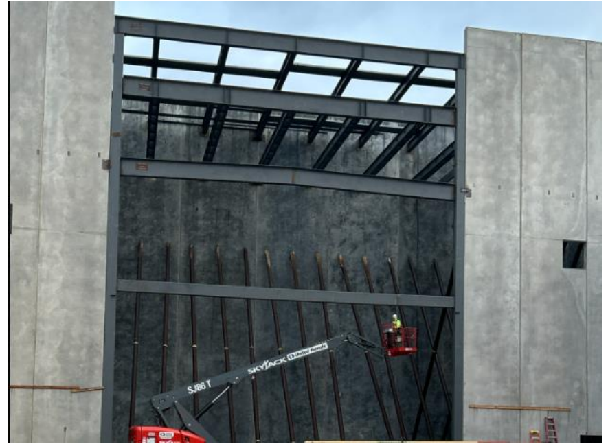
Steel beams and B decking being installed at Auditorium stage ceiling
