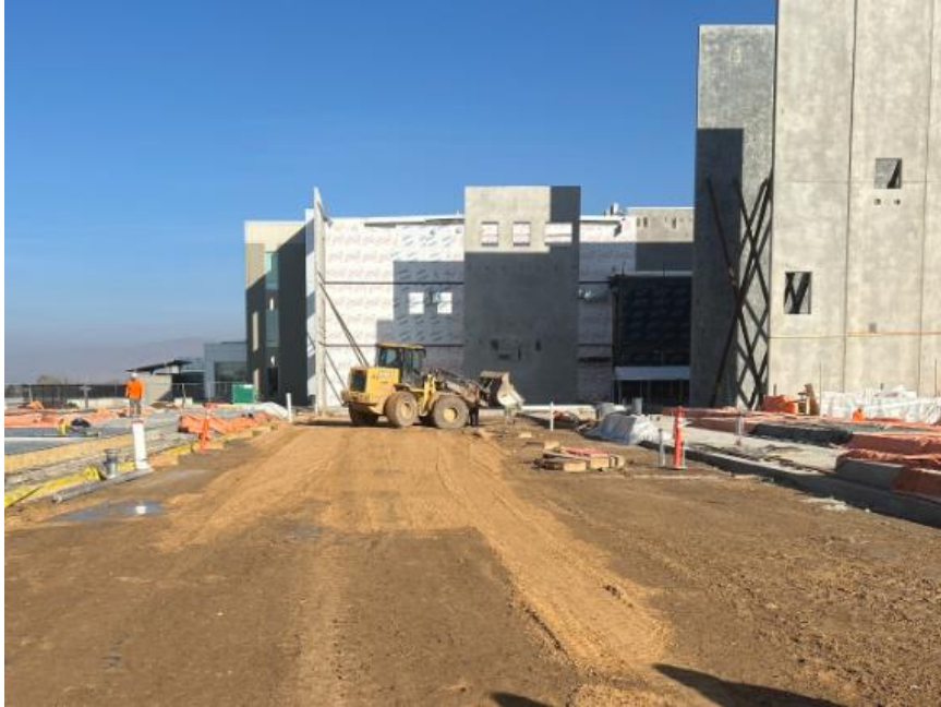
Sub concrete grade prep west of the Auditorium
