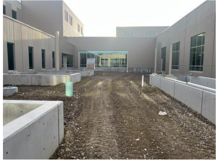
Sunshade footings in Administration Courtyard
