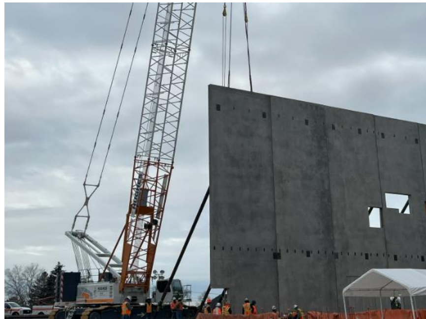
Tilt panel being placed west of the Auditorium
