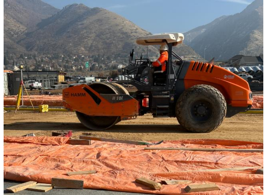
Sub concrete grade prep east of the Auditorium
