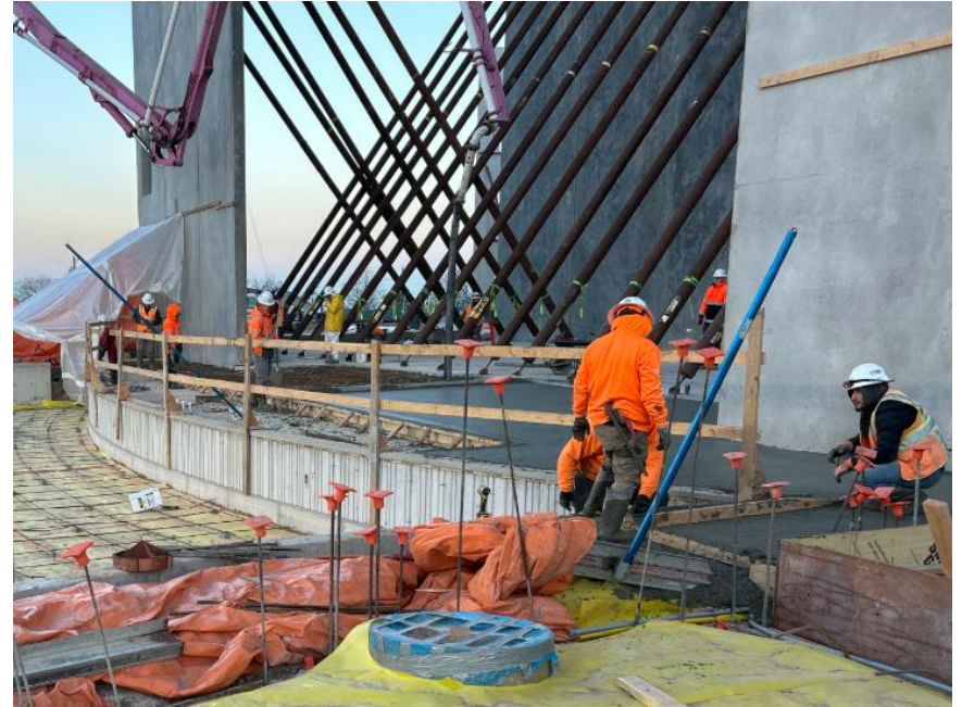
Crews pouring the suspended concrete slab at the Orchestra Pit
