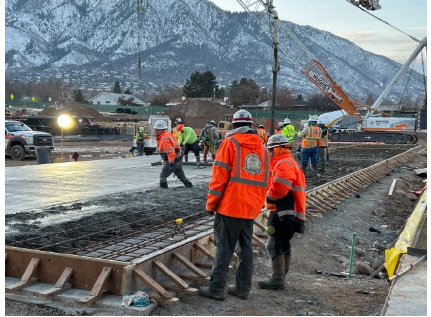
Pouring concrete east of the Auditorium
