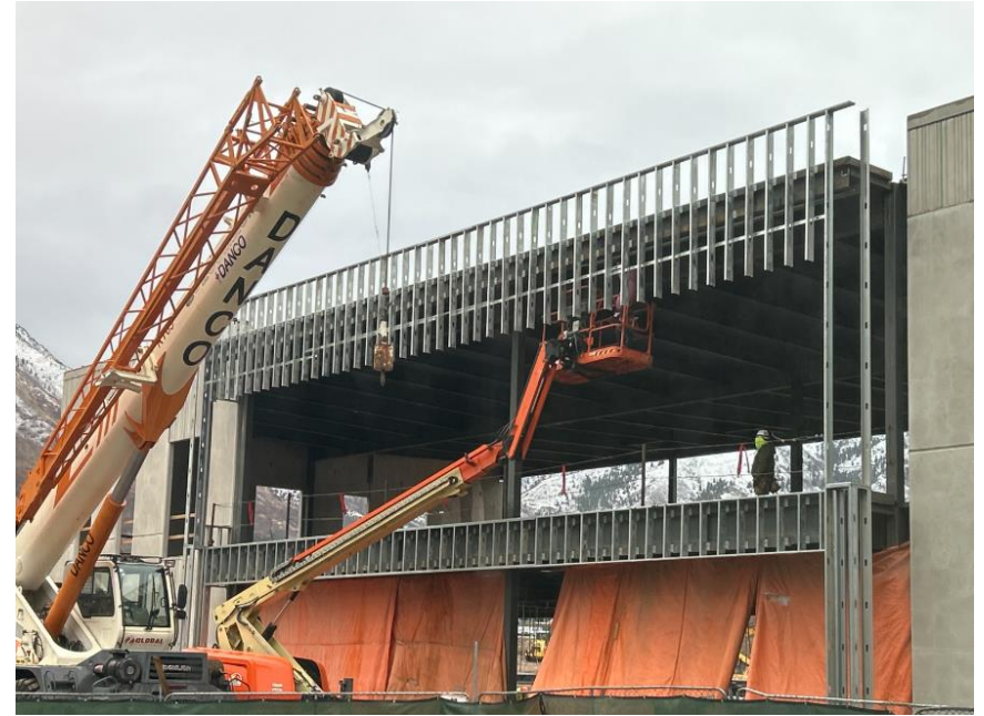
Structural steel placed and parapet wall framing north of the Auditorium
