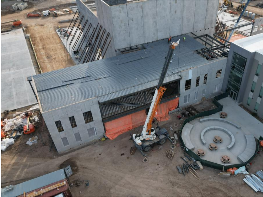
Structural steel placed and parapet wall framing north of the Auditorium
