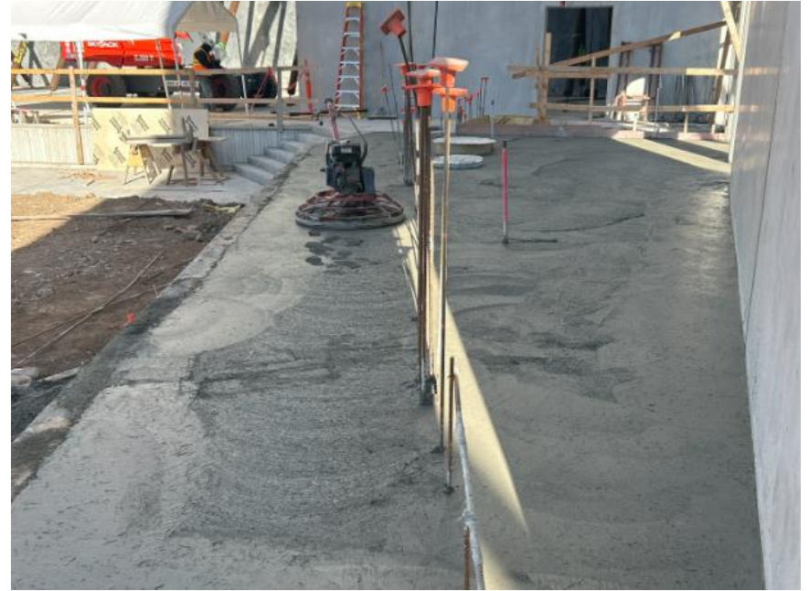
Concrete poured east of the Auditorium
