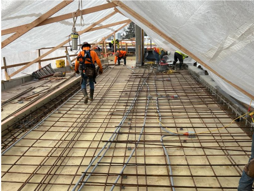
Crews prepping rebar and installing conduits for suspended concrete slab at the Orchestra Pit 31
