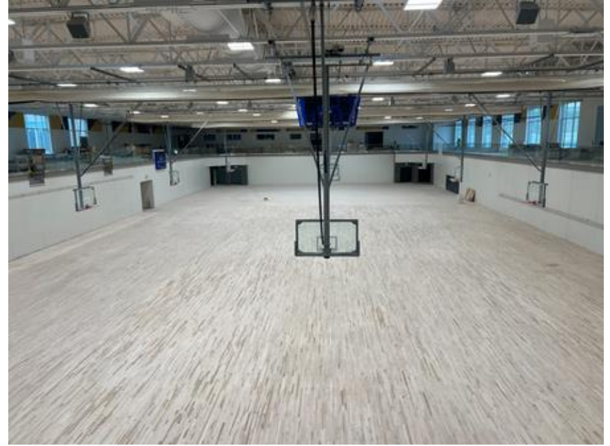
Basketball floor installation completed
