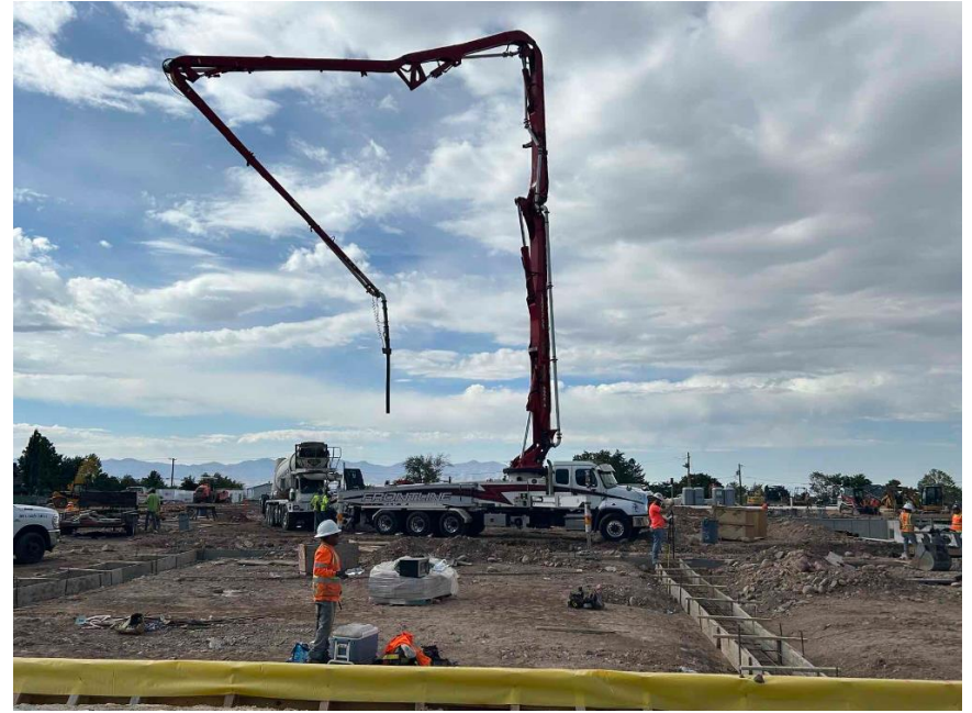
Pouring concrete footings East of the orchestra pit 27
