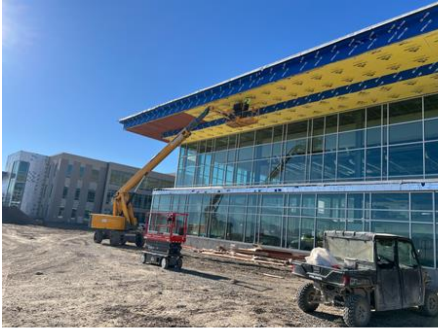
Metal panels on the exterior of Commons
