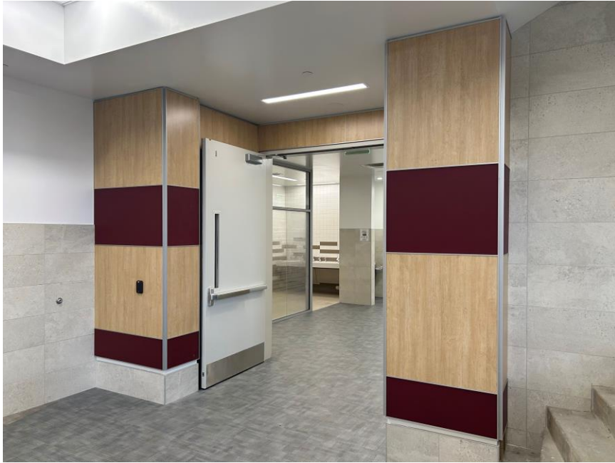
Wall finishes at entry to classroom pods
