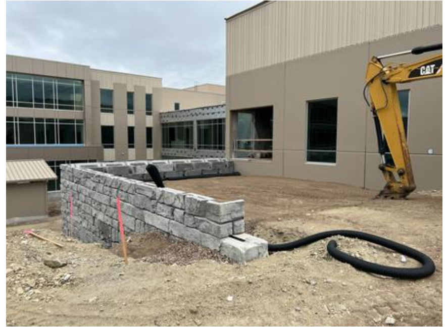
Retaining wall at CTE Entrance
