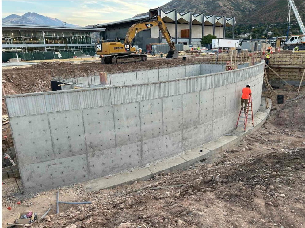
Orchestra pit foundation poured and preparing for backfill
