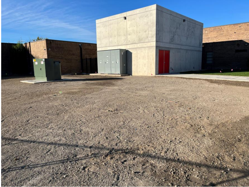
Central Plant exterior
