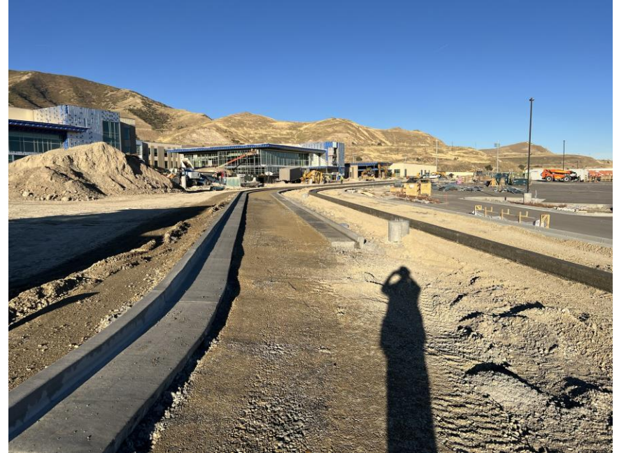
Curb and gutter to the South
