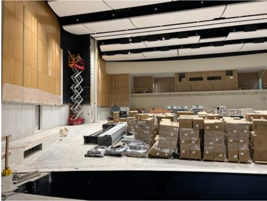
Wood paneling in the Auditorium
