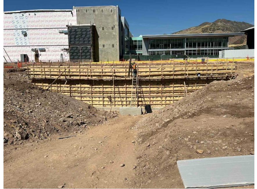
Preparing orchestra pit foundation for concrete
