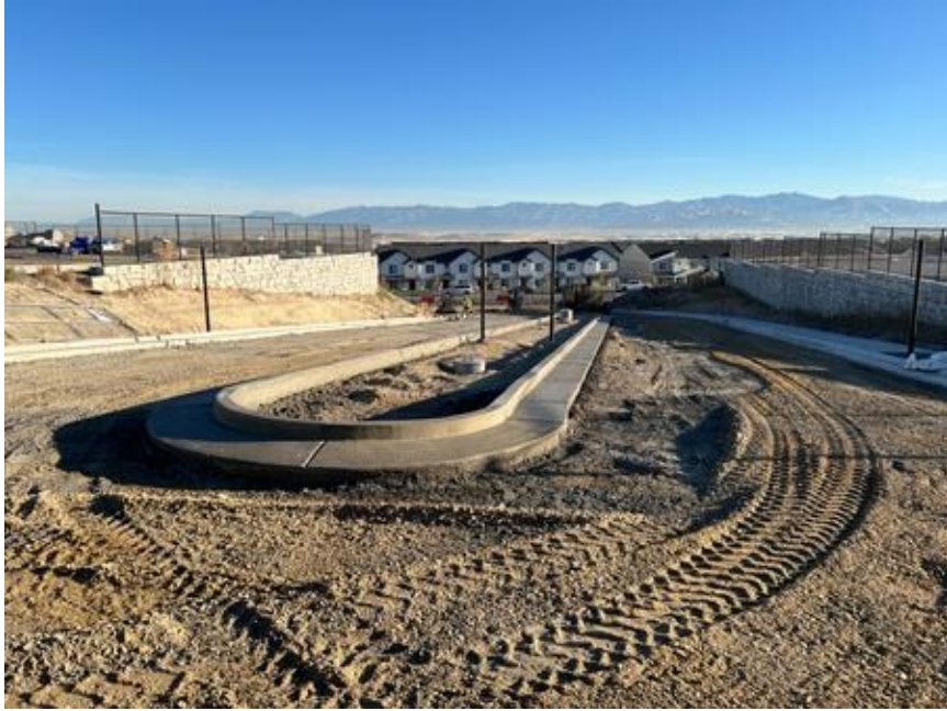
Curb and gutter at the East Entrance
