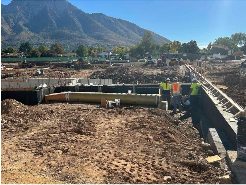
HVAC installation north of the orchestra pit
