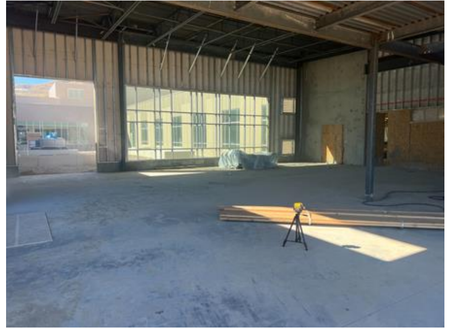
Cement floor in the Athletics Fieldhouse
