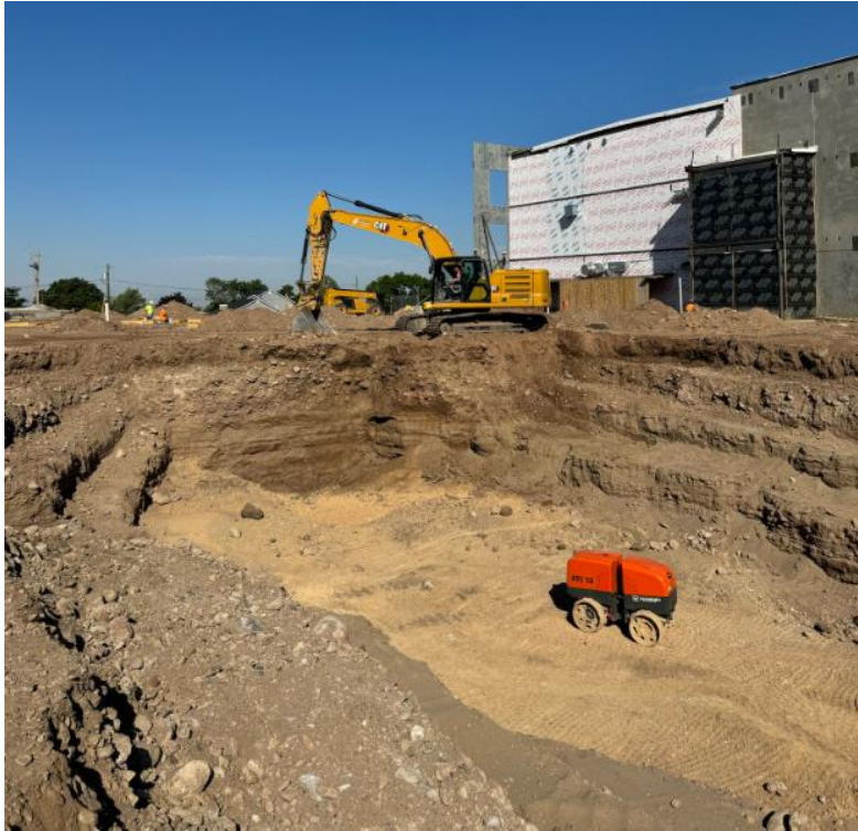
Orchestra pit being dug
