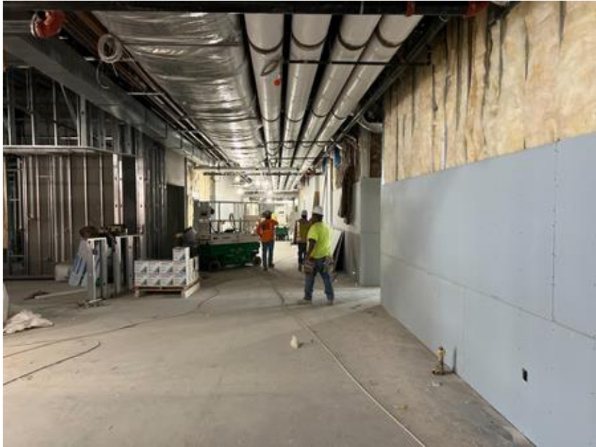
Insulation and drywall on Level 1 of Academics
