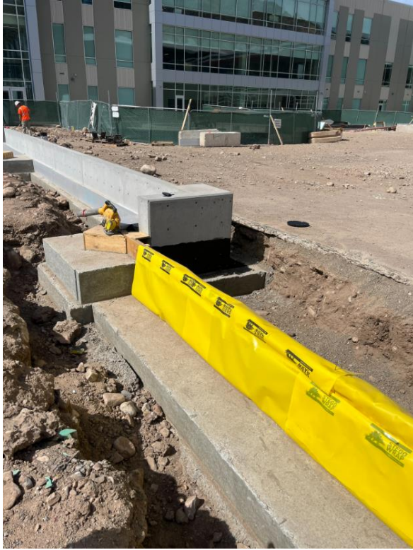
Waterproofing of foundation walls and moisture barrier on the north end
