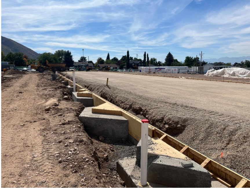
Footings poured along the west side
