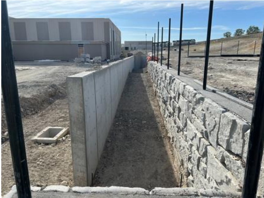
Ramp leading to the Lacrosse Field
