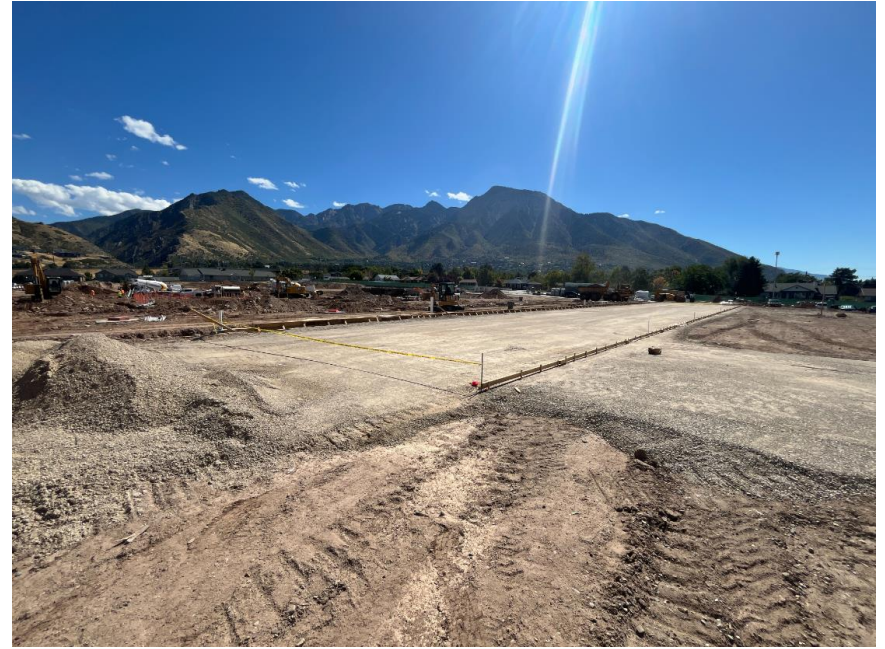
Tilt panel waste slab prepped and ready to be poured
