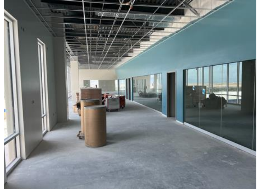
Glass installation at the classroom pods
