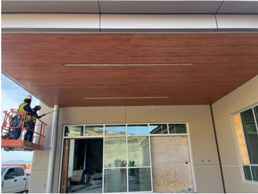
Soffit panels over the Pool entrance
