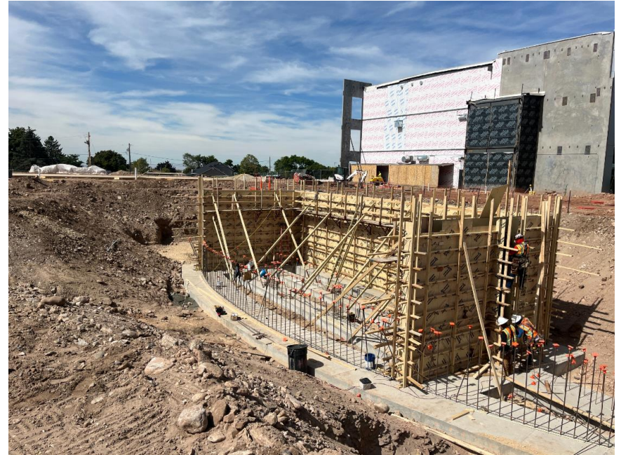
Orchestra pit with foundation walls poured
