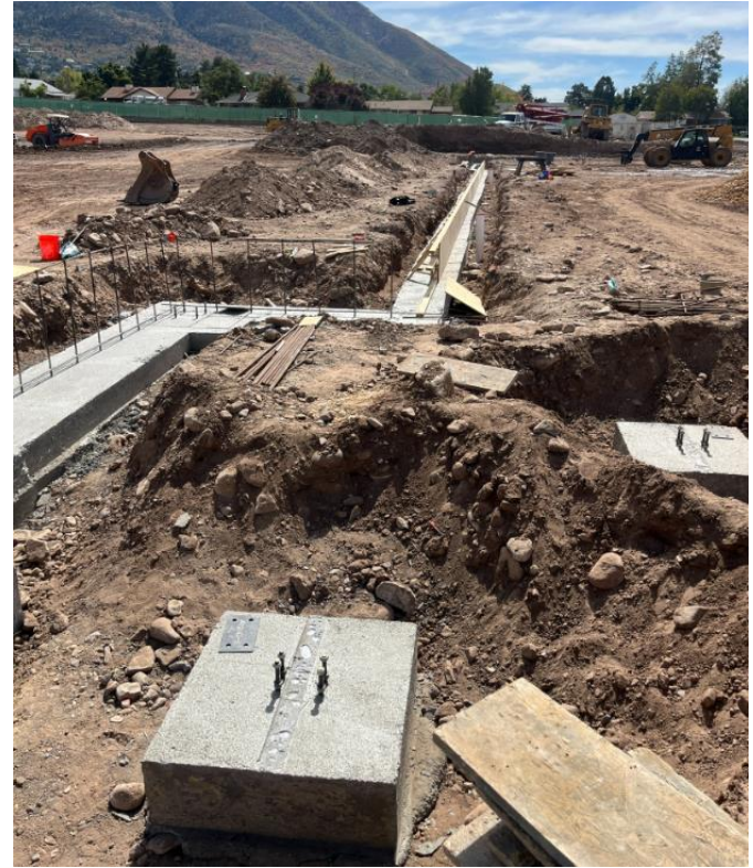
Footings poured along the east side of Performing Arts
