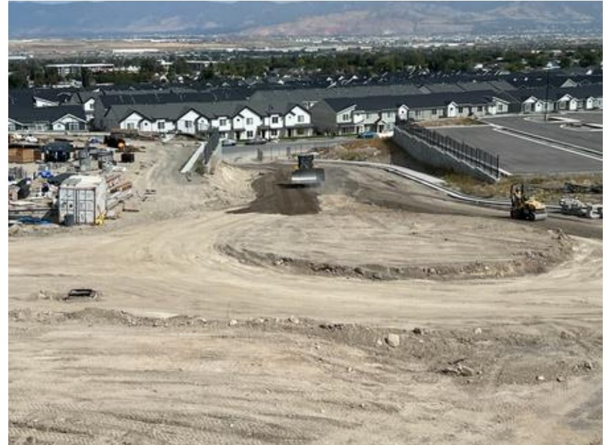
Grading the Main Drive
