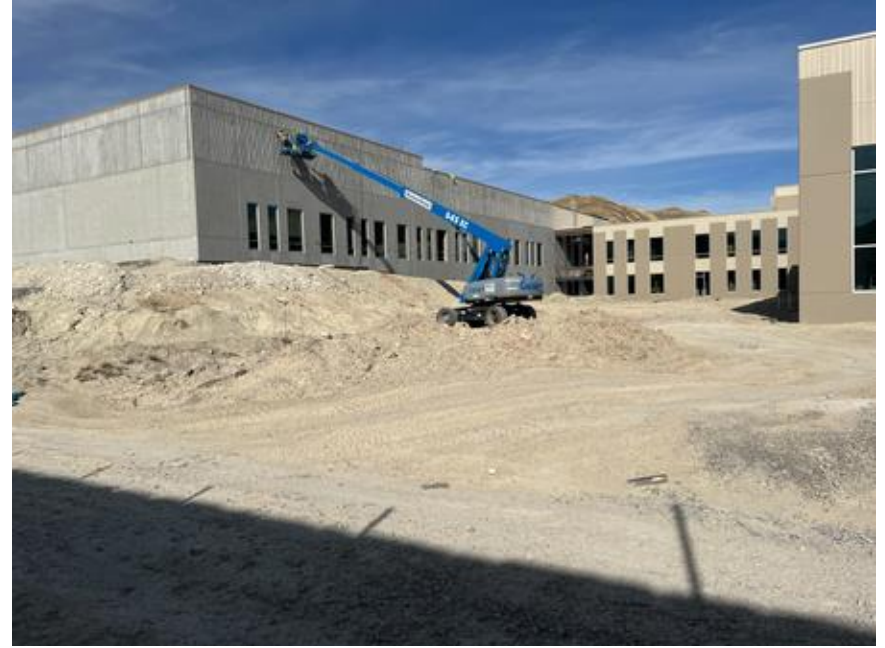
Glass installation on the exterior of CTE
