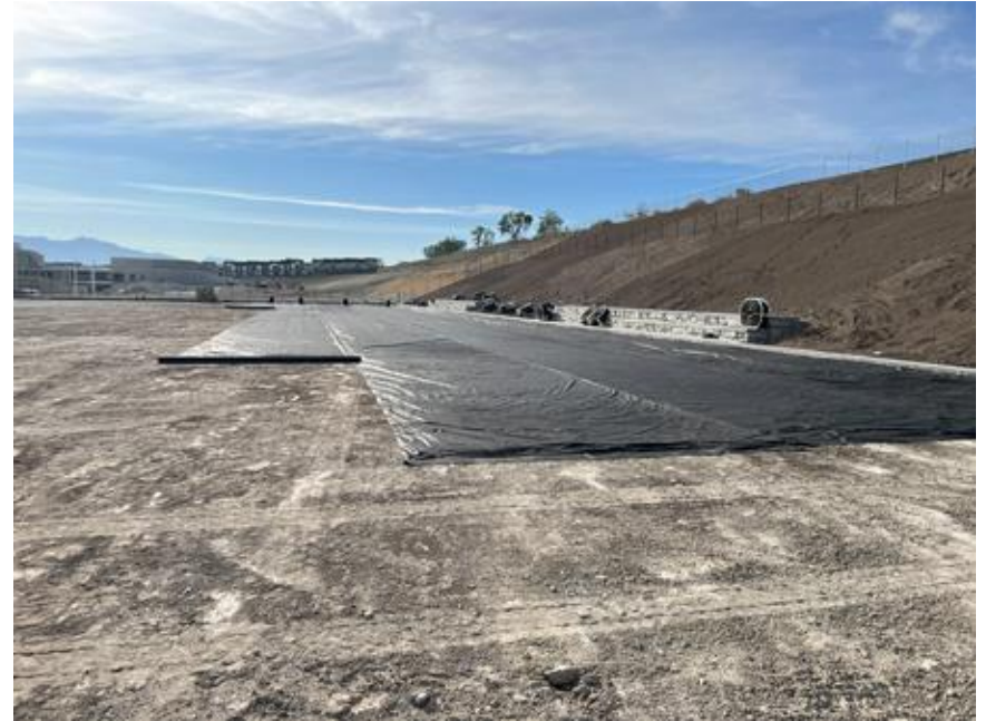
Geo-grid at the Lacrosse Field
