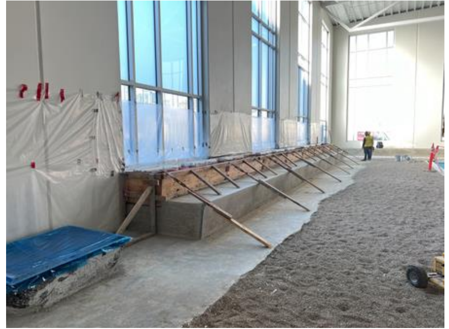
Cast in place benches at the Pool
