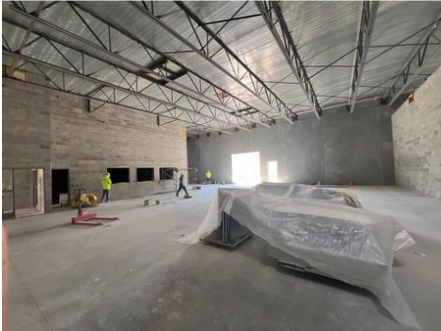
Roof decking in the Metal Shop
