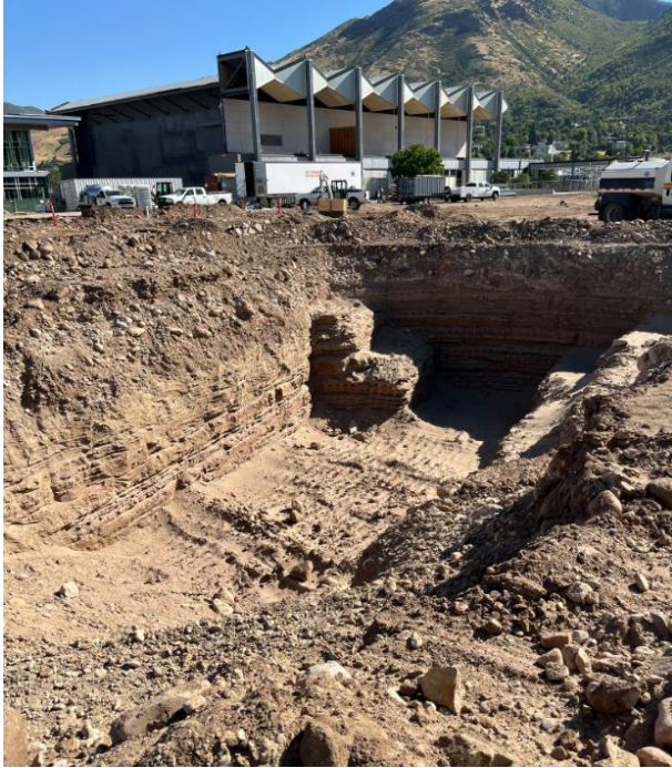
Orchestra Pit excavation
