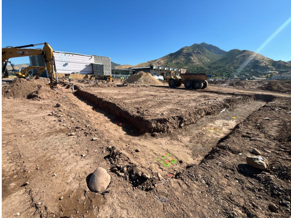
Footings being dug southwest of Performing Arts
