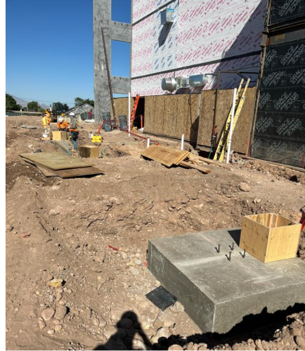
Spot footings being poured north of Performing Arts
