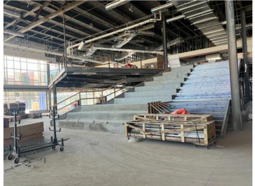
Learning Stairs poured in place
