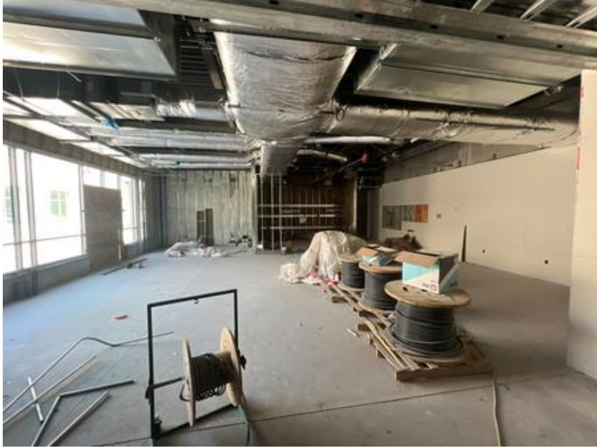
Drywall in the Faculty Lounge
