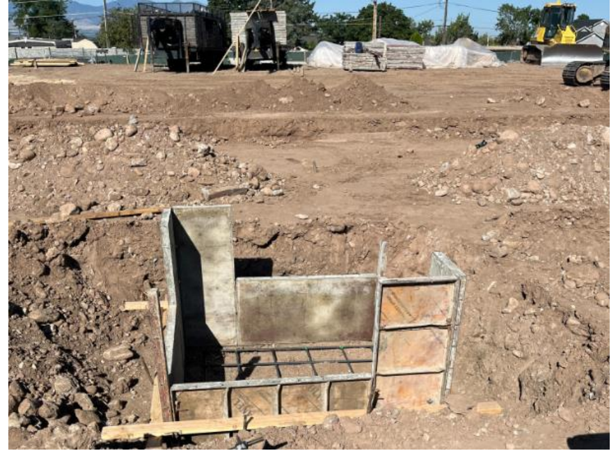
Spot footings being formed west of Performing Arts
