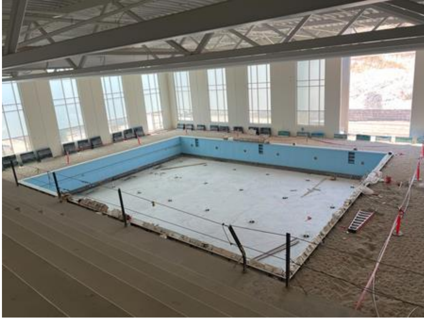
Slab on grade at the bottom of the Pool
