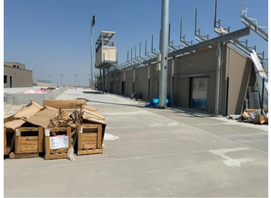
Roll up doors on home side bleacher storage
