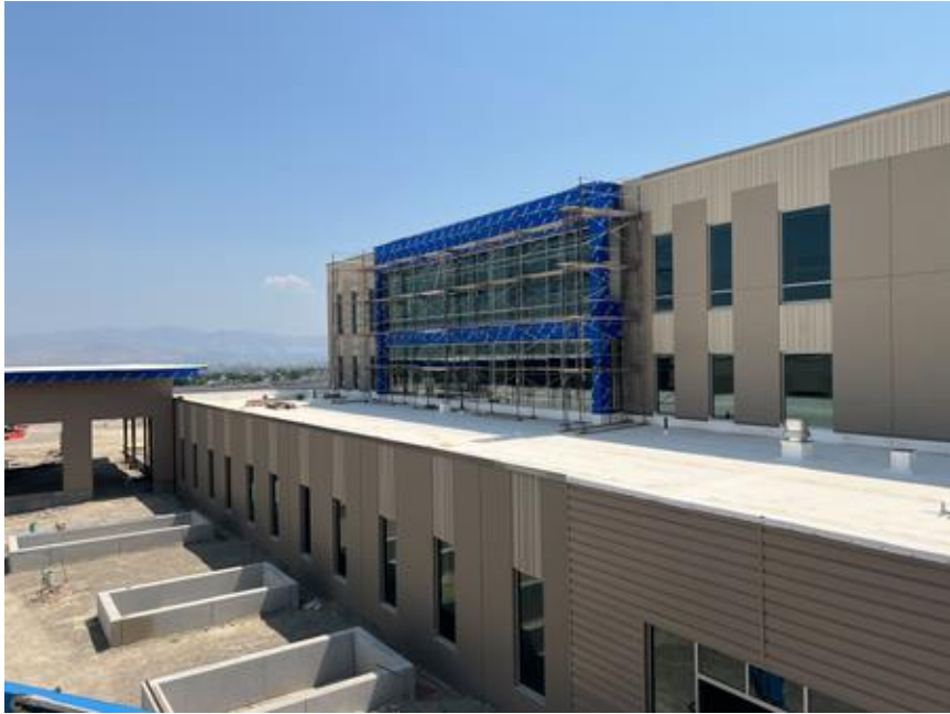
Metal panels on levels 2 and 3 of Administration
