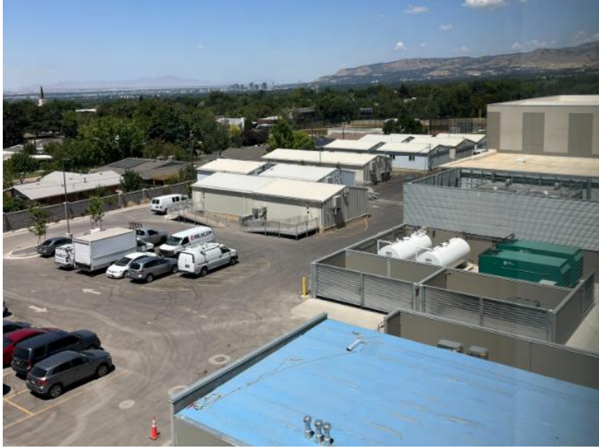
Relocatables set in west parking lot
