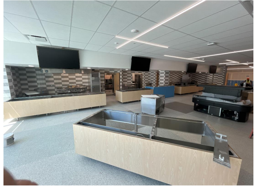
Serving line equipment being set
