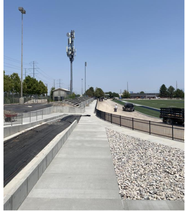
Concrete flatwork is complete
