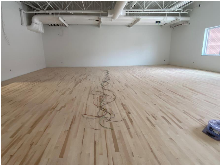
Hardwood floor in Dance Room installed
