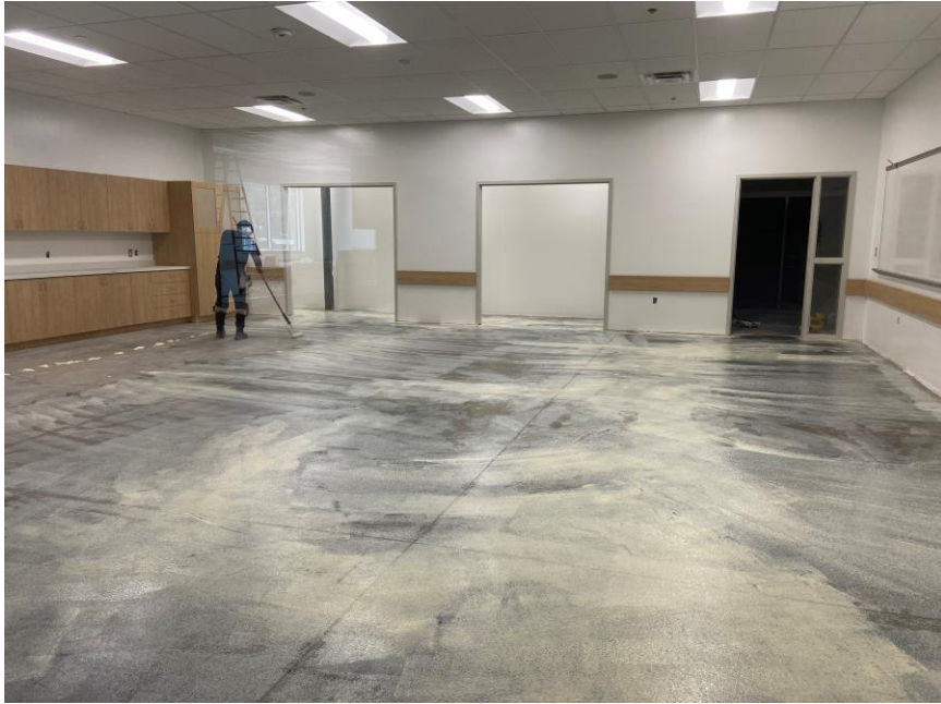
Floor slab preparation for tile in Tech Lab
