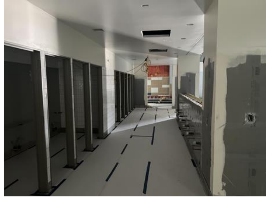
Tile in group restrooms
