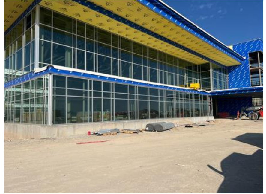
Curtain wall frame around the Commons
