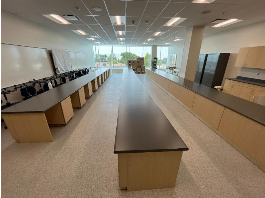
Sewing lab classroom nearing completion
