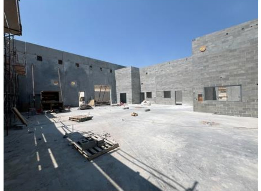
Masonry walls in the Manufacturing Shop
