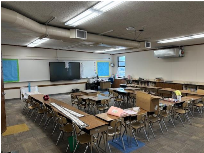
South wing classroom ready for students
