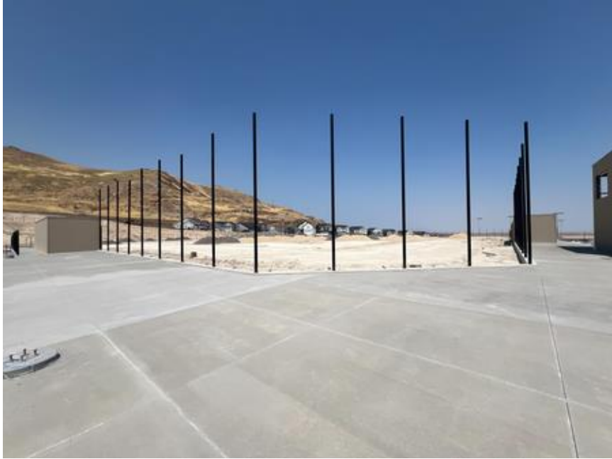
Baseball Field grading, infill, and fencing
