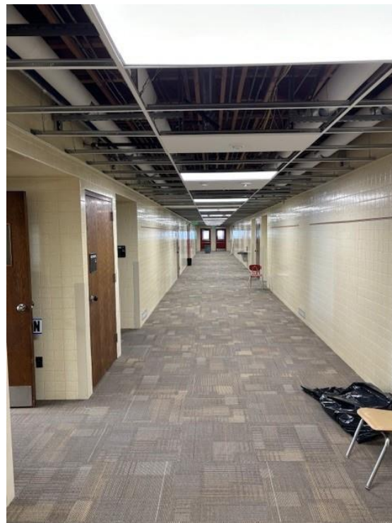
South wing corridor progress
