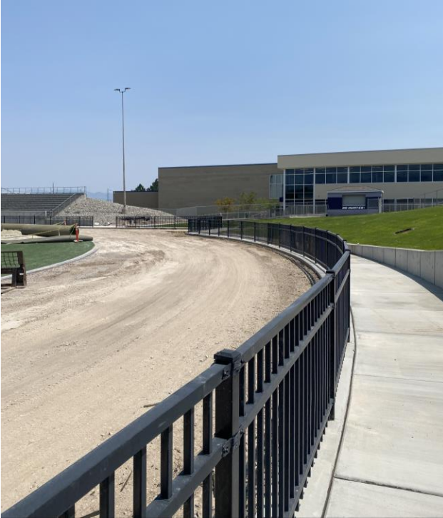
Fencing around Track is installed
