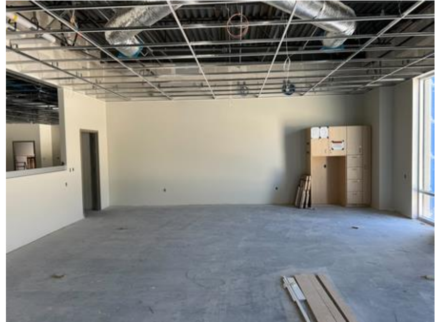
Casework, ceiling grid, and paint in Academics
