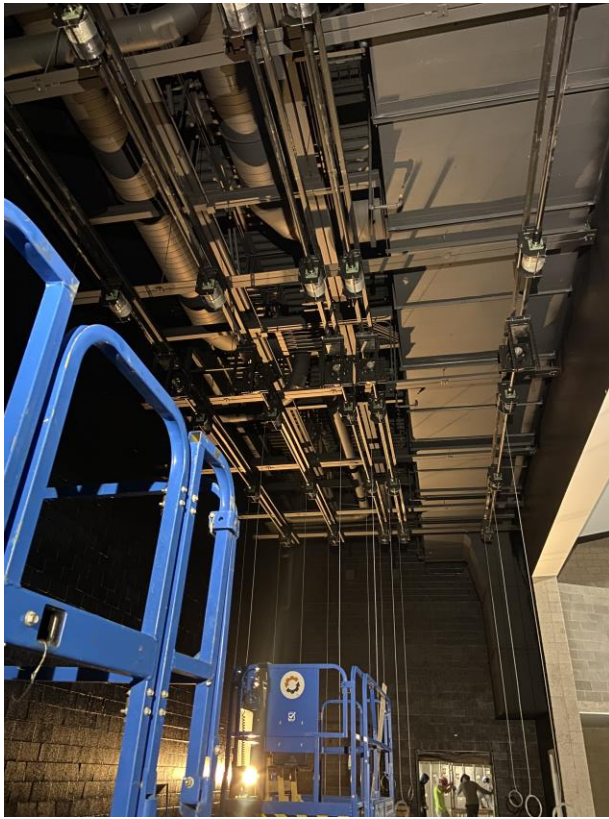
Stage rigging installation in progress
