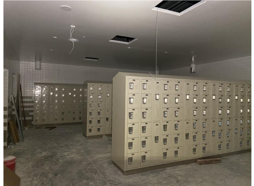
Lockers installed in Athletic locker rooms
