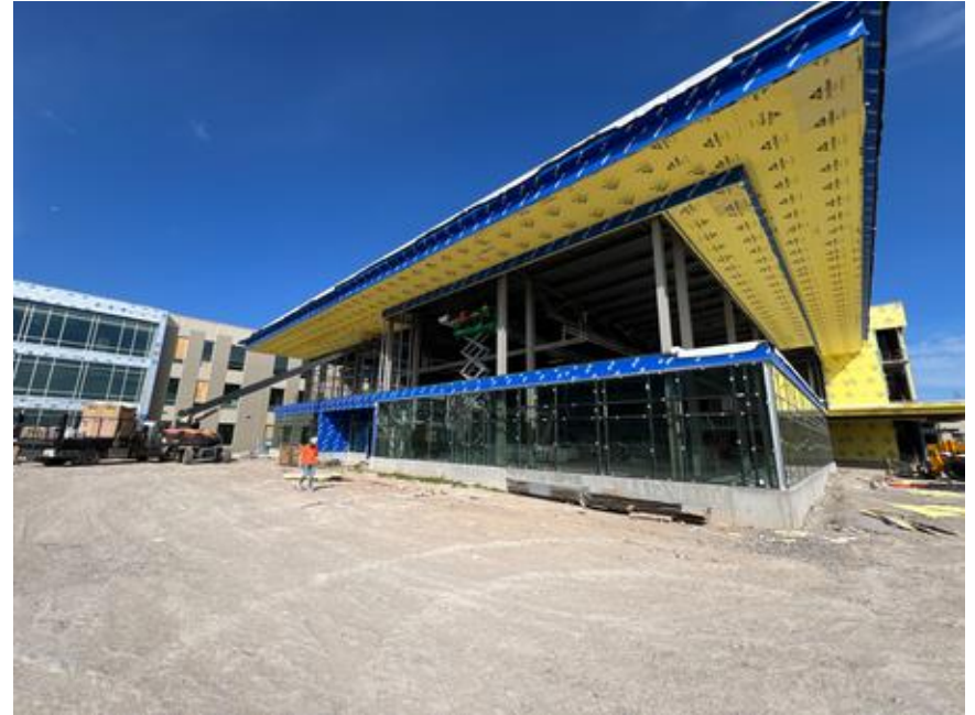
Glass glazing and frames outside Commons Area
