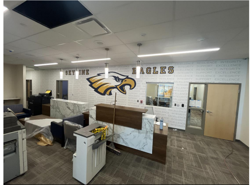
Furniture installation in Administration
