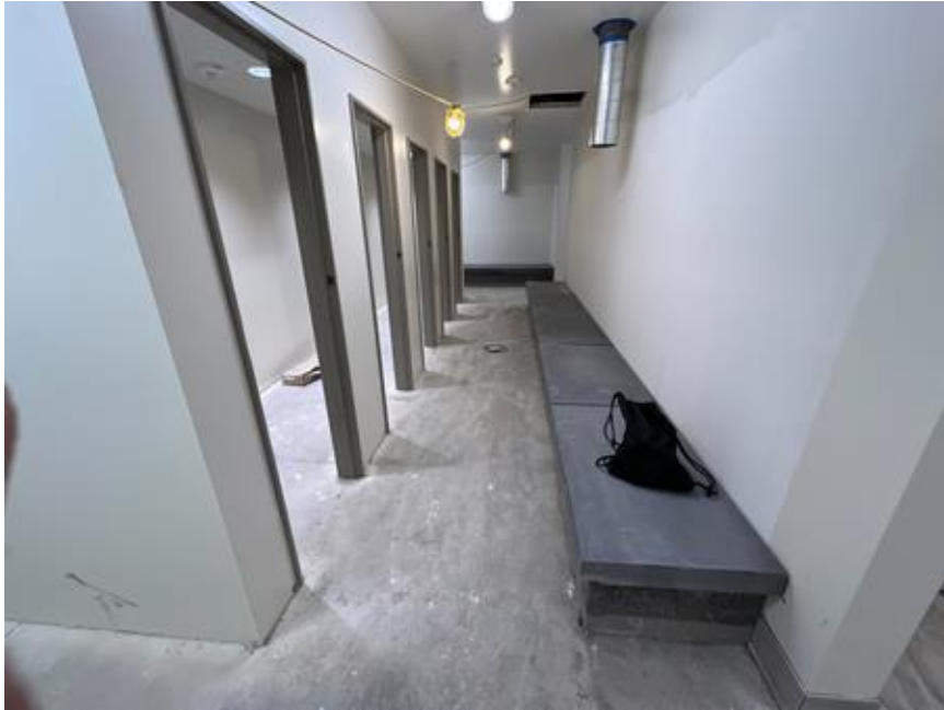
Pre-cast benches in team locker rooms
