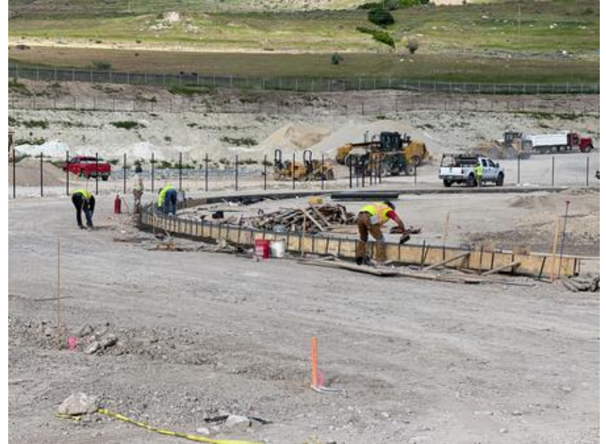
Stadium field drainage and curbing
