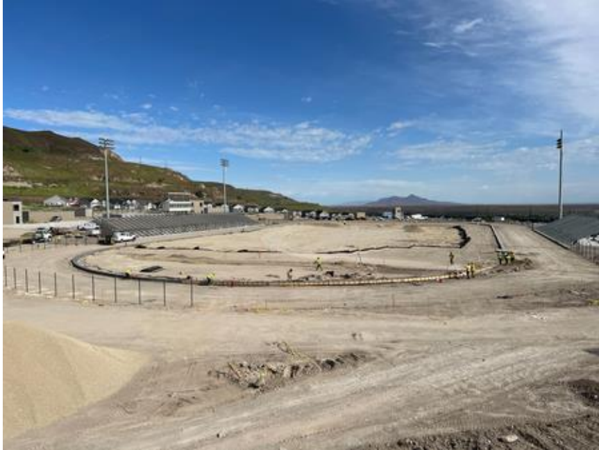
Stadium field base and perimeter fencing
