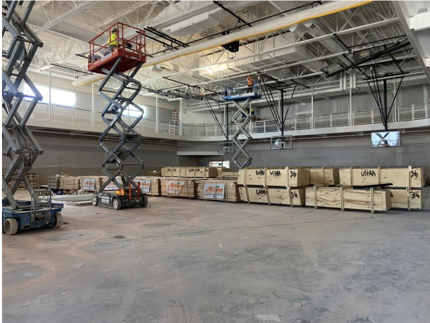
Gym flooring acclimatizing prior to installation
