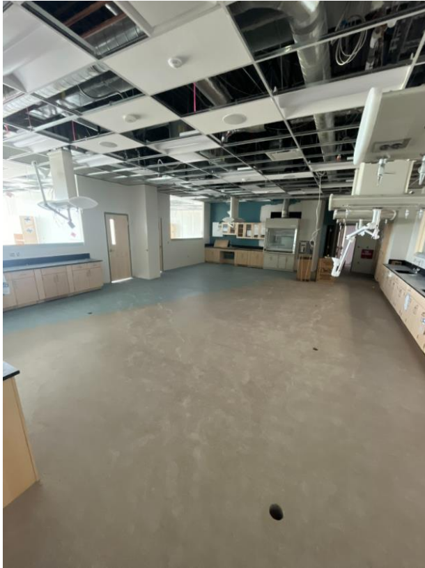
Science classroom with rubber flooring installed
