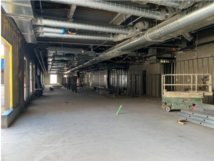
Framing in Administration
