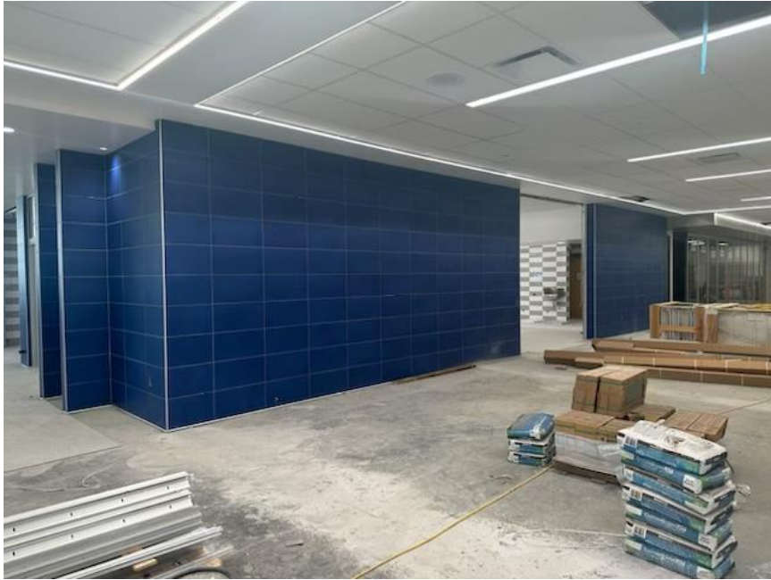
Large format tile installation in Serving Area
