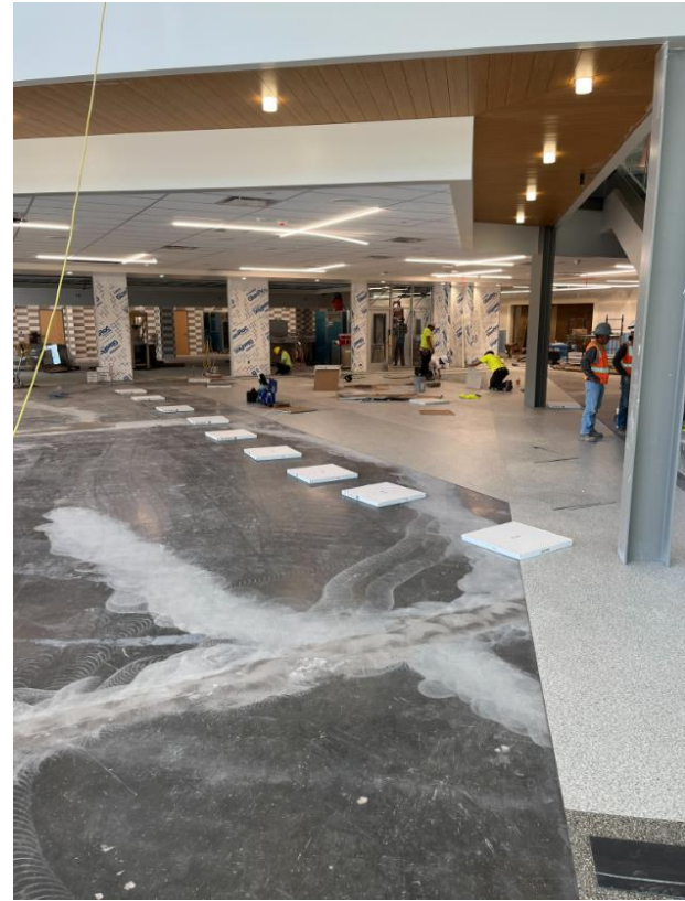
LVT flooring installation in the Commons Area
