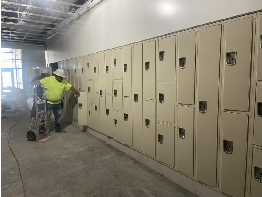
Lockers installed in hallways
