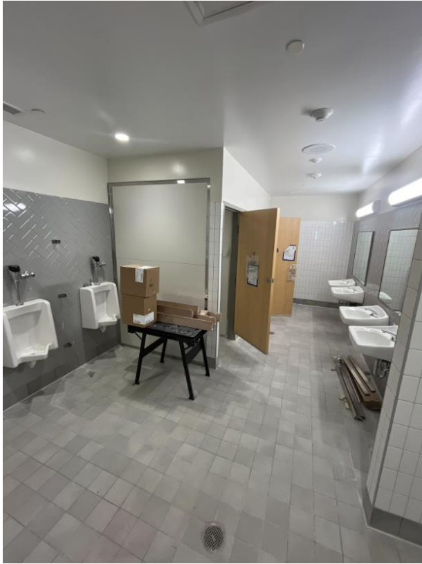
Men's restroom on Level 2
