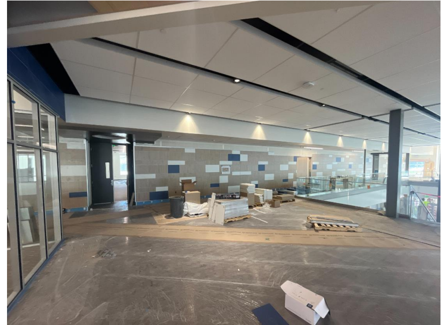
Wood accent wall installation in Level 2 Commons Space
