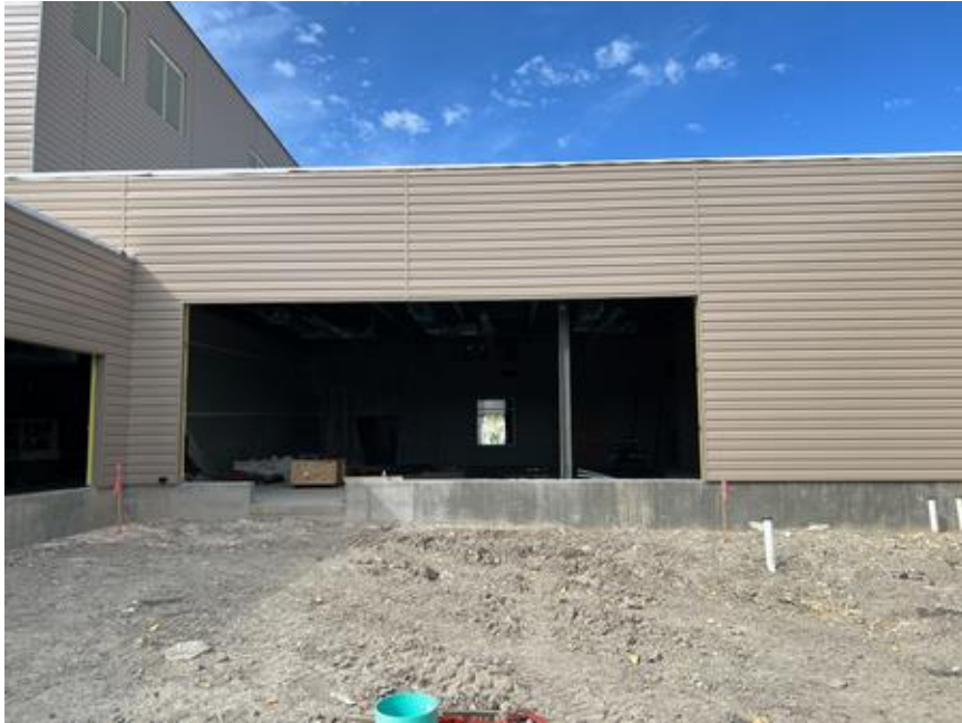
Testing Center siding
