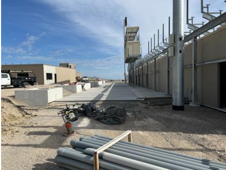
Flatwork behind the home team bleachers
