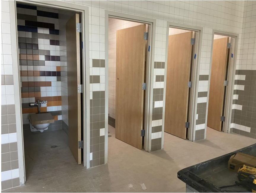
Restroom doors being installed
