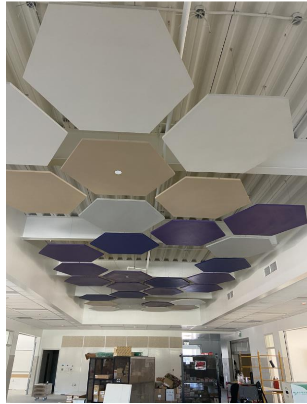
Collaboration space ceiling treatment installed
