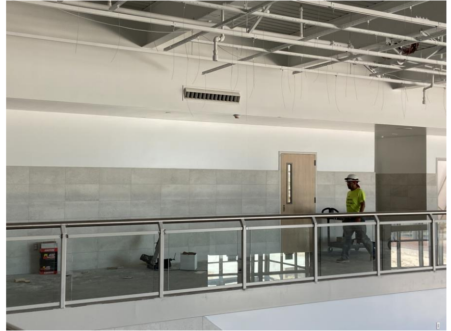
Balcony guardrail glass being installed
