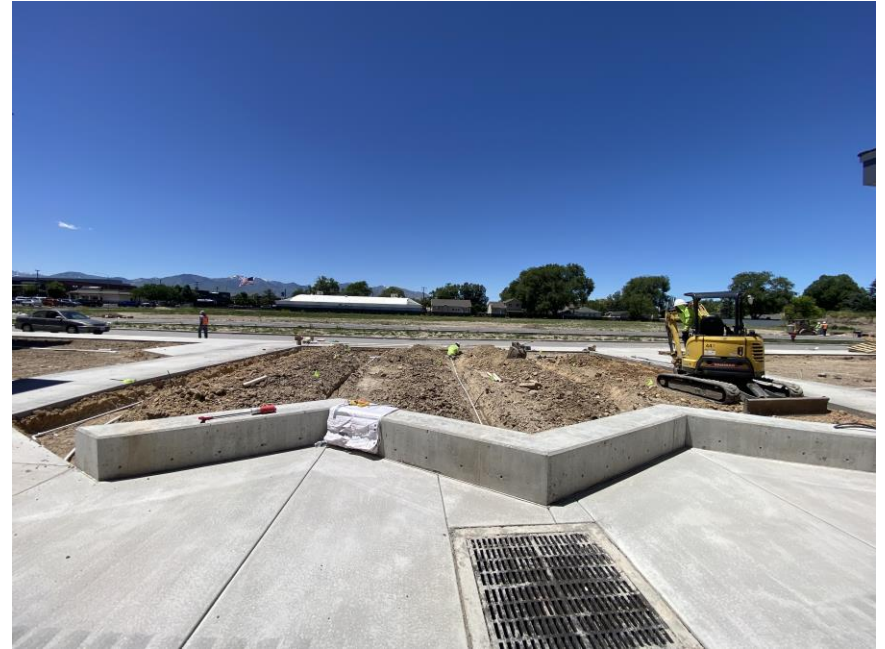
Landscaping and irrigation in progress
