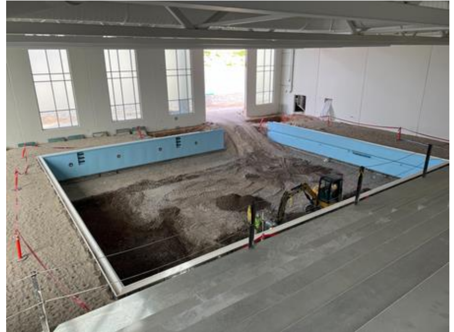
In-ground plumbing progress in the Pool
