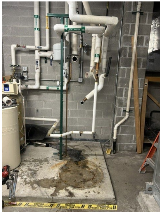
Empty platform after old hot water tank was removed.
